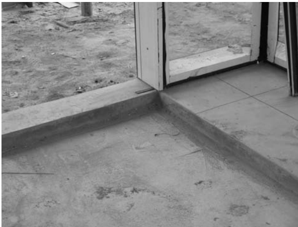
FIGURE 35.13 Blockout for a recessed floor mat. (Photo by author, courtesy of Hathaway Dinwiddie Construction Company and The California Institute of Technology.)
