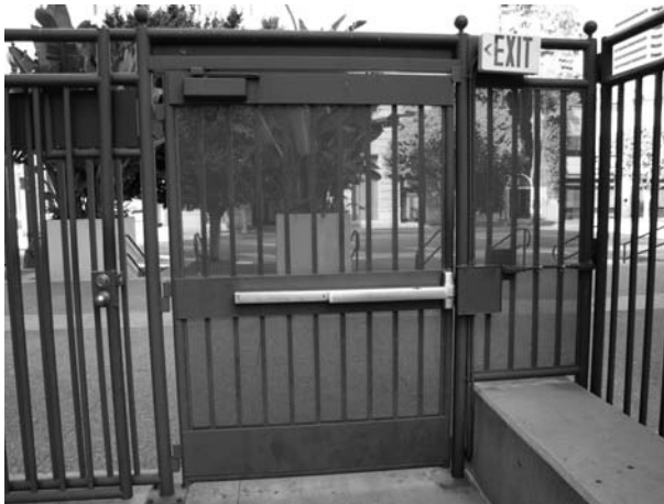
FIGURE 12.6 Door hardware at metal gate.
