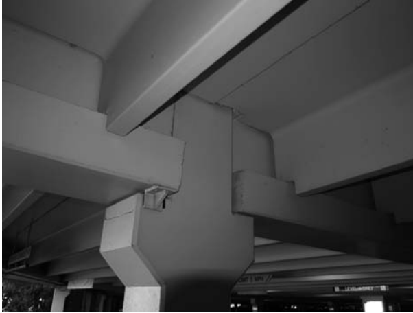
FIGURE 17.4 Structural precast connection.
