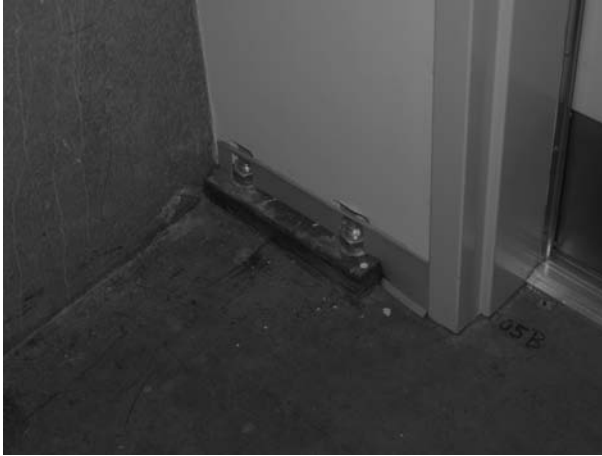
FIGURE 12.2 Baseplate sticking out of a wall.
