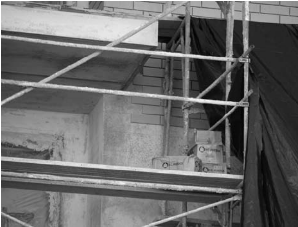
FIGURE 16.2 Thin brick on top of plaster base.
