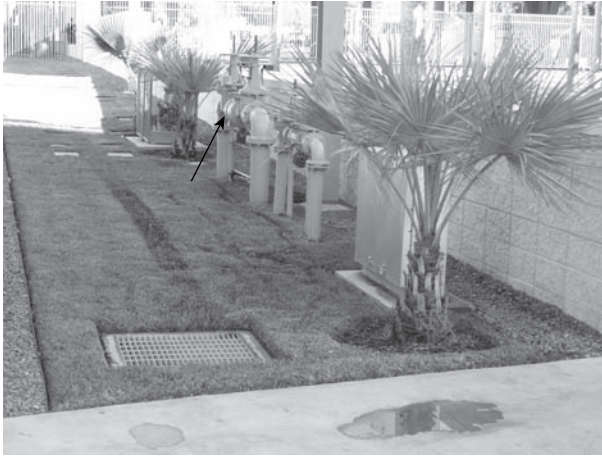
FIGURE 38.2 Backflow preventer.
