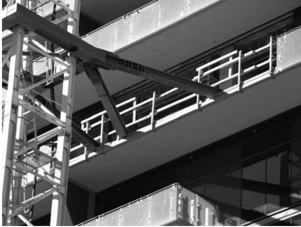
FIGURE 47.2 Tower crane lateral support at building deck.
