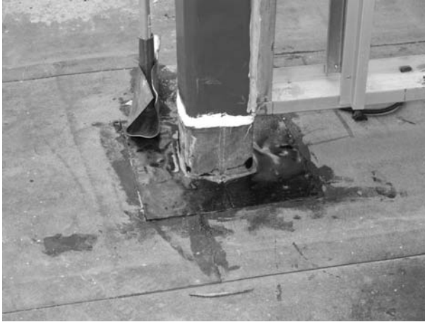
FIGURE 20.2 Lead roof jack. (Photo by author, courtesy of Hathaway Dinwiddie Construction Company and California State University Northridge.)
