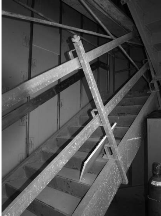
FIGURE 7.2 Slab grabber. (Photo by author, courtesy of Hathaway Dinwiddie Construction Company and The University of Southern California.)
