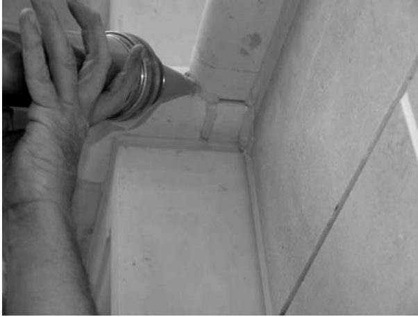
FIGURE 23.1 Sealant application. (Photo by author, courtesy of Hathaway Dinwiddie Construction Company and The University of Southern California.)
