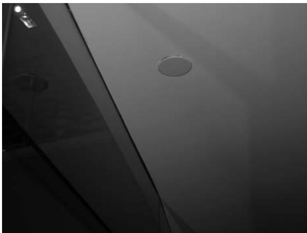
FIGURE 39.4 Sprinkler baffle.
