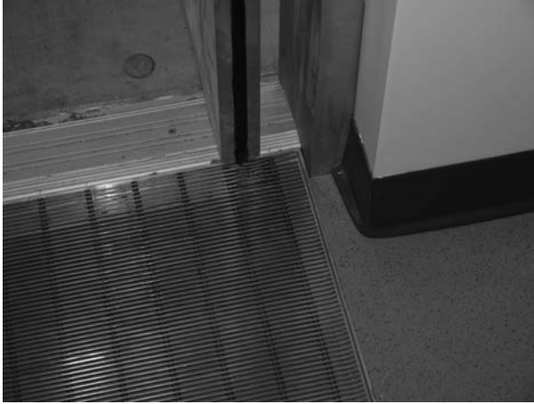
FIGURE 35.12 Recessed floor mat. (Photo by author, courtesy of Hathaway Dinwiddie Construction Company and The California Institute of Technology.)
