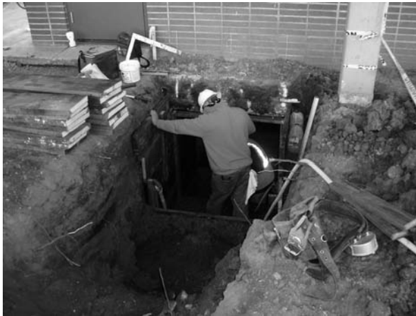
FIGURE 2.11 Underpinning. (Illustration provided by Malcolm Drilling.)
