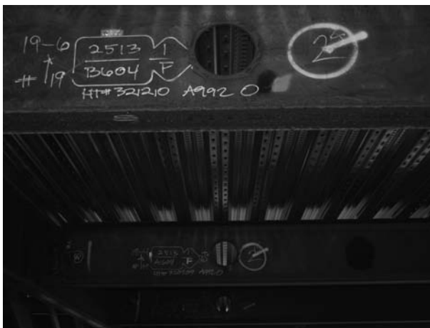
FIGURE 10.3 Beam penetration. (Photo by author, courtesy of Hathaway Dinwiddie Construction Company and Tishman Speyer.)
