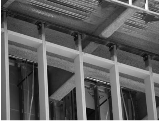
FIGURE 22.4 Curtain wall head support.
