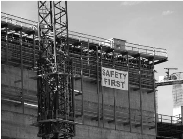
FIGURE 7.1 Integration of safety railings with the formwork.
