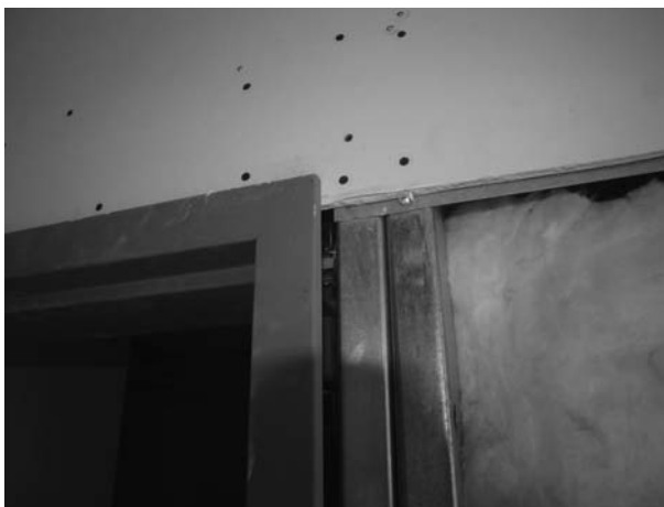
FIGURE 29.1 Door frame. (Photo by author, courtesy of Hathaway Dinwiddie Construction Company and California State University Northridge.)
