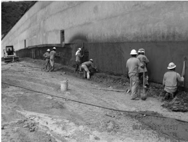
FIGURE 2.2 Shortcrete lagging. (Illustration provided by Malcolm Drilling.)
