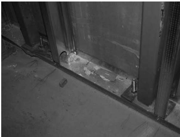
FIGURE 24.3 Low wall posts. (Photo by author, courtesy of Hathaway Dinwiddie Construction Company and The California Institute of Technology.)
