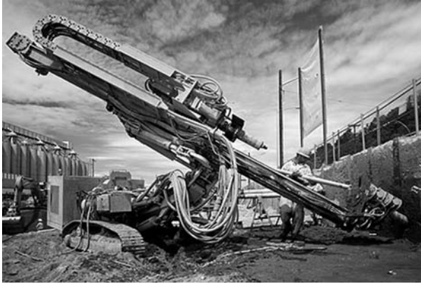
FIGURE 2.4 Tieback drilling rig. (Illustration provided by Malcolm Drilling.)
