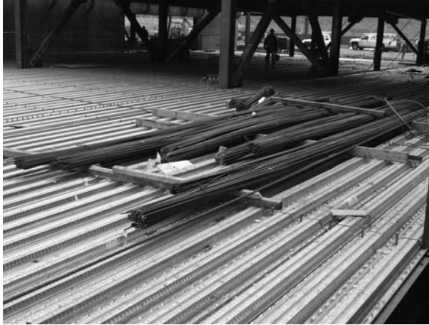
FIGURE 6.1 Reinforcing steel. (Photo by author, courtesy of Hathaway Dinwiddie Construction Company and Tishman Speyer.)
