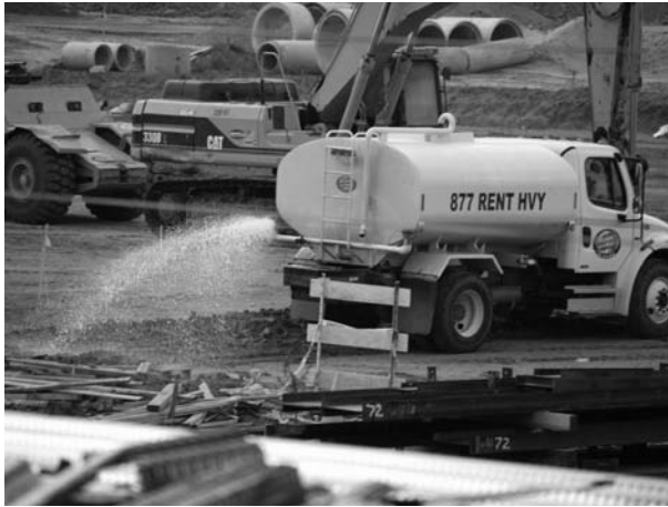
FIGURE 48.3 Water truck for dust control. (Photo by author, courtesy of Hathaway Dinwiddie Construction Company and Tishman Speyer.)
