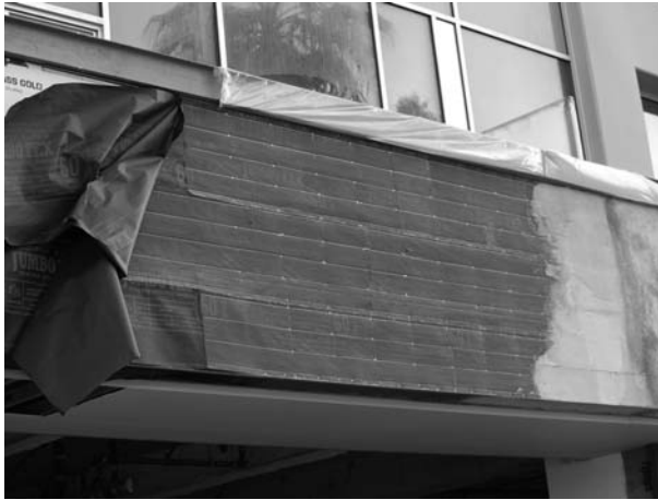
FIGURE 16.1 Plaster installation.
