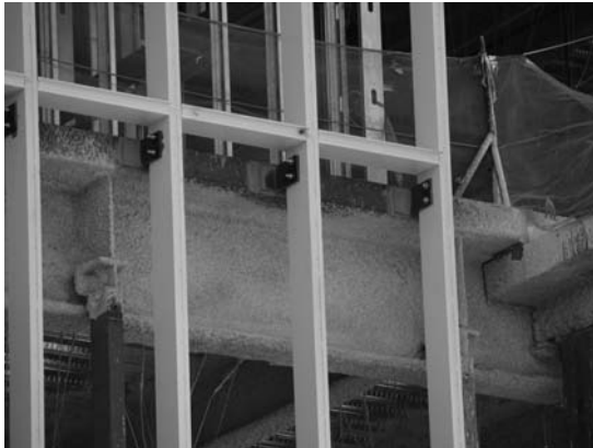
FIGURE 22.5 Curtain wall intermediate support.
