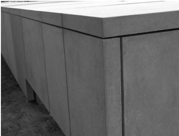
FIGURE 17.2 Architectural precast. (Photo by author, courtesy of Hathaway Dinwiddie Construction Company and The California Institute of Technology.)
