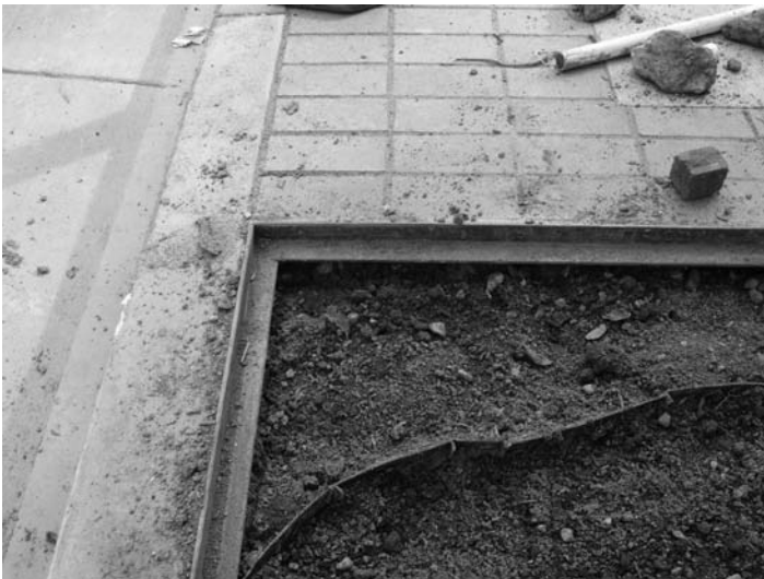
FIGURE 44.1 Tree grate. (Photo by author, courtesy of Hathaway Dinwiddie Construction Company and The University of Southern California.)
