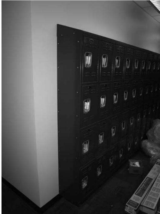
FIGURE 35.6 Locker with base and sloped top. (Photo by author, courtesy of Hathaway Dinwiddie Construction Company and The University of Southern California.)
