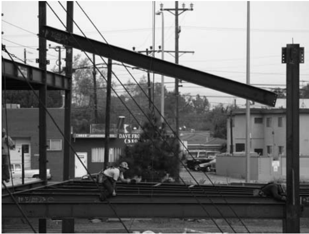
FIGURE 10.1 Steel erection. (Photo by author courtesy of Hathaway Dinwiddie Construction Company and Tishman Speyer.)
