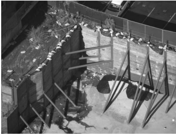
FIGURE 2.12 Rakers and corner bracing.
