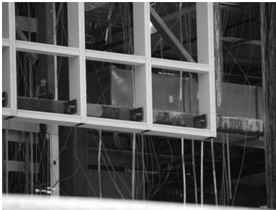
FIGURE 22.6 Curtain wall base support.
