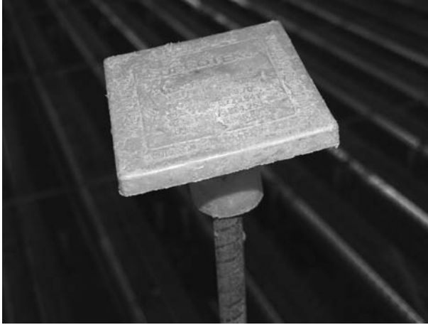
FIGURE 6.3 Rebar protective cap. (Photo by author, courtesy of Hathaway Dinwiddie Construction Company and Tishman Speyer.)
