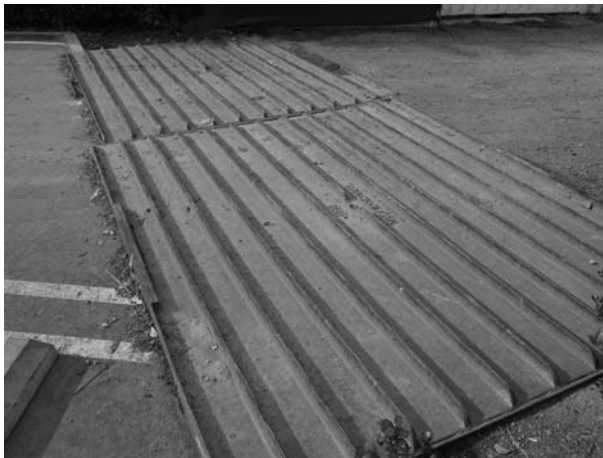
FIGURE 48.1 Roll off (rock) plates to knock mud off of truck tires. (Photo by author, courtesy of Hathaway Dinwiddie Construction Company and California State University Northridge.)
