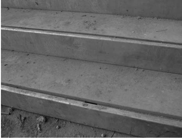
FIGURE 12.1 2x blocking in stair pan for construction use. (Photo by author, courtesy of Hathaway Dinwiddie Construction Company and California State University Northridge.)
