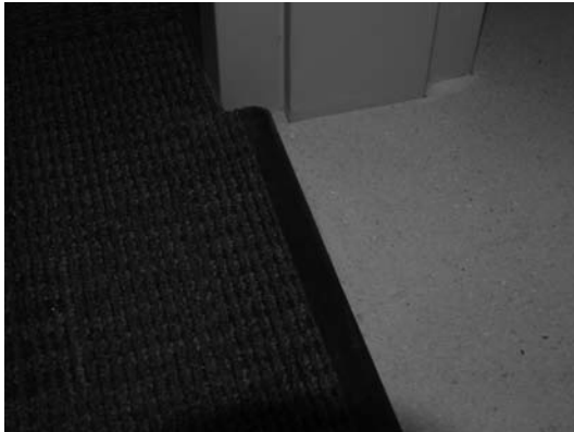
FIGURE 31.3 Transition strip. (Photo by author, courtesy of Hathaway Dinwiddie Construction Company and The University of Southern California.)
