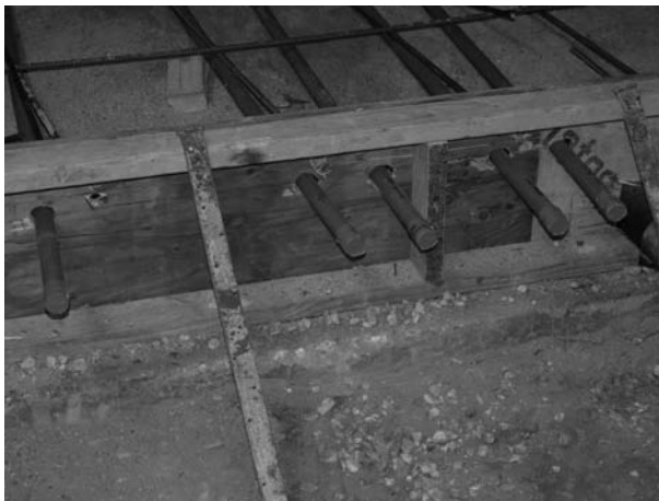
FIGURE 7.6 Conduits penetrating formwork. (Photo by author, courtesy of Hathaway Dinwiddie Construction Company and Tishman Speyer.)
