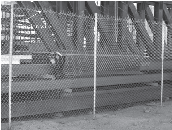
FIGURE 45.3 Chain link fence with tension wire.
