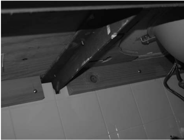
FIGURE 24.4 Counter support angles. (Photo by author, courtesy of Hathaway Dinwiddie Construction Company and The California Institute of Technology.)
