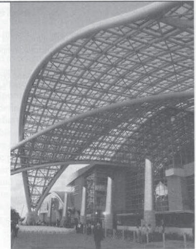
Puerto Rico Convention Center. Photo courtesy Walter P Moore.
