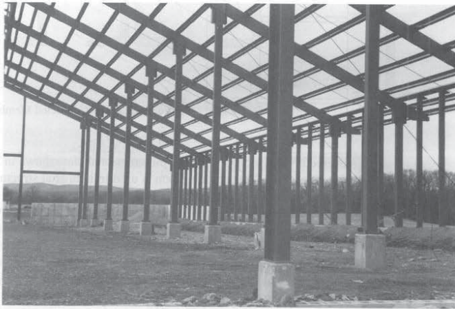
Figure 4.4 Sag Rods in a Roof System.
