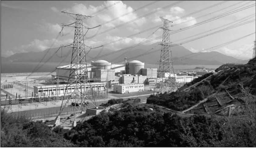
5.1: Ling Ao, China: first two of four 1000 MW PWR supplied by Areva and completed 2004. Two more units are under construction. (Photo Courtesy of Areva NP)
