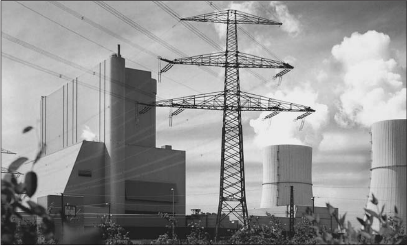
4.2; Schwarze Pumpe, Germany, 1600 MW supercritical steam plant, also sends steam loads to a briquette factory and the local district heating network. (Photo courtesy of Siemens)
