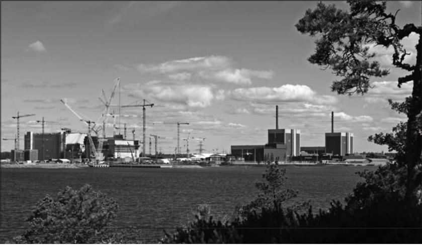
5.5: Okiluoto, Finland: View of the site in August 2008 with the first EPR reactor, Unit 3, under construction at left. Application has been made for a fourth unit at the site. (Photo courtesy of TVO)
