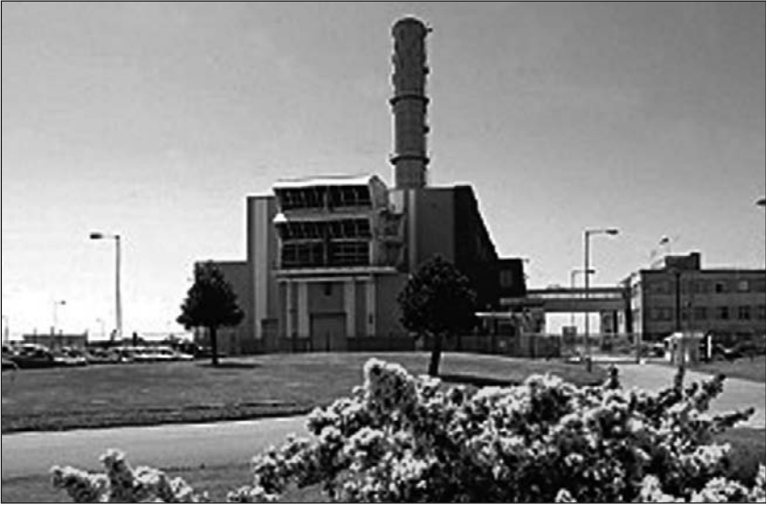
6.2: Roosecote, UK: 220 MW combined cycle plant was built in the turbine hall of a former 120 MW power station near Barrow in Furness. (Photo courtesy of Centrica)
