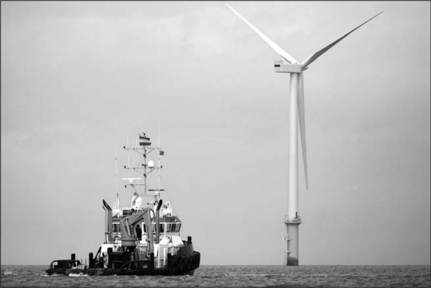
8.3: One of twenty-five units of Siemens' largest wind generator, rated 3.6 MW forming the Burbo Bank wind farm in Liverpool Bay. (Photo courtesy of Siemens)
