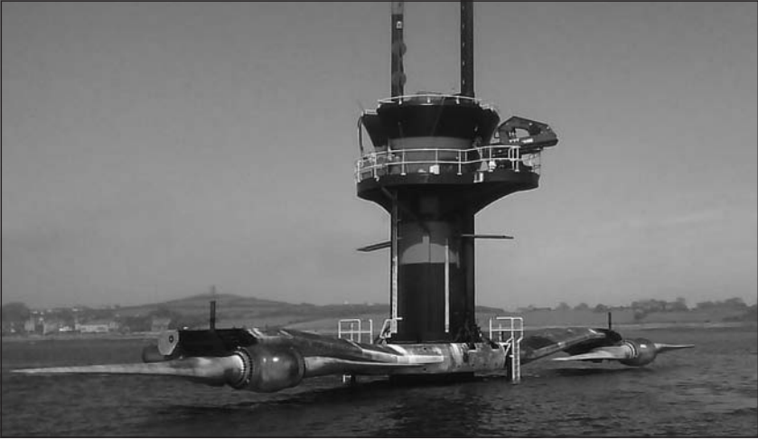
8.8: UK: Seagen commercial prototype with the generators raised out of the water as they would be for maintenance. (Photo courtesy of Marine Current Turbines )
