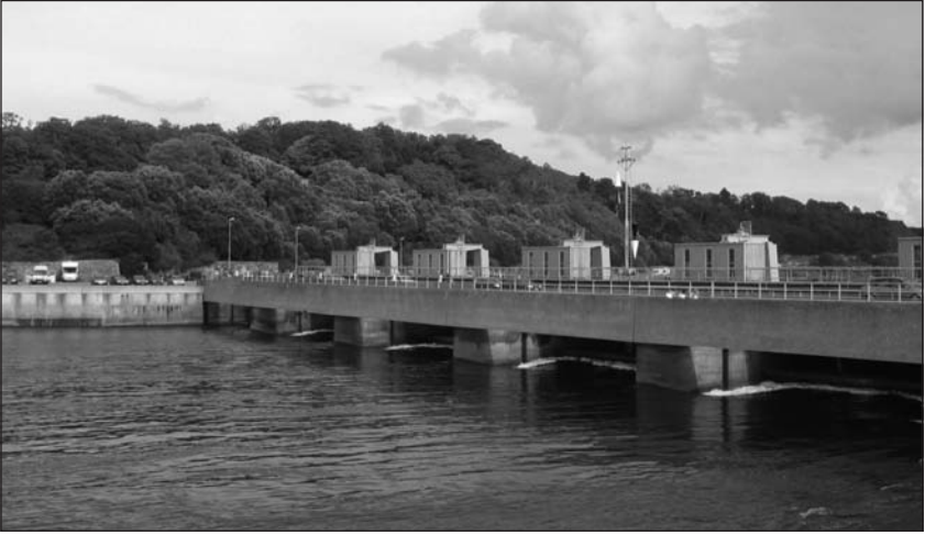
8,7 La Rance, France: 240 MW tidal power station generates on the rising and falling tides and is the largest of its type in the world. (Photo courtesy of Electricité de France)
