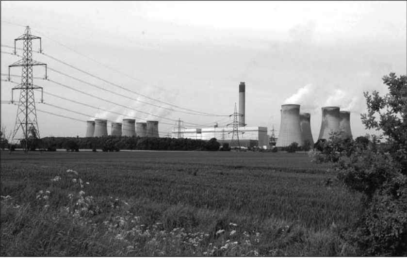
4.7: Drax, UK. This 4000 MW coal-fired power station, will from 2009 be co-firing 10% solid biomass along with turbine upgrades to reduce greenhouse gas emissions.
