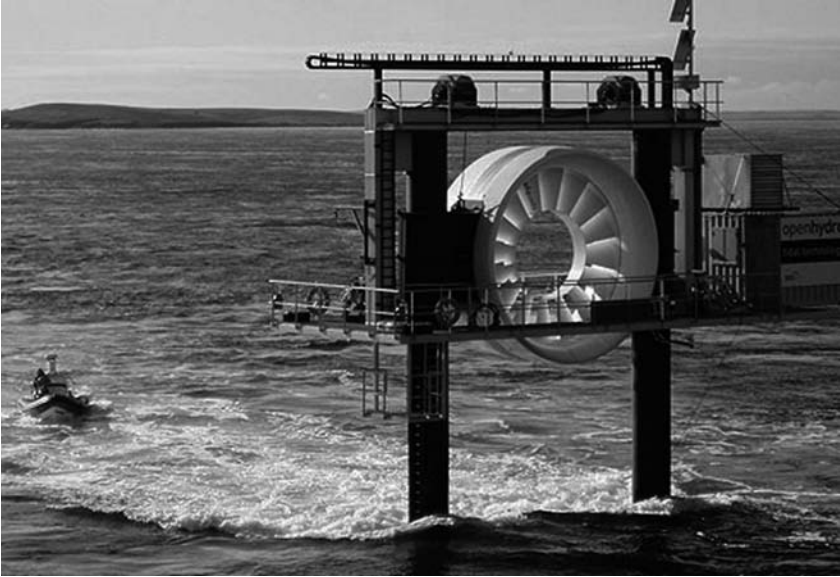
7.5: Open Hydro 250 MW prototype on the test rig at the European Marine Energy Centre in Orkney. (Photo Courtesy of Open Hydro)
