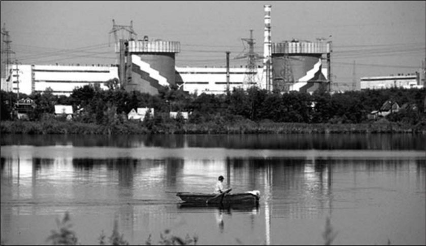
5.8: Kalinin, Russia: the first station with the 1000 MW PWR went into service in 1984. There are three operating reactors on the site and a fourth under construction. (Photo courtesy of Rosenergoatom)
