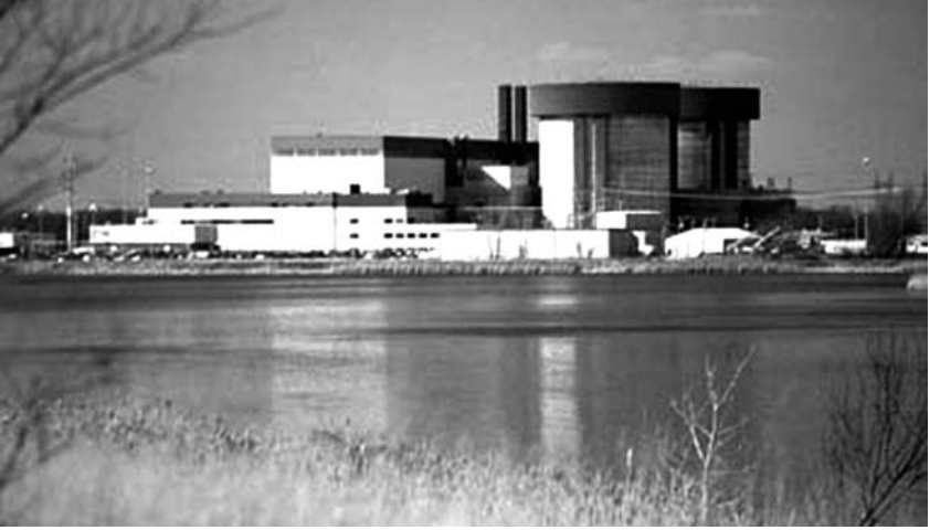
5.9: Braidwood, IL, USA. Located 100 km southwest of Chicago, these two 1200 MW Westinghouse PWR's went into service in 1988. (Photo courtesy of Exlelon Corporation)
