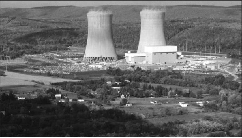
5.10: Susquehanna, PA, USA: PPL's twin BWR station has had turbines uprated and license extension. Plan to install a US-EPR nearby at Bell Bend. (Photo courtesy PPL)
