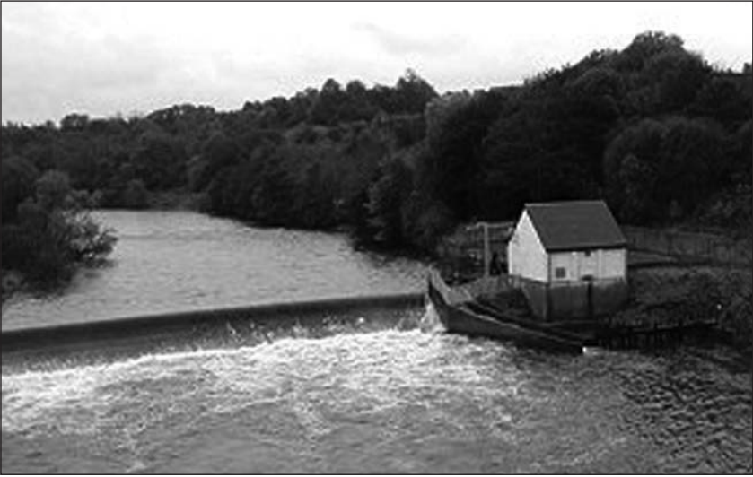
8.5: Blantyre, Scotland: RWE Npower's 575 kW hydro station 15 km above Glasgow on the Clyde was built at an existing weir. (Photo courtesy of Npower Renewables)
