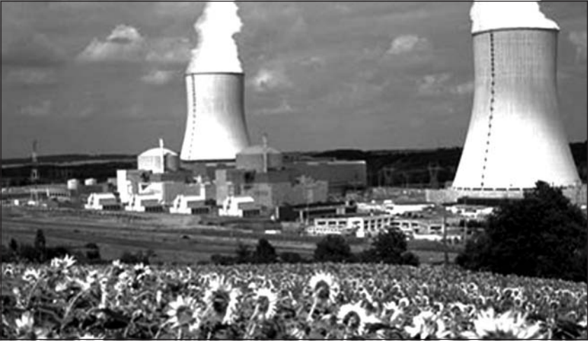
5.4: Civaux, France. EdF's station was the first with the 1400 MW Type N4 reactor from which has been developed the EPR. (Photo courtesy of Areva NP)
