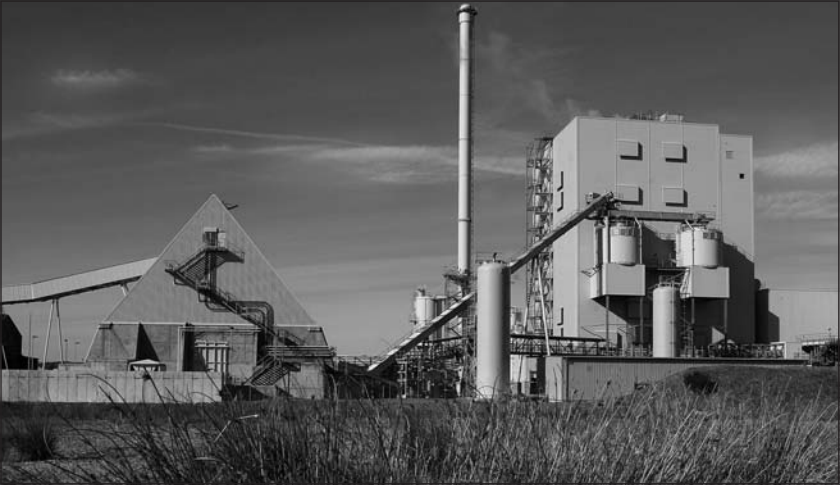
8.2: Lockerbie, UK: This 44 MW biomass-fired power plant burns wood waste from local saw mills and forestry operations. (Photo courtesy of E.ON (UK))
