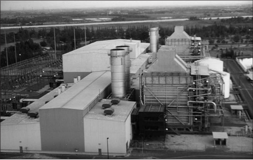
6.3: Thailand. Bang Pakong: the second combined cycle there completed 1992, was the first of four plants built by EGAT using a common 310 MW block design.
