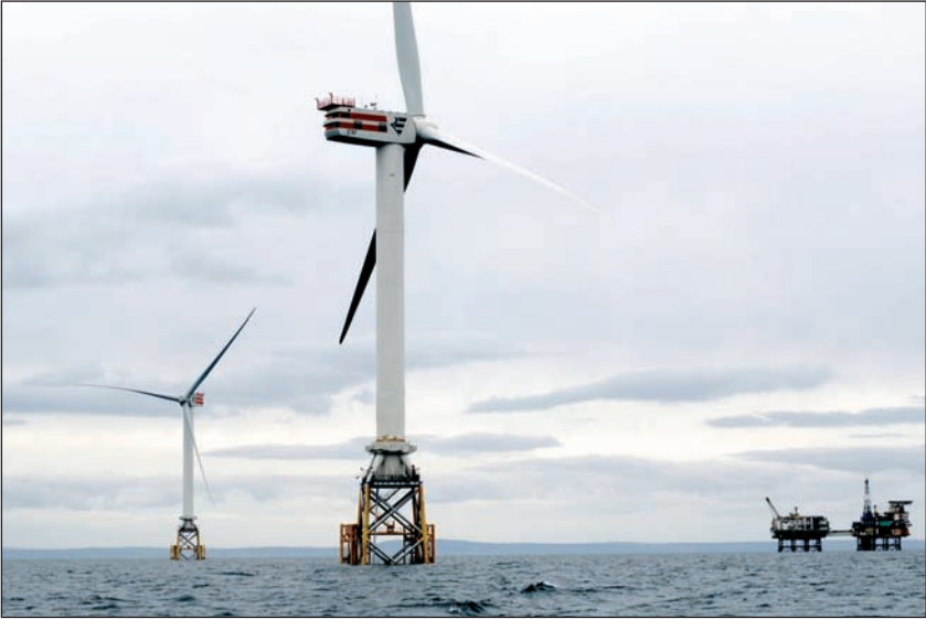
8.4: Two 5MW wind generators off the Scottish coast supply all their output to the Talisman oil platform shown at right. (Photo courtesy of RE Power Systems)
