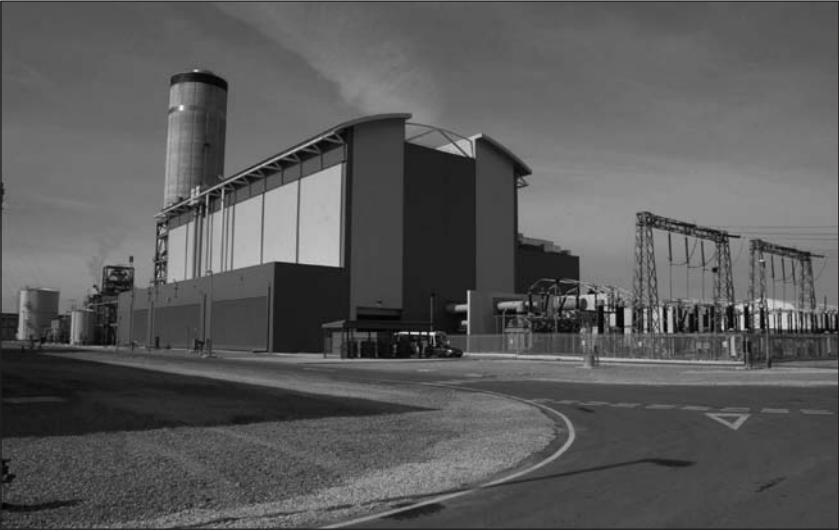
6.8: Baglan Bay, South Wales. This 480 MW combined cycle was the first with the GE Frame 9H gas turbine, which went into commercial operation in September 2002.
