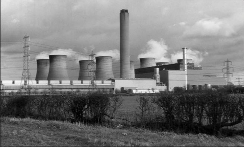
6.5: Cottam, UK: 400 MW combined cycle with prototype Benson heat recovery boiler. In the background EdF Energy's 2000 MW coal-fired power plant.
