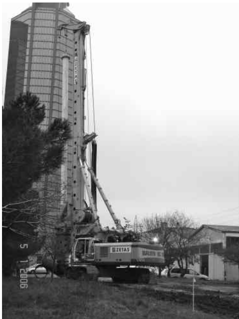
FIGURE 13.1 Rotary drill rig, Bauer BG 36 used in Istanbul in one construction site. (Adapted from the archive of Bilgin, N., 2006. A large-diameter drill rig study in Cifteler construction site in Istanbul. Istanbul Technical University, p. 30.)
