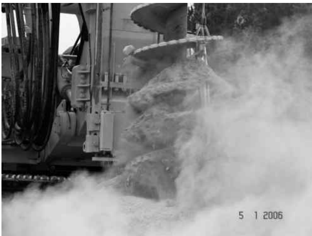
FIGURE 13.2 Cutting debris and dust generation when pulling out the drilling drum. (Adapted from the archive of Bilgin, N., 2006. A large-diameter drill rig study in Cifteler construction site in Istanbul. Istanbul Technical University, p. 30.)
