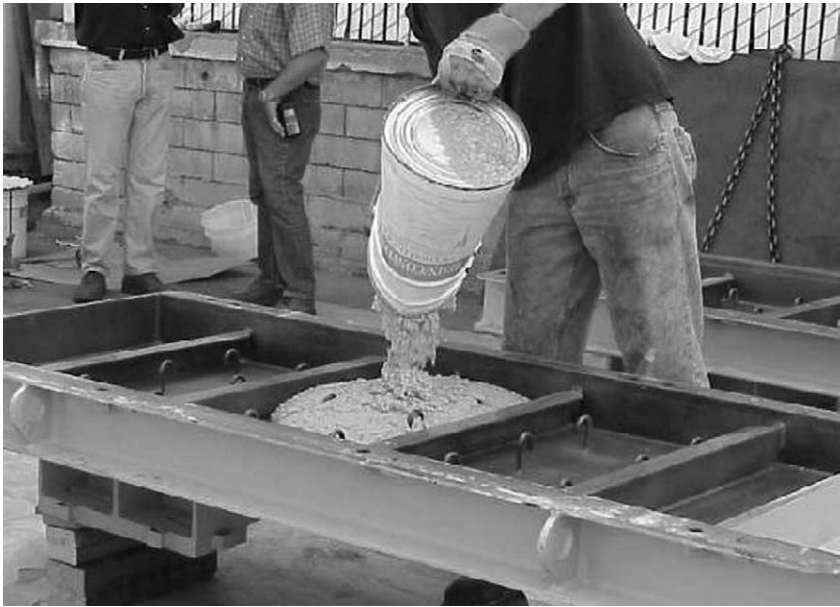
Figure 14-13. Pre-grouting a pump base.
