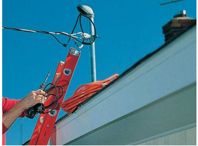
Use fiberglass or wood ladders when making routine household repairs near the service mast.
