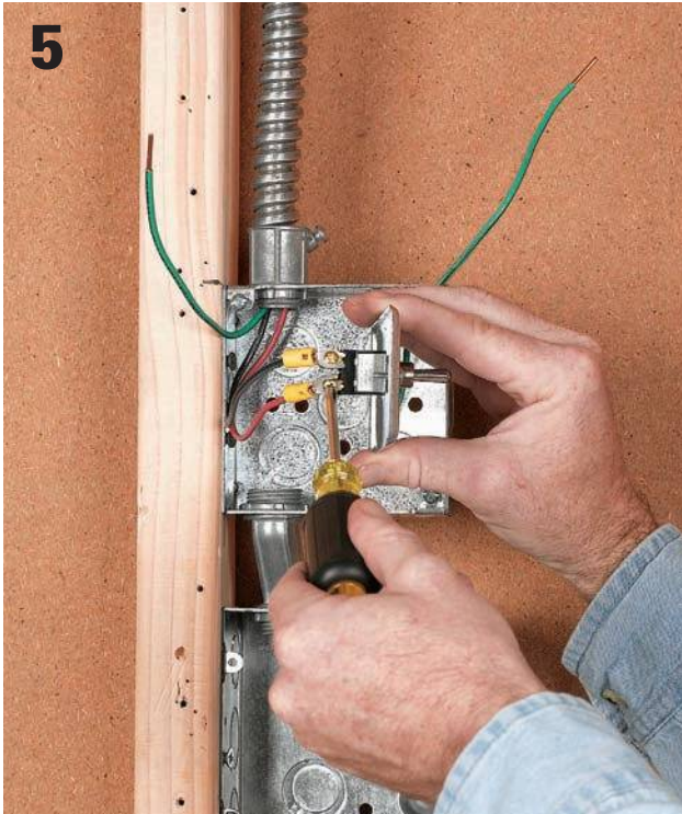
5 Attach the DC disconnect switch to the wire leads from the power source.
