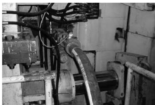
Figure 22. Grout port at axis of TBM.
