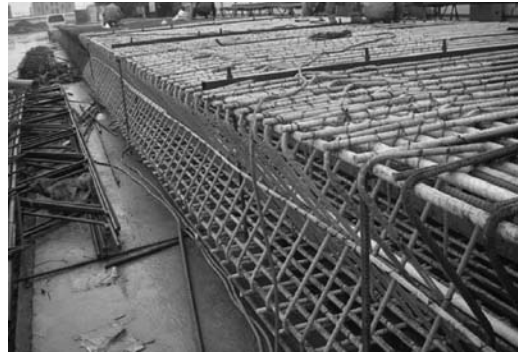
Figure 17. GFRP bars binding site.
