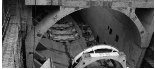
Figure 7. Concrete reaction structure.
