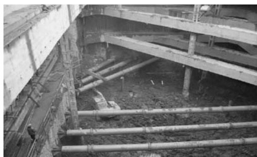
Figure 3. Fuxing (E) Tunnel – Foundation pit excavation.
