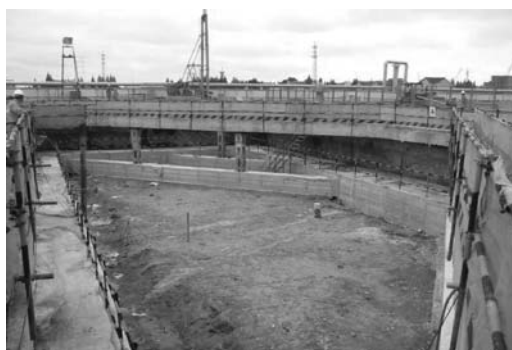
Figure 5. Changjiang Tunnel – Enclosure structure construction.
