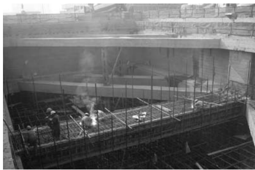
Figure 4. Xiangyin Road Tunnel – inner structure construction.
