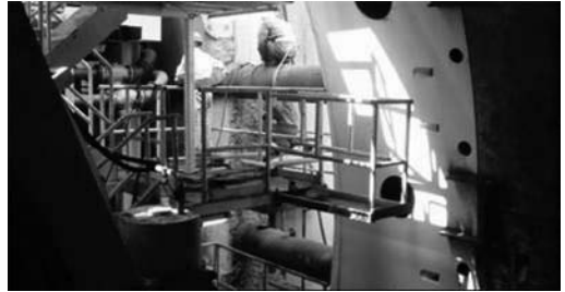
Figure 8. Installing the pipe struts between the concrete reaction structure and the steel thrust frame.
