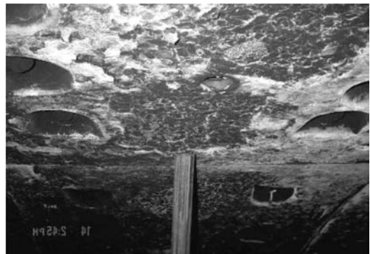
Figure 2. Fire damage to tunnel lining in Shanghai Metro tunnel fire.
