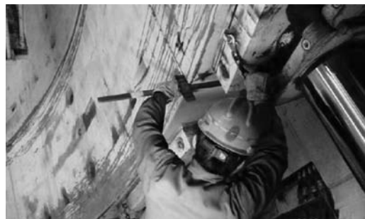
Figure 24. Measuring ‘tailskin gaps’.
