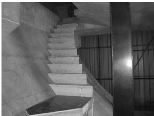
Figure 12. Wooden prototype of escape stairs.
