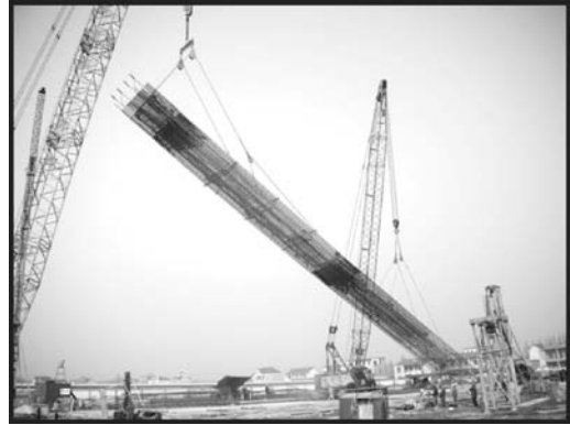
Figure 3. Lifting of GFRP reinforcement cage.
