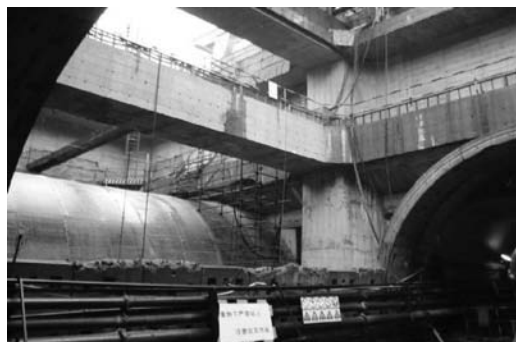
Figure 2. Dalian Road Tunnel – Shield launching.
