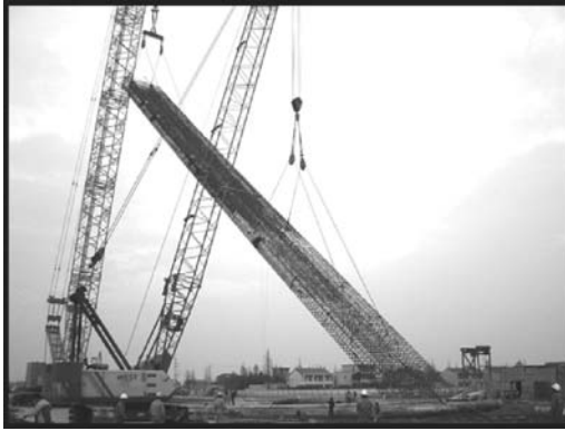
Figure 5. Lifting of reinforcement cage.
