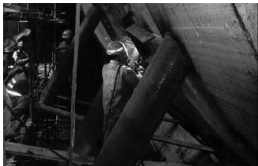
Figure 10. Propping 'shove' rings in shaft.
