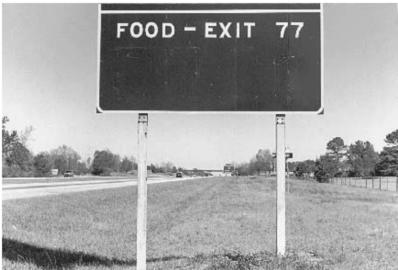
FIGURE 7.31 Multiple-mount sign support.
