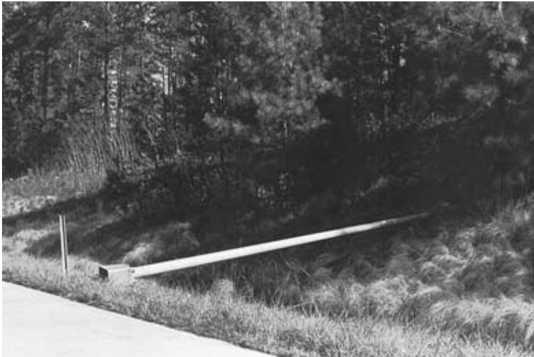
FIGURE 7.95 Failure of luminaire support without impact.
