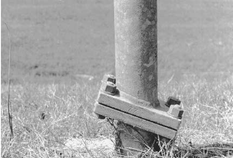
FIGURE 7.27 Installation of unidirectional slip base.
