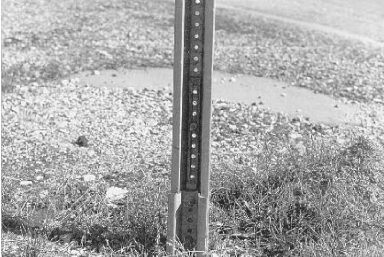
FIGURE 7.7 Example of breakaway single sign support.
