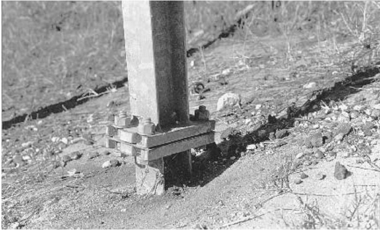
FIGURE 7.8 Example of mechanical release support type.
