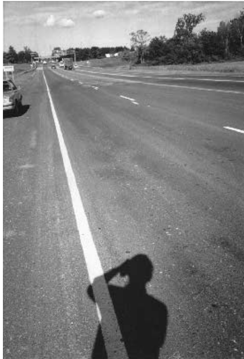
FIGURE 3.32 Example of bleeding in flexible pavement.
