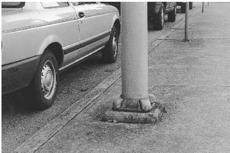
FIGURE 7.89 Flange-type steel base.
