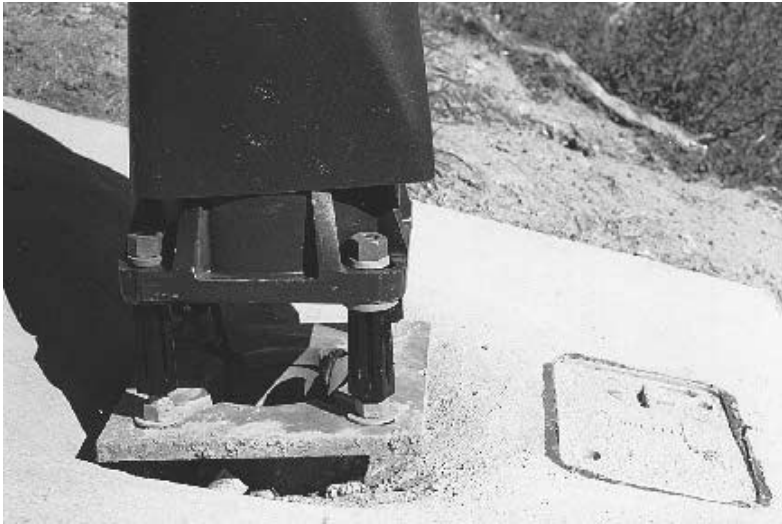
FIGURE 7.90 Frangible-coupling luminaire support.
