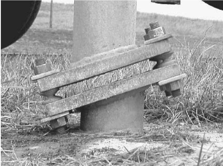
FIGURE 7.30 Frangible-coupling sign support.
