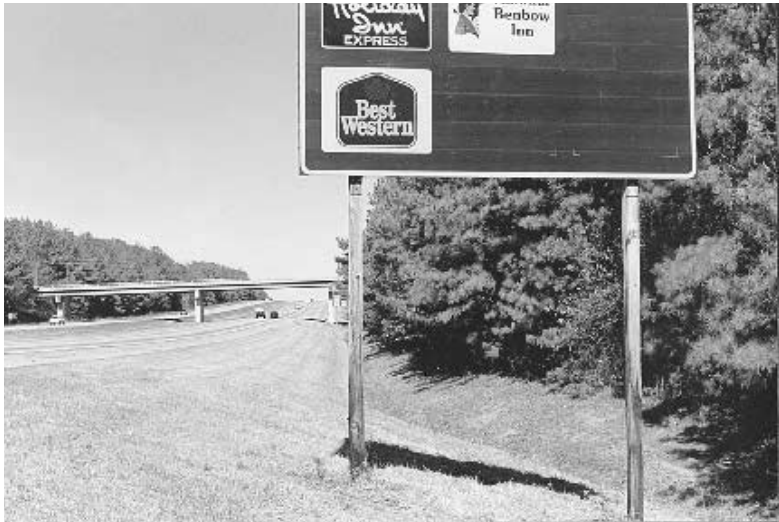
FIGURE 7.61 Multiple-mount frangible wood post design.
