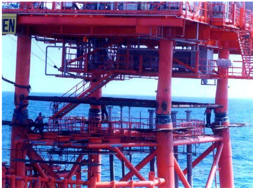
FIGURE 5.46 Installation of the deck on the pile.
