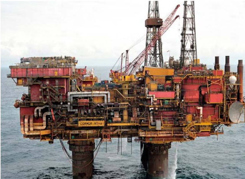
FIGURE 1.6 Concrete gravity platform.
