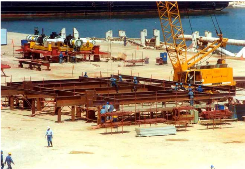
FIGURE 5.26 Fabrication of the topside.
