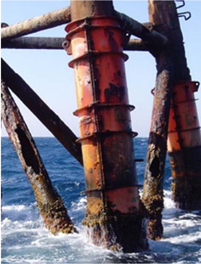
FIGURE 7.47 Corroded bracing.
