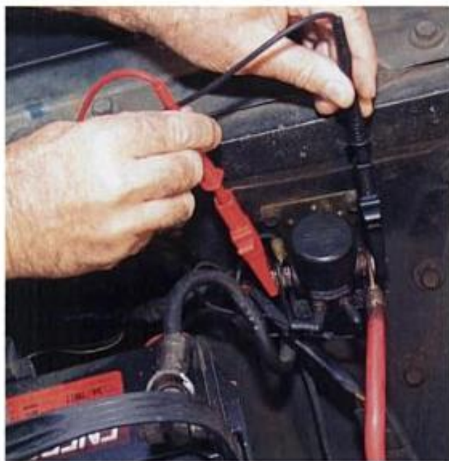
This remote starter solenoid can easily be checked for high resistance using a voltage drop test. The contacts inside the solenoid should not exceed a drop of 0.2 volt during starter cranking.
