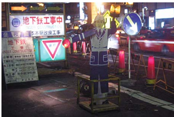
Figure 6.5. A policeman-shaped figure in a street in Tokyo, Japan, is being used to alert traffic at a construction site. Photo by Adi Marom.
