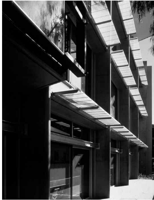
Figure 27.6 Horizontal sunshades on the northern façade.
