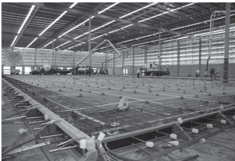
Figure 3.3 Examples of post-tensioned slabs before concrete casting. (Courtesy of VSL Australia Limited, Sydney, New South Wales, Australia.)
