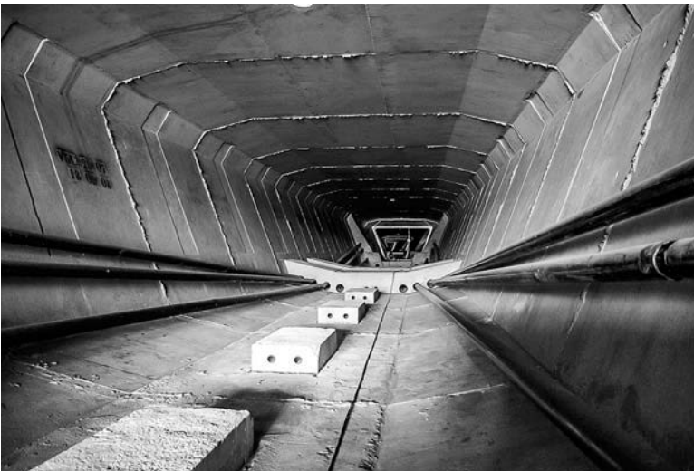
Figure 3.14 External tendons in bridge box girder section. (Courtesy of VSL International Limited, Hong Kong, China.)
