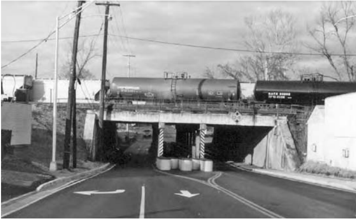
FIGURE 5.3 View of the viaduct with a train running on top (East Street Viaduct, West Virginia).
