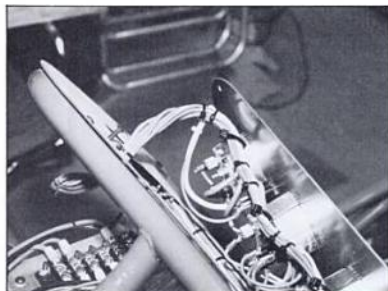
Instrument panel tips out for easy service. We provided loop in gauge feed wires to accommodate this feature. As you can see, wiring was done before car's outer skin was installed, making it a snap.
