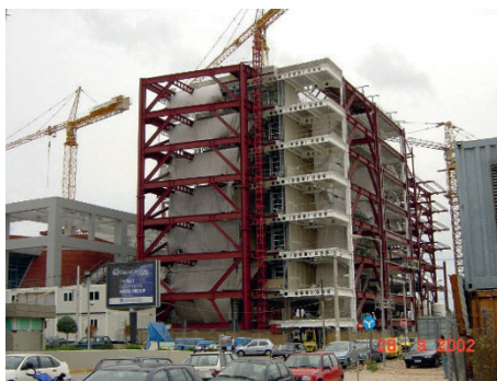
Fig. 7.31. Steel building with eccentric bracings
