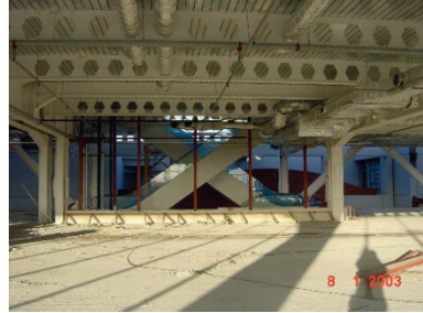
Fig. 7.9. Castellated beams in steel buildings
