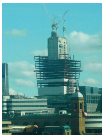
Fig. 7.33. Steel building with a concrete core, under erection
