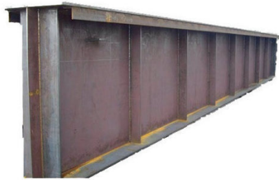
Fig. 4.20. Plate girder with transverse stiffeners
