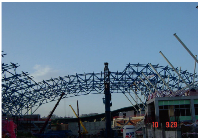
Fig. 8.23. Erection of the central part of a large opening structure follows erection of the end parts
