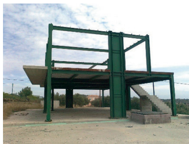
Fig. 7.35. Example of a steel building with steel shear panels
