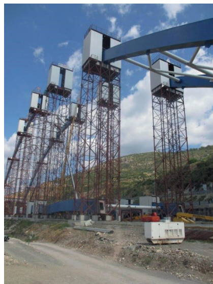
Fig. 8.3. Protection cabins for on-site welding between arch segments of a bridge
