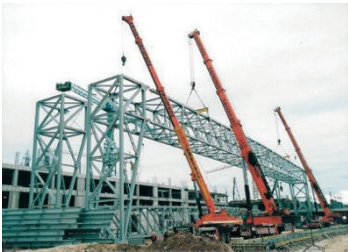
Fig. 8.21. Erection of a pair of plane latticed frames
