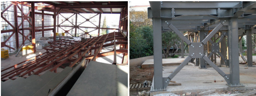
Fig. 7.29. Examples of buildings with concentric bracing systems
