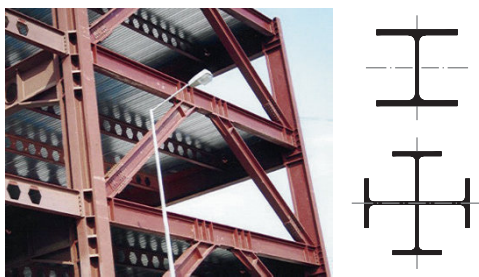
Fig. 7.2. Steel buildings column with crossed double I-section
