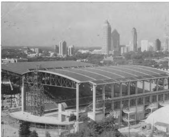
FIGURE 8.8 Roof of Atlanta's Aquatic Center with 345-kW grid-connected PV power system. (From Georgia Institute of Technology. With permission.)
