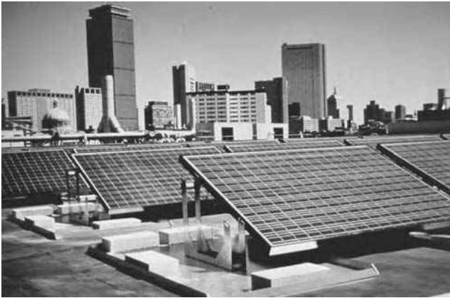
FIGURE 13.2 18 kW grid-connected PV system on the Northeastern University Student Center in Boston. (Source: ASE Americas, Billerica, MA. With permission.)
