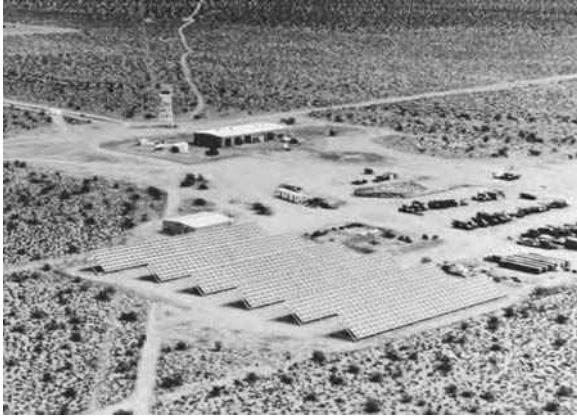
FIGURE 12.6 A 300-kW PV–diesel hybrid system in Superior Valley, California. (From ASE Americas, Inc., Billerica, MA. With permission.)
