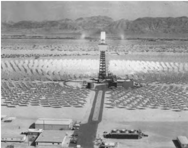
FIGURE 17.3 Solar-II plant site view. (From: U.S. Department of Energy.)
