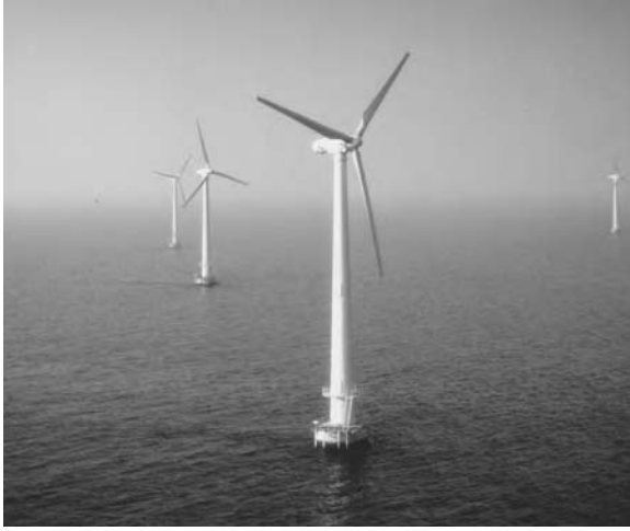
FIGURE 7.1 Vindeby offshore wind farm in Denmark. (From Vestas Wind Systems, Denmark. With permission.)
