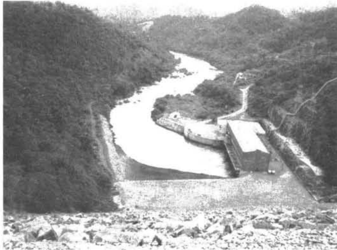
Fig. 3.14 An overall view of Power Station.
