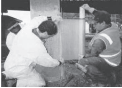
Wrapping with Glass Fiber
