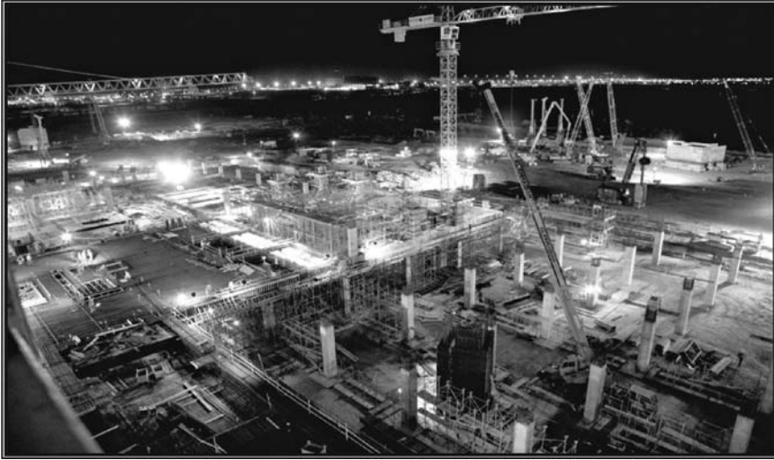
FIGURE 9.5 Masdar Institute under construction.
