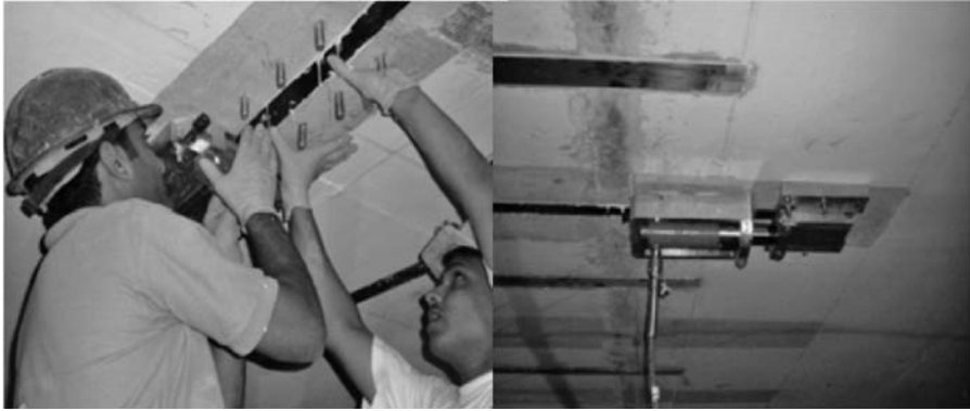
FIGURE 10.8 Fixing of laminate with adhesive in the machine. The pump for giving pressure is attached.
