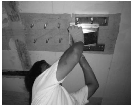
FIGURE 10.7 Positioning of laminate clamping device between L-clamps.
