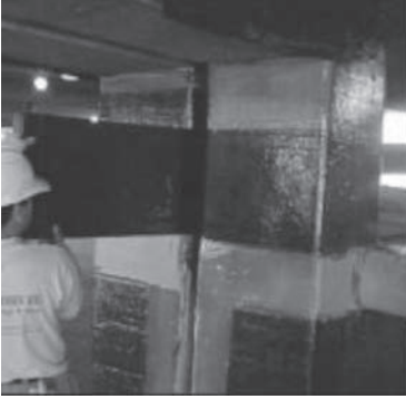
Wrapping with Carbon Fiber
