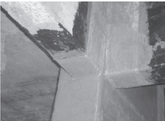
RC Columns after Completion of FRP Wrapping
