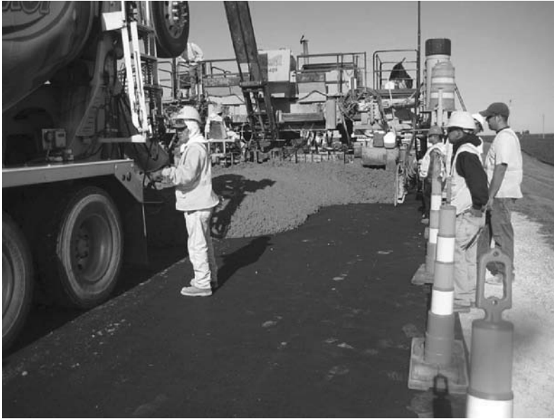
FIGURE 5.3 Concrete overlays can restore or enhance an existing pavement's functional and structural performance. (From Van Dam, T. and Taylor, P. C. Building Sustainable Pavements with Concrete—Briefing Document, Ames, IA, CP Road Map, 2009. http://www.cproadmap.org/publications/sustainability_briefing.pdf [accessed May 2011]. With permission.)
