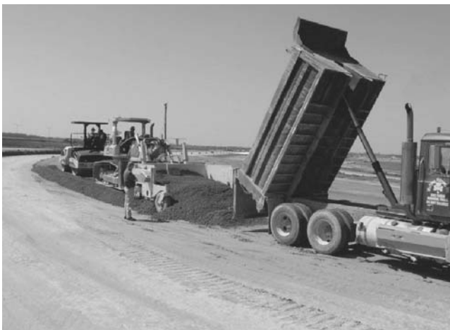
FIGURE 6.14 DFW airport perimeter taxiway being paved with RCC. (From Johnson, J. 2008. RCC pavement at Denver International Airport, PCA.)
