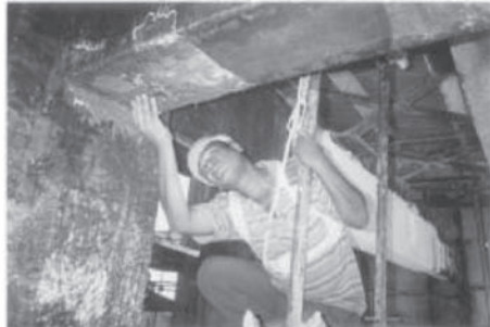
Repair of Hairline Cracks
