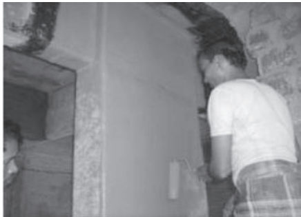
Application of Saturant on FRP Wrapping
