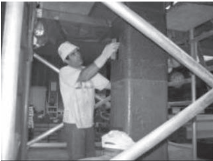
Application of Saturant on FRP Wrapping
