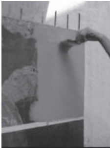
Application of Saturant
