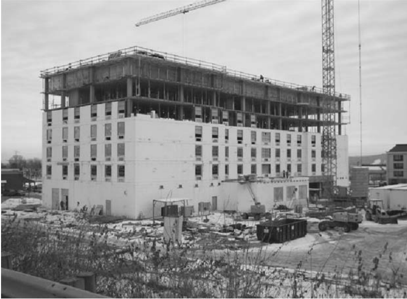
FIGURE 4.13 Drury Inn, Indianapolis, Indiana, under construction with ICF walls. (Courtesy of Amvic Building Systems.)
