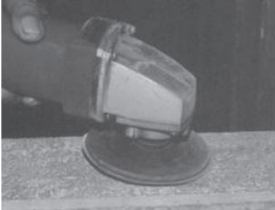
Grinding the Concrete Surface
