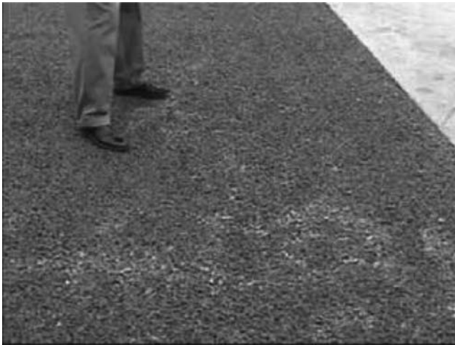
FIGURE 7.1 Demonstration of water draining in pervious concrete. (Courtesy of Green Builder.)
