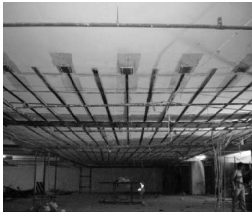
FIGURE 10.9 The final look of the slab after fixing all the prestressed laminate.
