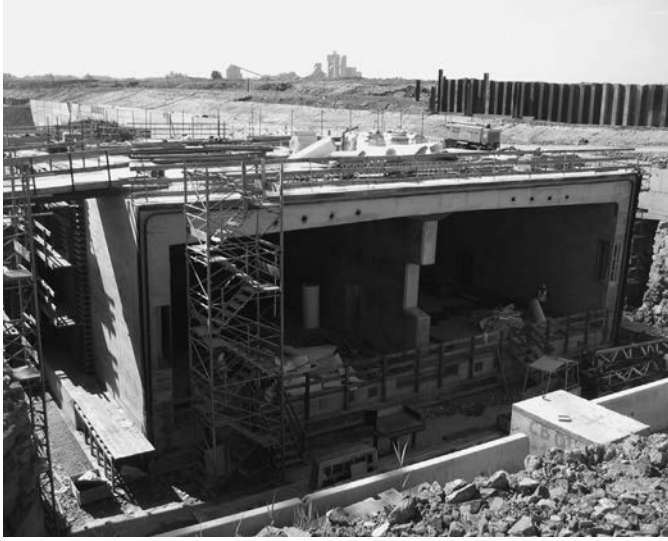
Figure 5.71 Construction of one of the elements for the Limerick immersed tube tunnel in Ireland. (Courtesy of COWI A/S.)
