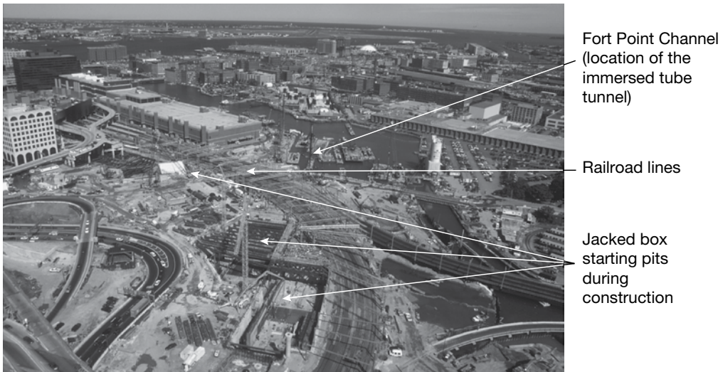
Figure 5.84 An overview of the jacked box sites in Boston showing the railroad lines and Fort Point Channel. (Courtesy of Massachusetts Turnpike Authority.)
