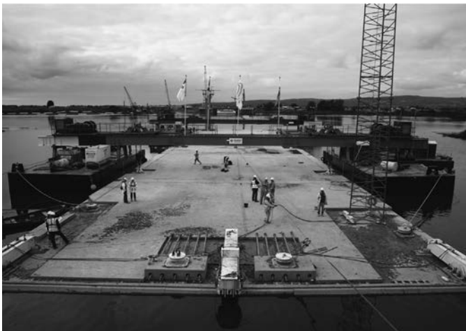
Figure 5.72 One of the elements for the Limerick immersed tube tunnel being towed into position ready for sinking. (Courtesy of COWI A/S.)
