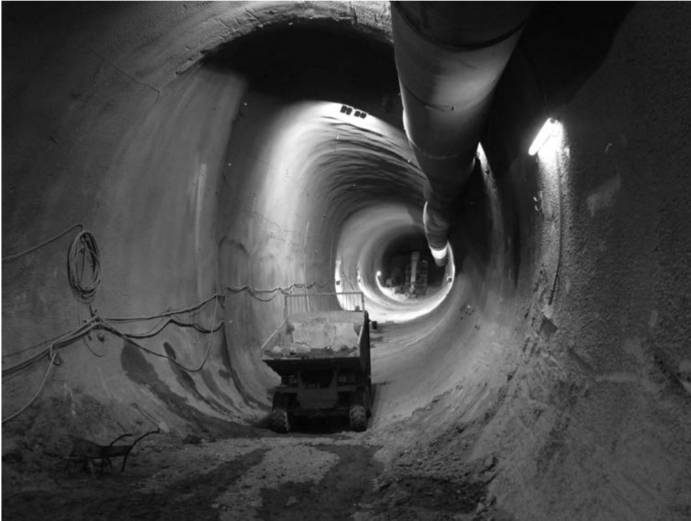
Figure 8.37 Whitechapel Station, Eastbound Cavern. This photograph shows the cavern (where the lorry is) after completion of stage 4 (see Figure 8.36 ). The circular Eastbound Running tunnel is visible in the foreground and background (line of sight is west). (Photo Credit: Crossrail Ltd., used with permission.)
