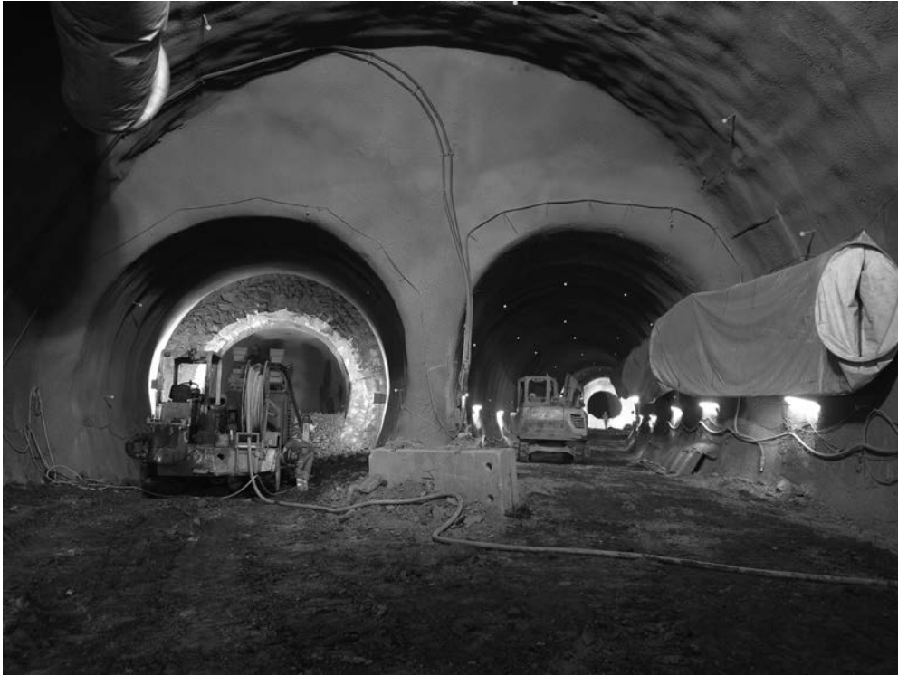
Figure 8.35 Whitechapel Station, Westbound Cavern. On the left is the TBM Launching Chamber, with the advance of the enlargement ready to be sprayed. The Crossover tunnel on the right is nearly completed. (Photo Credit: Crossrail Ltd., used with permission.)
