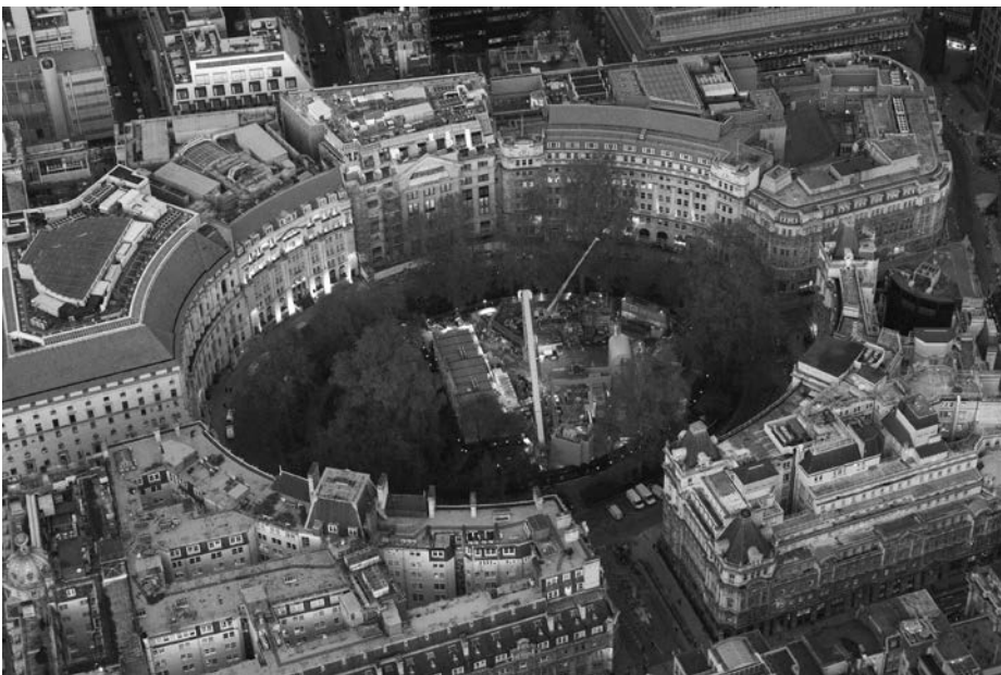
Figure 8.39 Construction site for Liverpool Street Station at Finsbury Circus. (Photo Credit: Crossrail Ltd., used with permission.)
