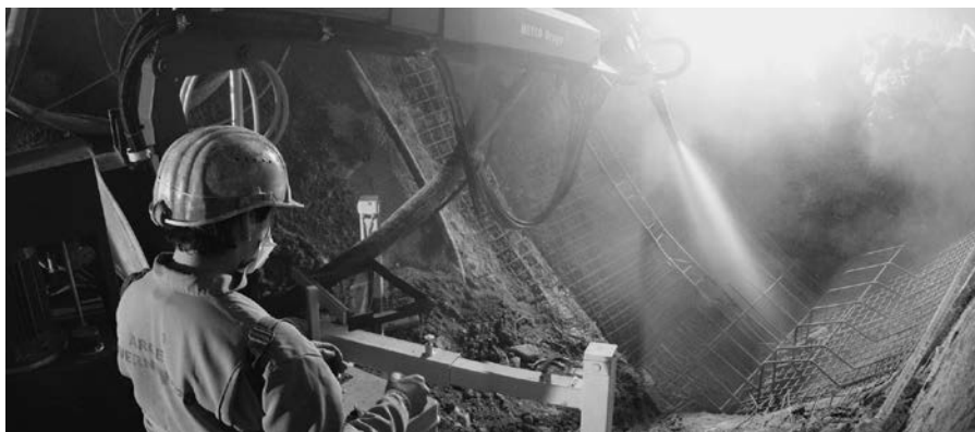
Figure 4.18 Sprayed concrete application of the invert of a side wall drift during the construction of the Lainzer Tunnel LT31 in Vienna, Austria.
