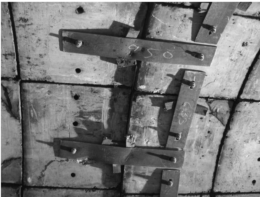
Figure 8.16 Existing Piccadilly Line Westbound Tunnel showing steps of up to 60 mm between concrete segments.
