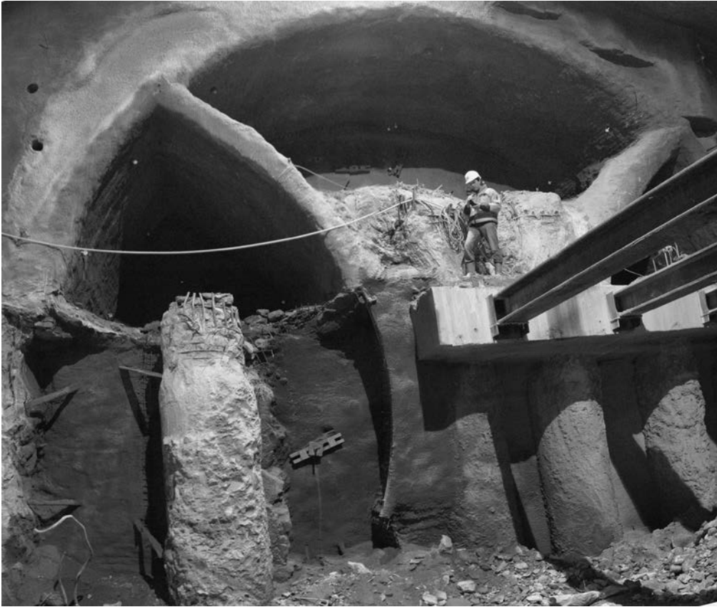
Figure 8.19 Crown excavated, and enlargement of the leading sidewall drift started. Remaining bracing still in place.
