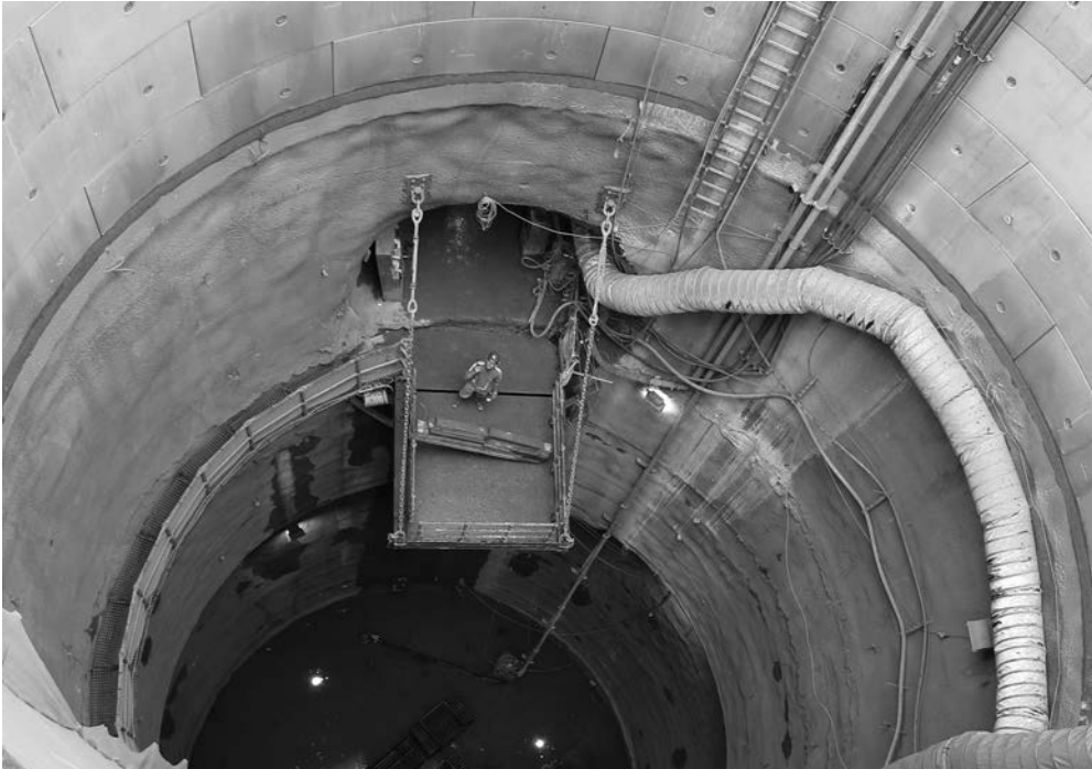
Figure 8.48 Drawbridge for one of the Geotechnical Adits at Liverpool Street Station. (Photo Credit: Crossrail Ltd., used with permission.)
