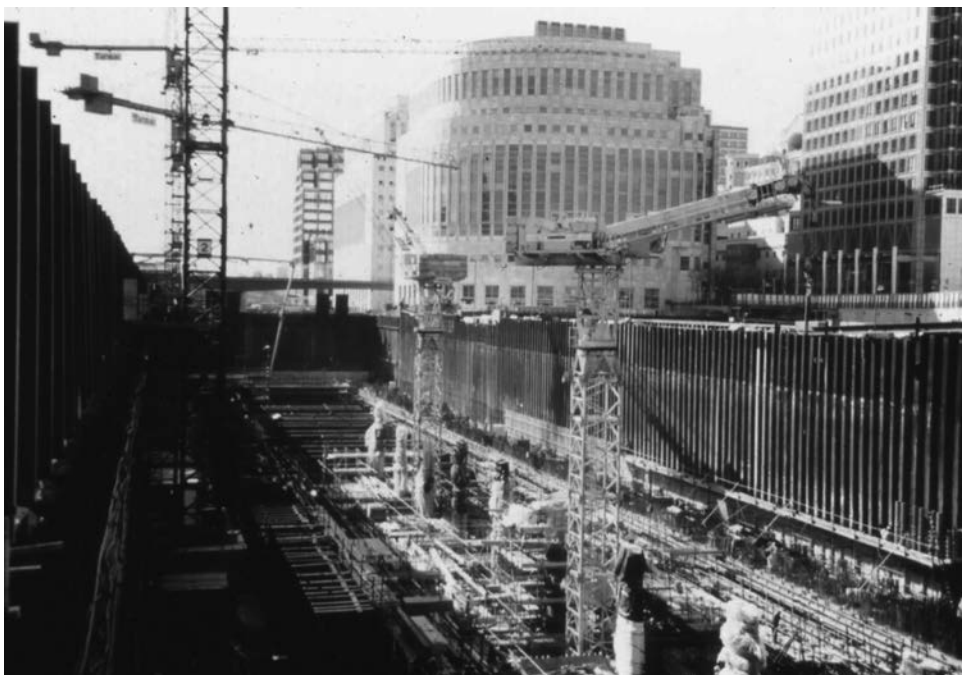
Figure 5.58 Canary Wharf Station during construction on the London Underground Jubilee Line Extension, UK.
