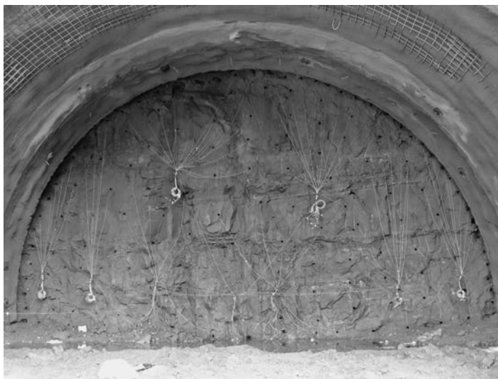
Figure 5.47 Example of a face ready to blast in the Heidkopf Tunnel, Germany.
