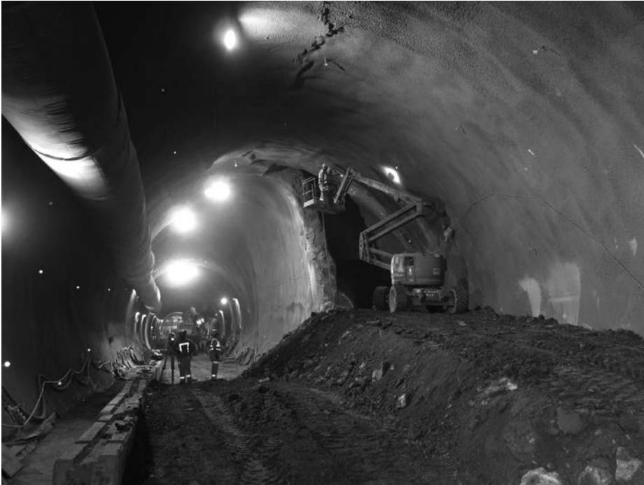
Figure 8.38 Whitechapel Station, Eastbound Cavern. The oval part shown in Figure 8.37 is visible on the left. The Eastbound Cavern was enlarged to its full size using a single sidewall drift on the right (line of sight is east). The surveyors on the left are waiting for the miners in the mobile working platform to clean the monitoring targets. (Photo Credit: Crossrail Ltd., used with permission.)
