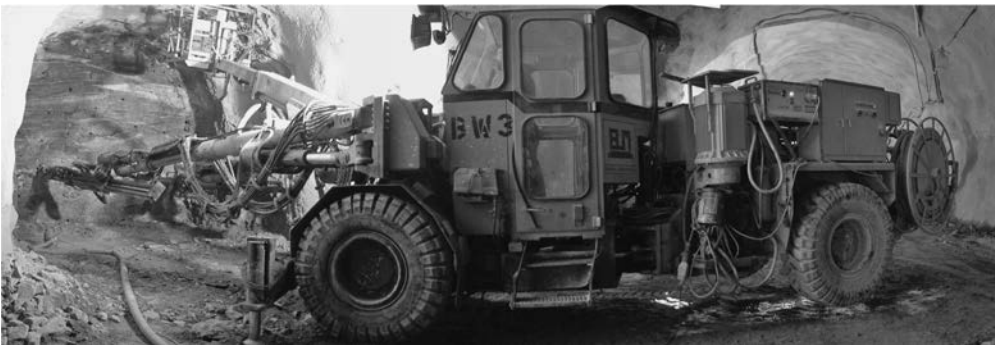
Figure 5.40 Example of a rubber tyred drilling carriage ‘jumbo’ as used on the second tube of the Katschberg Tunnel, Austria (details are provided in Section 4.3.3).
