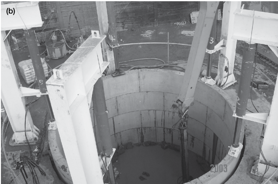
Figure 4.27 (a) Caisson-sinking method to construct shafts. (After BTS/ICE 2004, used with permission from ICE Publishing.) (b) Construction of a reception shaft for a pipe jacking operation as part of the Terminal 5 project at Heathrow, UK.
