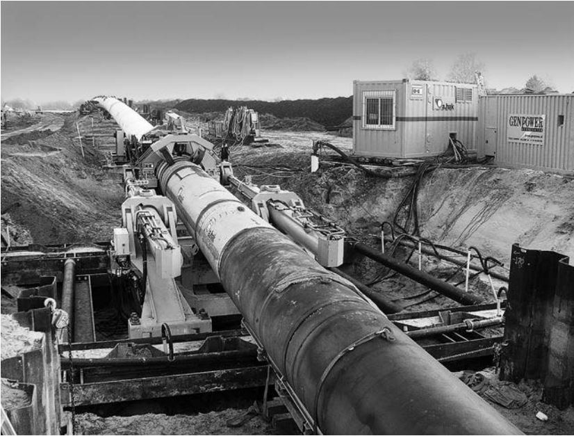
Figure 5.100 Example of Herrenknecht's pipe thruster as used in their Direct Pipe method for the North-South gas pipeline in the Netherlands. (Courtesy of Herrenknecht.)
