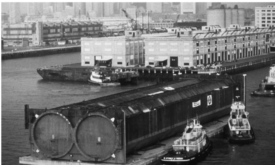
Figure 5.73 One of the tunnel elements for the Ted Williams Tunnel being towed prior to additional outfitting work. (Vanderwarker 2001.)
