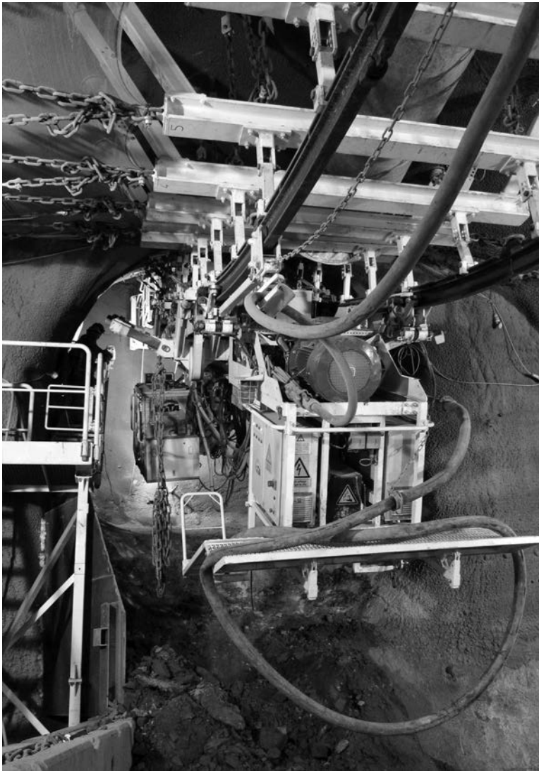
Figure 8.49 The Uphill Excavator hangs on rails which are braced back in the crown and shoulders of SCL (ES2, Liverpool Street Station). (Photo Credit: Crossrail Ltd., used with permission.)
