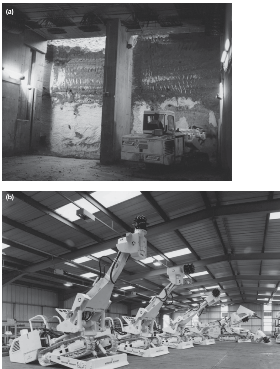
Figure 5.87 (a) Excavating the lower half of a 10 m high face through frozen, water-bearing sands and gravels and (b) Webster Schaeff excavating machines used on the Boston jacked box tunnels. (Clayton et al. 2001; Courtesy of BAM Nuttall Ltd. and John Ropkins Ltd.)
