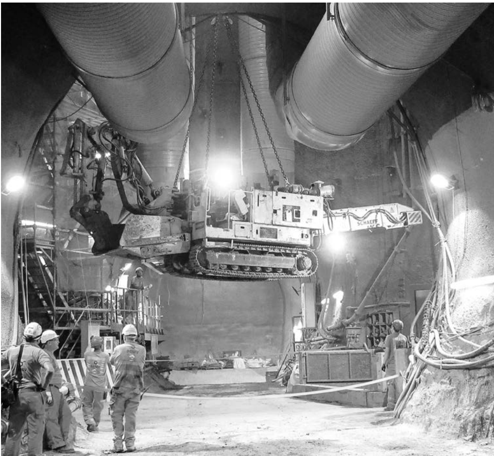
Figure 8.41 Construction Shaft, lifting a Schaeff ITC 312 excavator. During the lifting operation, only the two supervising banksmen (lifting operation supervisors) are allowed to stay within the shaft area. (Photo Credit: Crossrail Ltd., used with permission.)
