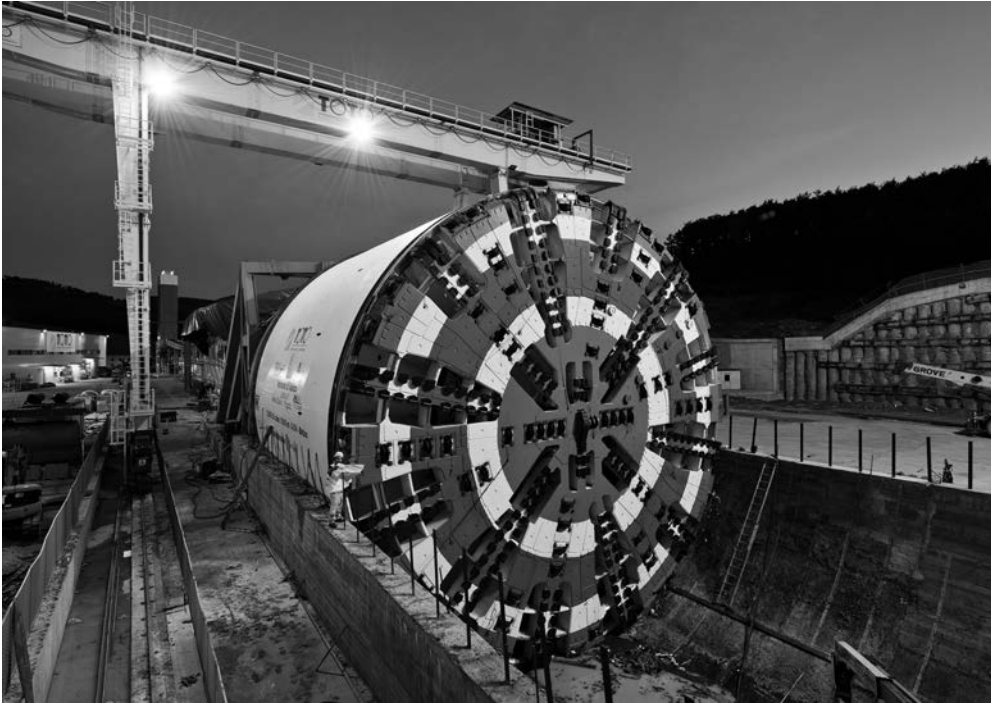
Figure 8.57 A 15.6 m diameter EPBM used on the Sparvo tunnel in Italy. (Courtesy of Herrenknecht.)
