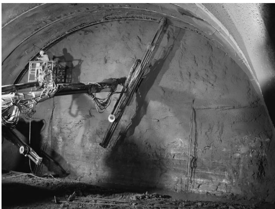
Figure 4.9 Anchor installation associated with sprayed concrete lining, HKT Tunnel, Germany. (Courtesy of BeMo Tunnelling GmbH Innsbruck.)
