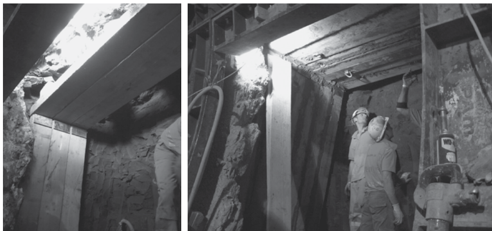
Figure 5.1 Timber heading as used in London Clay for constructing a connecting passage between the two running tunnels (connecting passages \sim 4\text{--}9\text{ m}^2 ), King's Cross Station upgrade, London (construction period 2002–2008). (Courtesy of BeMo Tunnelling GmbH Innsbruck.)
