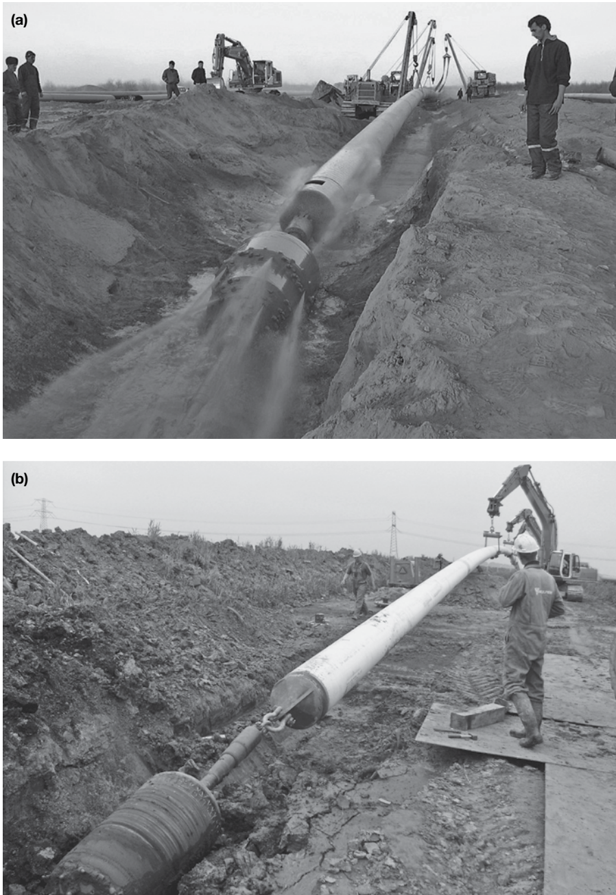
Figure 5.99 (a) Pullback operations showing back reamer and (b) final pipe. (Courtesy of Prime Drilling HDD-Technology.)
