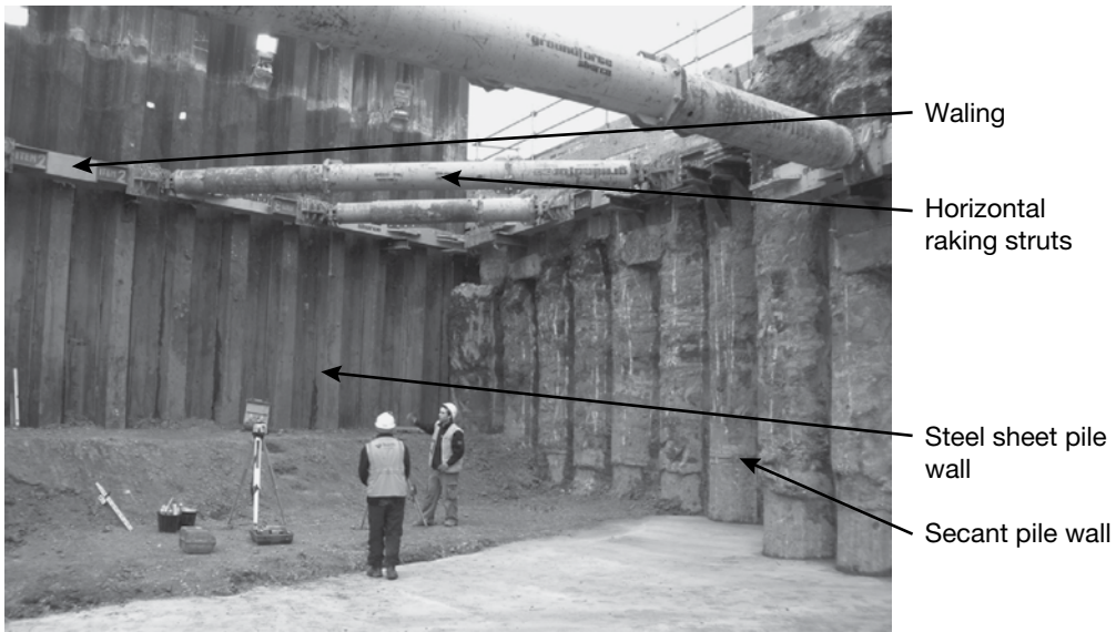
Figure 5.66 Secant pile wall as used as part of the jacking pit for a jacked box tunnel at Owen Street, Tipton, UK (see Section 5.10 on jacked box tunnels). The photograph also shows the steel sheet pile headwall with its waling and horizontally raking struts transferring the headwall loading into one of the secant piled sidewalls. (Courtesy of BAM Nuttall Ltd. and John Ropkins Ltd.)
