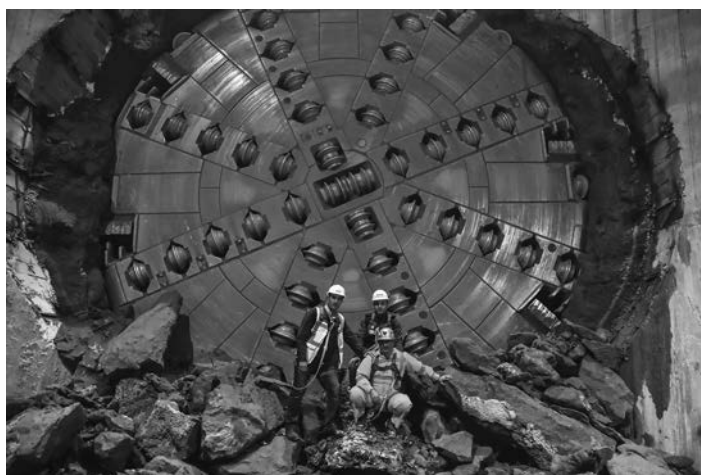
Figure 5.38 Breakthrough of an XRE TBM (8.7 m diameter) in Mexico City used to construct a 5.8 km long wastewater tunnel. (Courtesy of The Robbins Company.)
