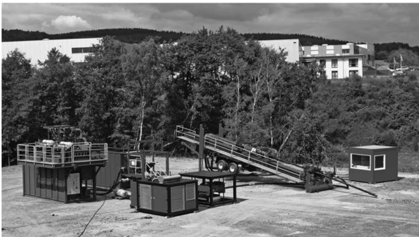
Figure 5.98 Example of a large HDD rig and associated facilities, pumps and mud recirculation system. (Courtesy of Prime Drilling HDD-Technology.)
