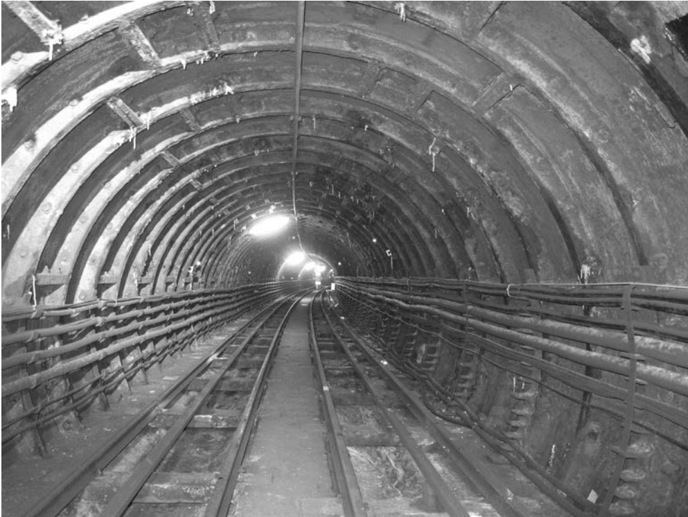
Figure 8.47 Post Office Tunnel. (Photo Credit: Crossrail Ltd., used with permission.)
