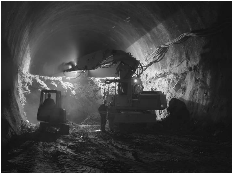
Figure 5.54 Example of a NATM crown and bench excavation during the construction of the Katschberg Tunnel, Austria.
