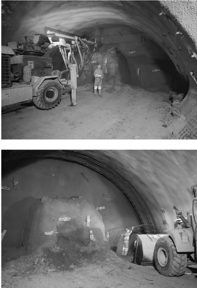
Figure 4.13 Installation of temporary dowels into the tunnel face during the construction of the Lainzer Tunnel LT31 in Vienna, Austria.
