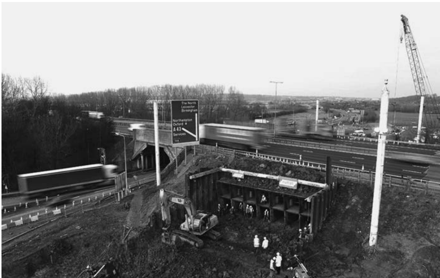
Figure 5.83 Completion of the jacking process showing the shield. (From Allenby D. and Ropkins J.V.T. 2004. The use of jacked-box tunnelling under a live motorway. Proceedings of the Institution of Civil Engineers, Geotechnical Engineering . Courtesy of BAM Nuttall Ltd. and John Ropkins Ltd. used with kind permission from ICE Publishing and Dr. Douglas Allenby, 2004, Figure 3 (p. 232); Figure 5 (p. 234); Figure 9 (p. 237) and Figure 10 (p. 237).)
