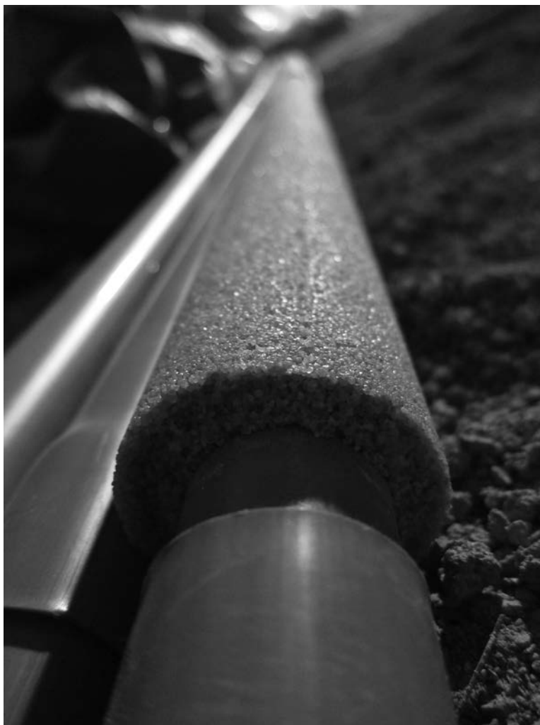
Figure 8.45 Resin bonded filter. (Photo Credit: Crossrail Ltd., used with permission.)
