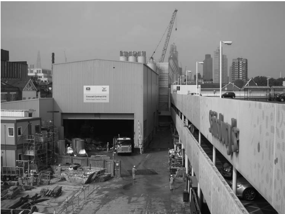
Figure 8.32 Whitechapel Station, acoustic shed. The construction site was formerly a car parking area. To replace this lost space, the two-storey car park on the right was built. In the background, the City of London is also visible. (Photo Credit: Crossrail Ltd., used with permission.)
