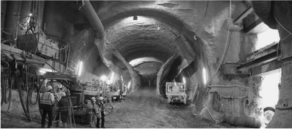
Figure 8.20 30 m of total cross section (on the RHS, in the opening to the oval section, the remainder of the lower most bracing can be seen still in place).
