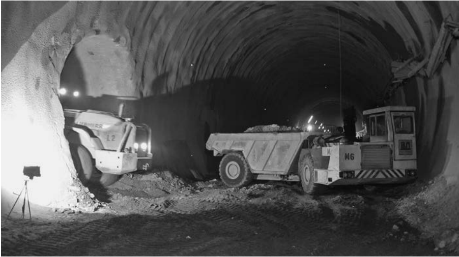
Figure 5.56 Example of mucking equipment used during the construction of one of the emergency cross-passages of the Katschberg Tunnel, Austria.
