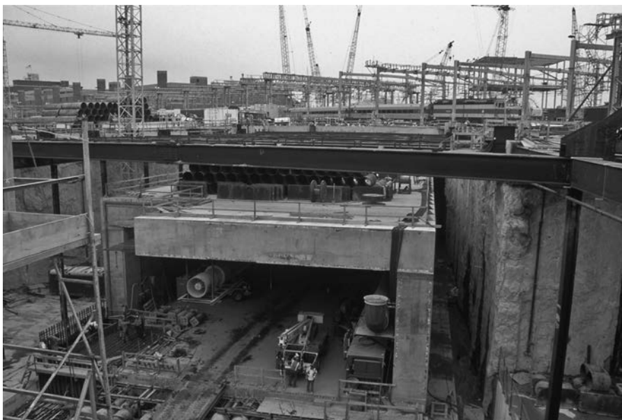
Figure 5.85 One of the jacked box tunnels during the jacking process, note the cover depth above the tunnel and rail road lines at the ground surface. (Courtesy of Massachusetts Turnpike Authority.)
