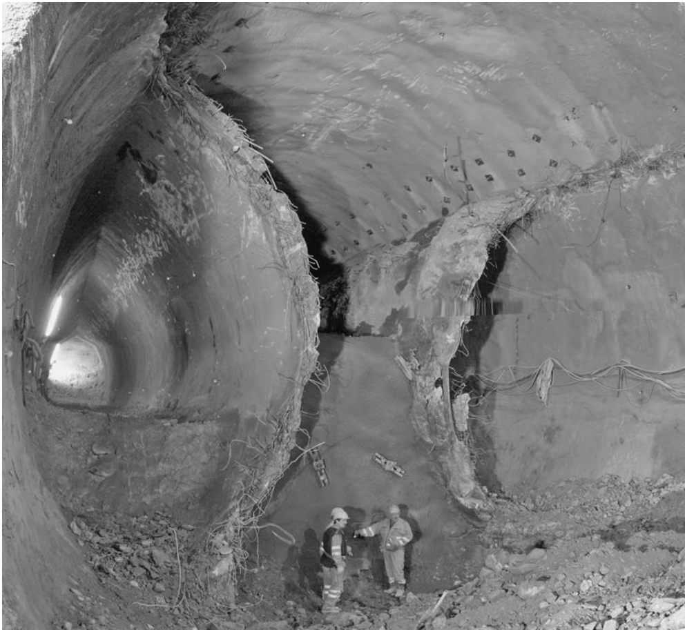
Figure 8.23 Construction of the invert at the total cross section (excavation Centre Drift 2 and demolition of inner walls of the sidewall drift).
