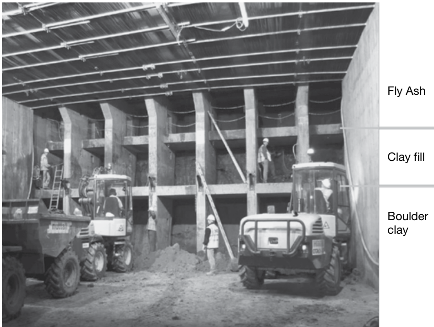
Figure 5.81 Rear view of the cellular-reinforced concrete shield (annotation indicates the ground strata). (Allenby and Ropkins 2004, courtesy of BAM Nuttall Ltd. and John Ropkins Ltd.)
