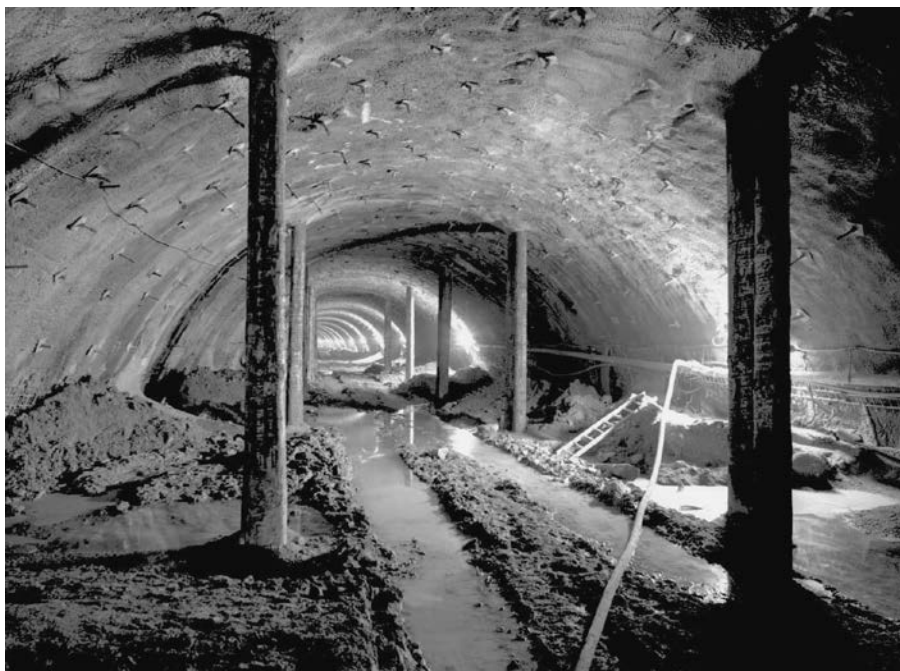
Figure 7.25 Emergency support measures using tree trunks during the tunnel excavation (Eggetunnel, crown heading). (Courtesy of Professor Dr-Ing. habil. Reinhard B. Rokahr, photograph by Ulrich Mertens DFA DGPh, Atelier für Kunst und Fotografie, Hamburg.)
