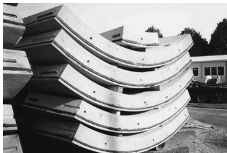
Figure 4.23 Example of an expanded segmental lining set for one complete ring.
