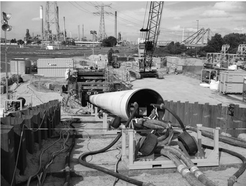
Figure 5.101 One of the worksites on the North-South gas pipeline in the Netherlands, using the Direct Pipe method of construction. (Courtesy of Herrenknecht.)
