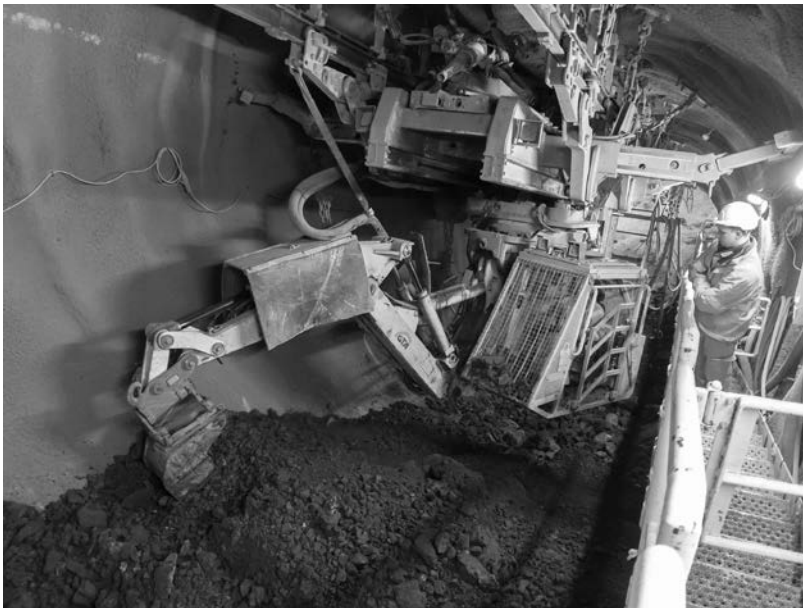
Figure 8.50 The Uphill Excavator. Following the excavation of one advance, the muck is moved down the escalator shaft (ES2, Liverpool Street Station). (Photo Credit: Crossrail Ltd., used with permission.)
