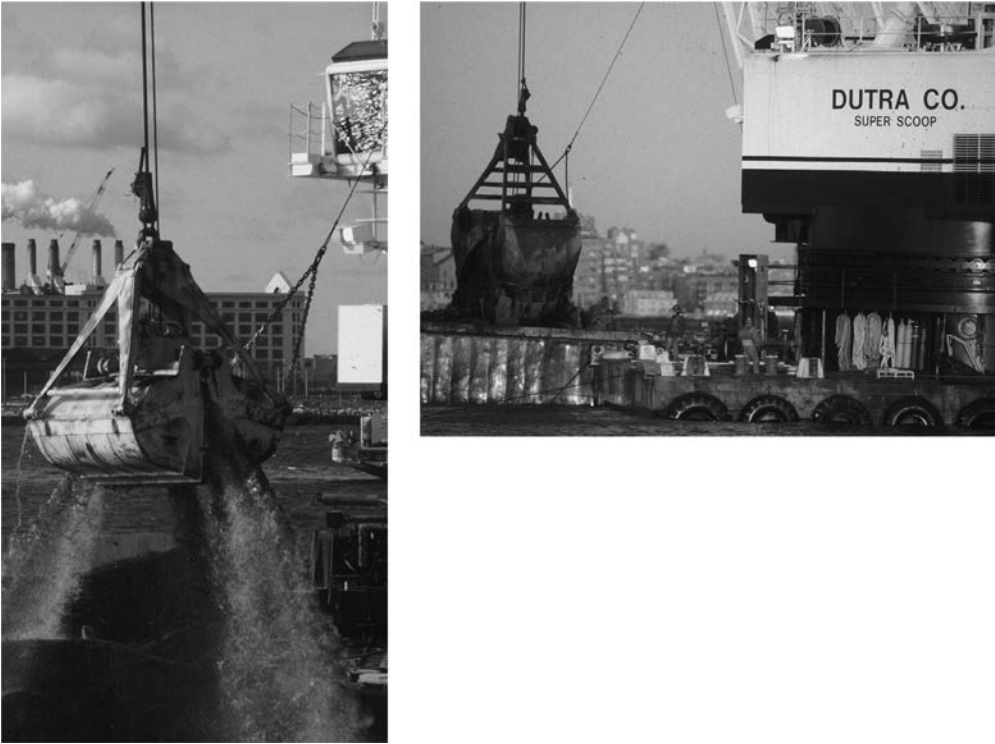
Figure 5.74 The trench was excavated using floating cranes with grab excavators. (Courtesy of Massachusetts Turnpike Authority.)
