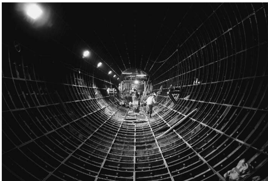
Figure 4.25 Example of bolted SGI lining as used in London, UK. (Courtesy of BeMo Tunnelling GmbH Innsbruck.)
