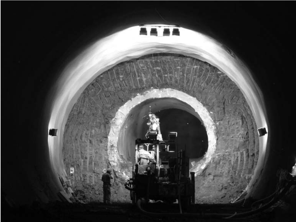
Figure 8.34 Tunnel enlargement of the previously excavated Pilot tunnel. In this photograph, the excavation of this advance has just been completed and it is ready for the concrete spraying. The tunnel face shows the exposed London Clay. (Photo Credit: Crossrail Ltd., used with permission.)
