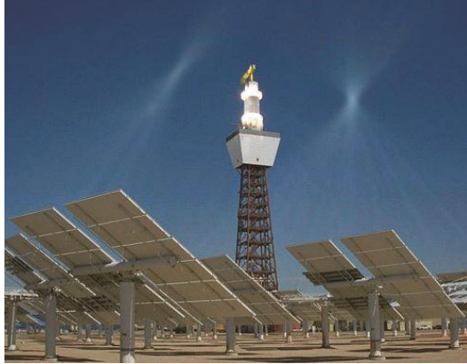
Figure 2.2. Solar thermal plant.
