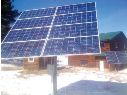
Figure 2.5. Remote standalone PV system.
