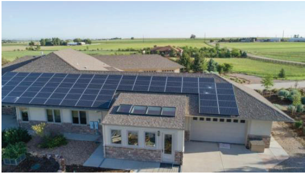
Figure 2.6. Residential PV system.
