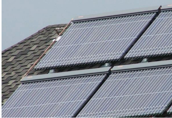
Figure 7.4. Vacuum tube collector.
