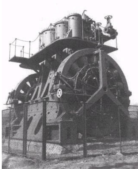
Marine-type, triple expansion, engine-driven dynamo as it appeared in 1889, before its restoration and relocation inside the Henry Ford Museum. Today, the engine and dynamo operate with the assistance of an electric motor.
