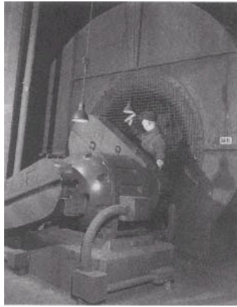
One of eighty-four fans at the Holland Tunnel. Courtesy Port of New York Authority.
