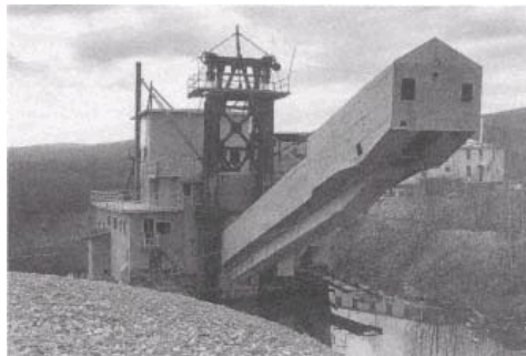
Fairbanks Exploration Company Gold Dredge No. 8.
