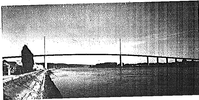
Figure 1.58 Brotonne Bridge, France
