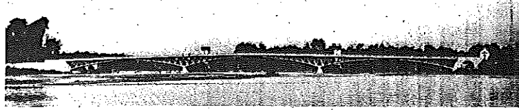
Figure 1.22 Allier River Bridge, Le Veudre, France
