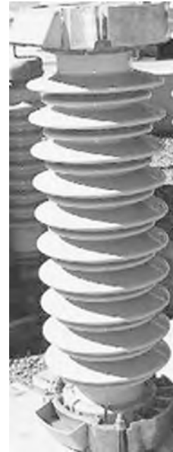
FIGURE 10.8 Post insulators.
