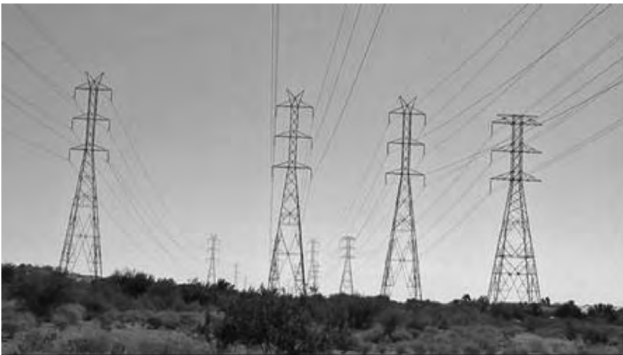
FIGURE 19.3 Transmission line corridor.
