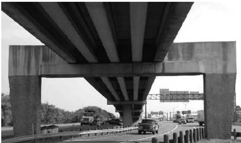
FIGURE 5.13 Bent cap.
