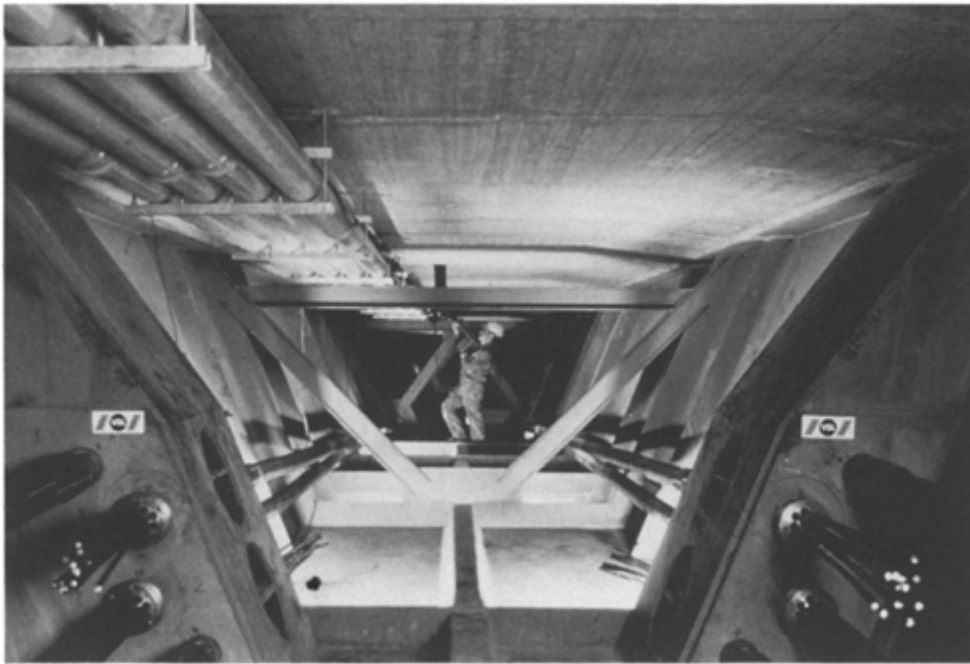
Figure 1.5 Externally prestressed bridge deck ( courtesy VSL International ).
