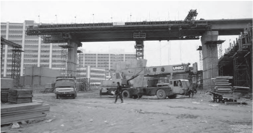
Figure 12.2 Contract 304 HKMTR: semi-mechanised falsework (Photo: Robert Benaim)
