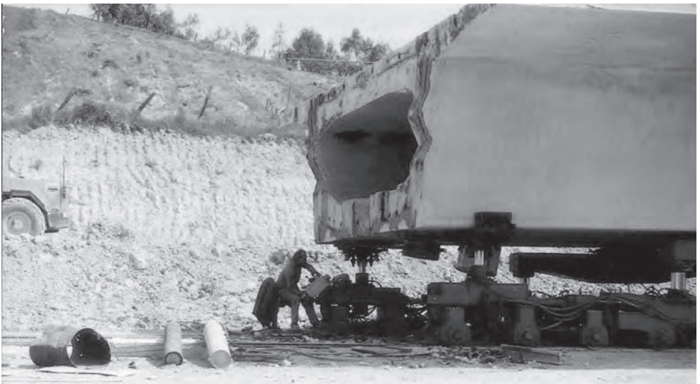
Figure 15.46 Poggio Iberna Viaduct, Italy: deck unit on its transporter (Photo: David Benaim)
