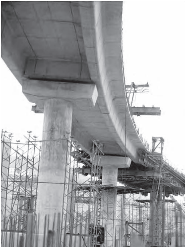
Figure 12.8 Contract 308 of the HKMTR, Tai Ho Viaduct: twin rib deck with pier diaphragms (Photo: Robert Benaim)
