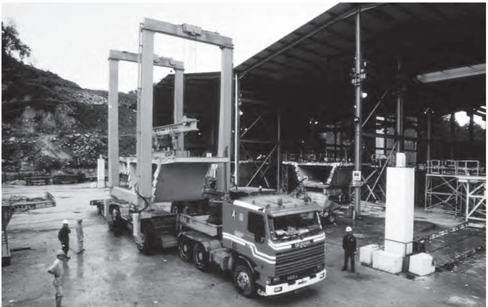
Figure 14.15 STAR: segment handler (Photo: Benaim)
