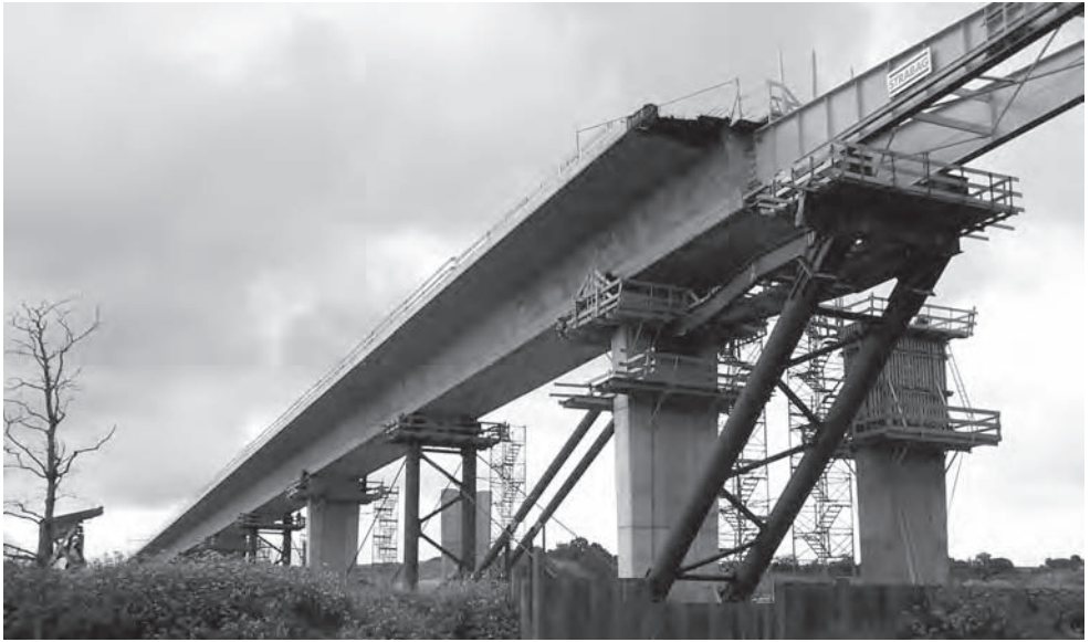
Figure 15.37 Blackwater Viaduct, Ireland (Photo: Strabag SE)
