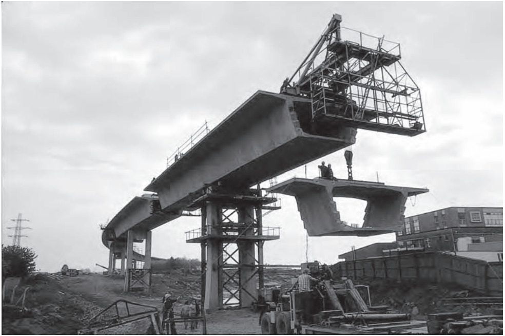
Figure 7.26 East Moors Viaduct (Photo: Benaim)
