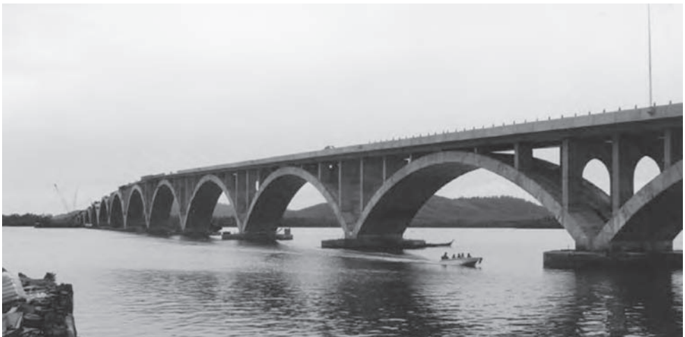
Figure 17.16 Bridge over Sungai Dinding (Photo: Benaim)
