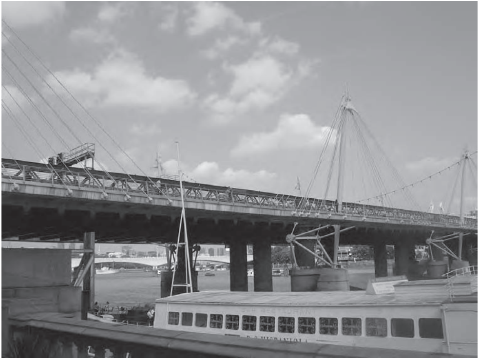
Figure 1.11 Hungerford Footbridge (Photo: Robert Benaim)
