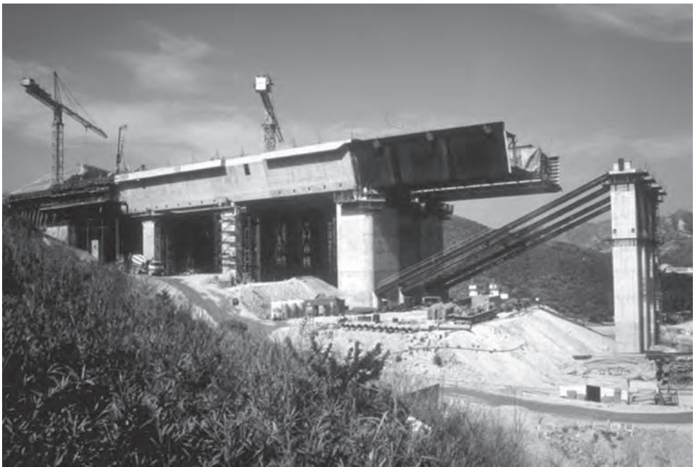
Figure 15.42 Kap Shui Mun Bridge, Hong Kong: launching of approach span (Photo: Benaim)
