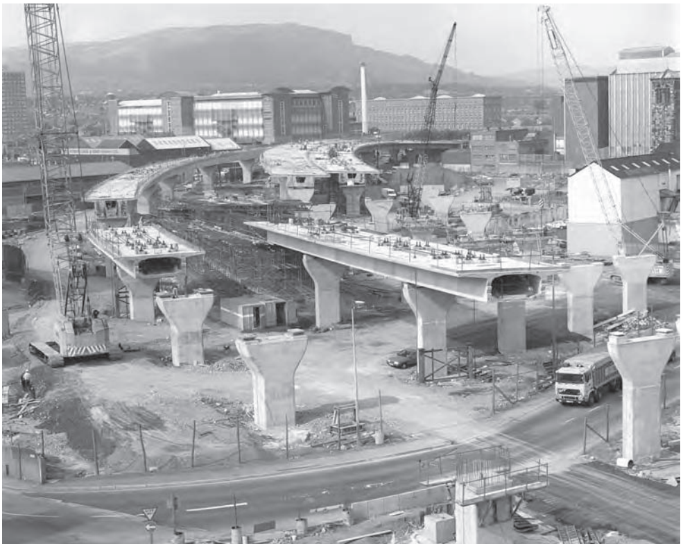
Figure 15.29 Belfast Cross Harbour Bridges: the flexibility of crane erection (Photo: Graham-Farrans JV/Esler Crawford)
