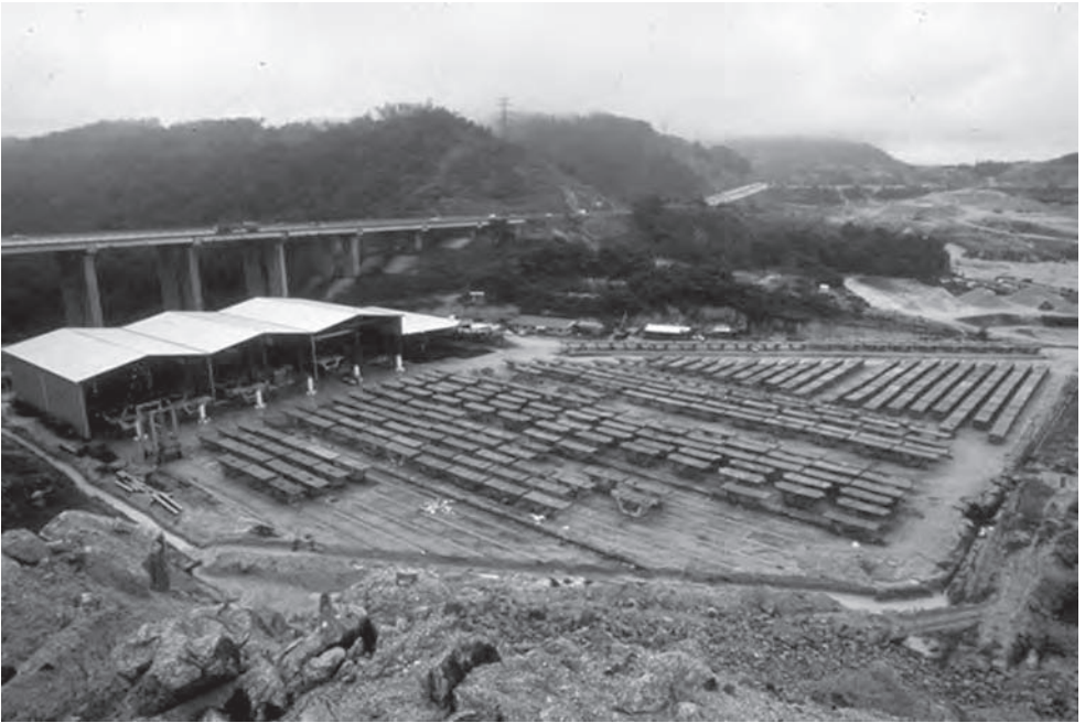
Figure 14.16 STAR: casting factory and storage (Photo: Benaim)
