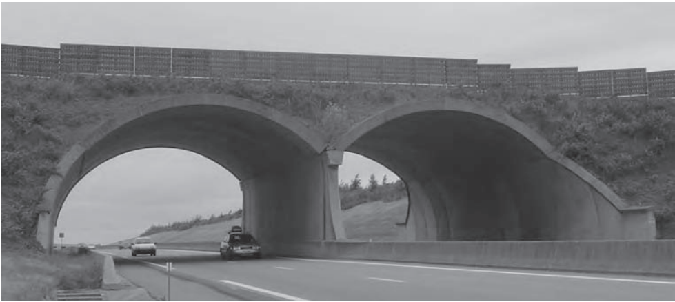
Figure 17.11 Bridge on A16, France (Photo: Robert Benaim)
