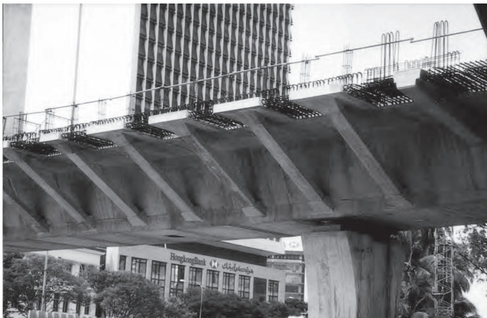
Figure 9.11 STAR Viaduct: stitches between precast segments (Photo: Benaim)
