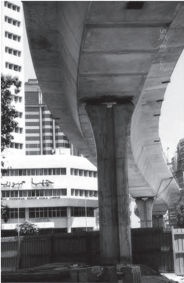
Figure 7.11 Pier of STAR Viaduct (Photo: Benaim)
