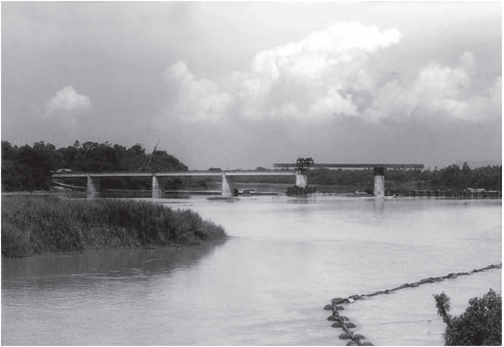
Figure 10.13 Sungai Kelantan Bridge (Photo: Robert Benaim)
