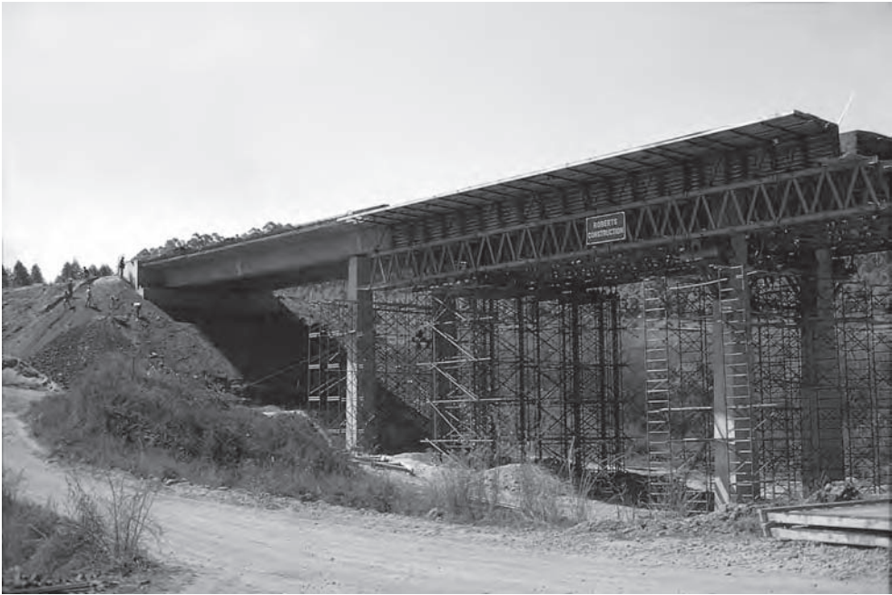
Figure 12.16 Doornhoek Bridge: typical falsework for span-by-span construction of short bridge (Photo: Arup)
