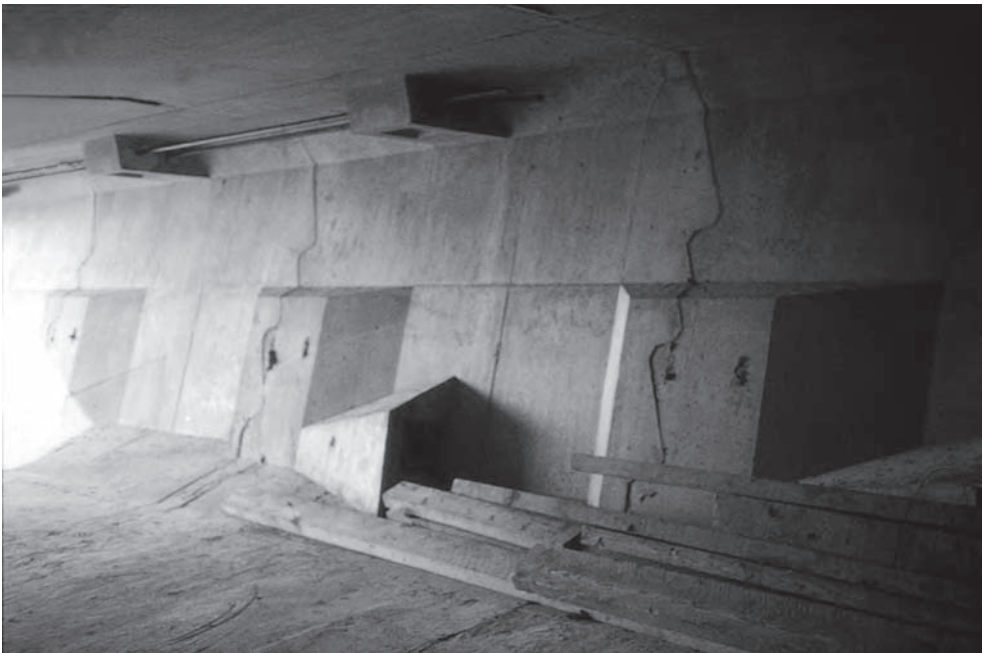
Figure 15.21 East Moors Viaduct: interior of box showing temporary stressing bars, web thickenings for face anchors and blisters for Stage 2 cables (Photo: Robert Benaim)
