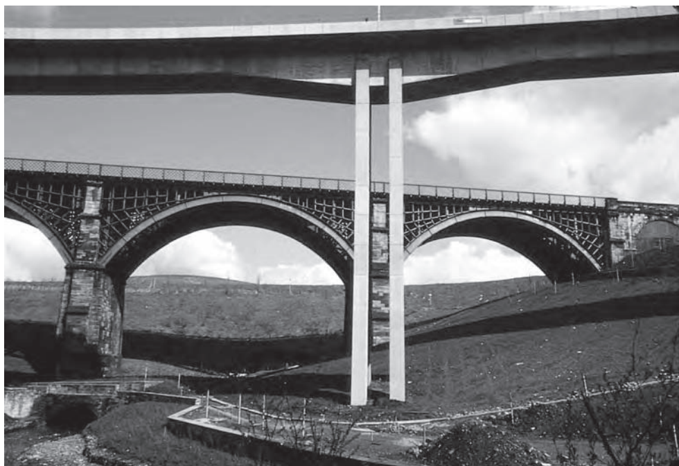
Figure 7.24 Byker Viaduct: valley piers (Photo: Robert Benaim)
