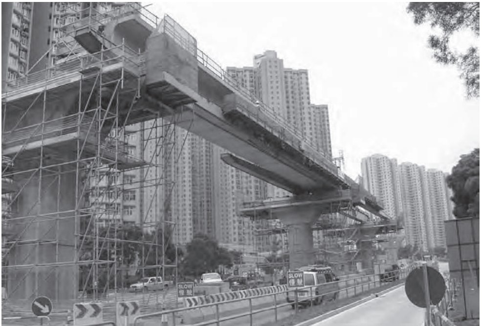
Figure 15.7 East Rail Gantry (Photo: VSL, www.vsl.com )
