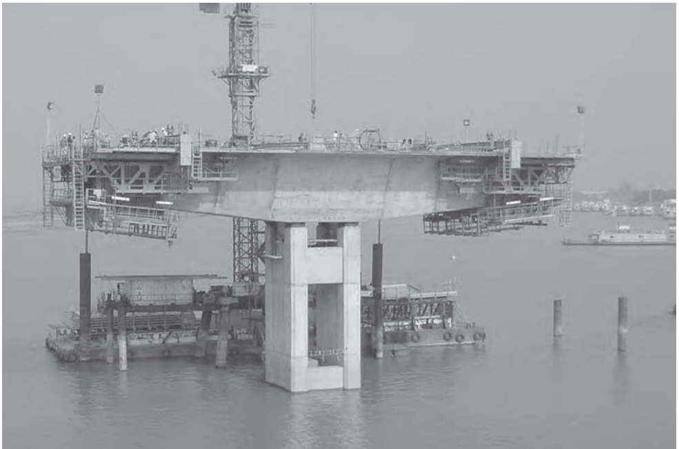
Figure 15.16 Bhairab Bridge, Bangladesh: underslung falsework travellers (Photo: Roads and Highways Department, Government of Bangladesh and Edmund Nuttall)
