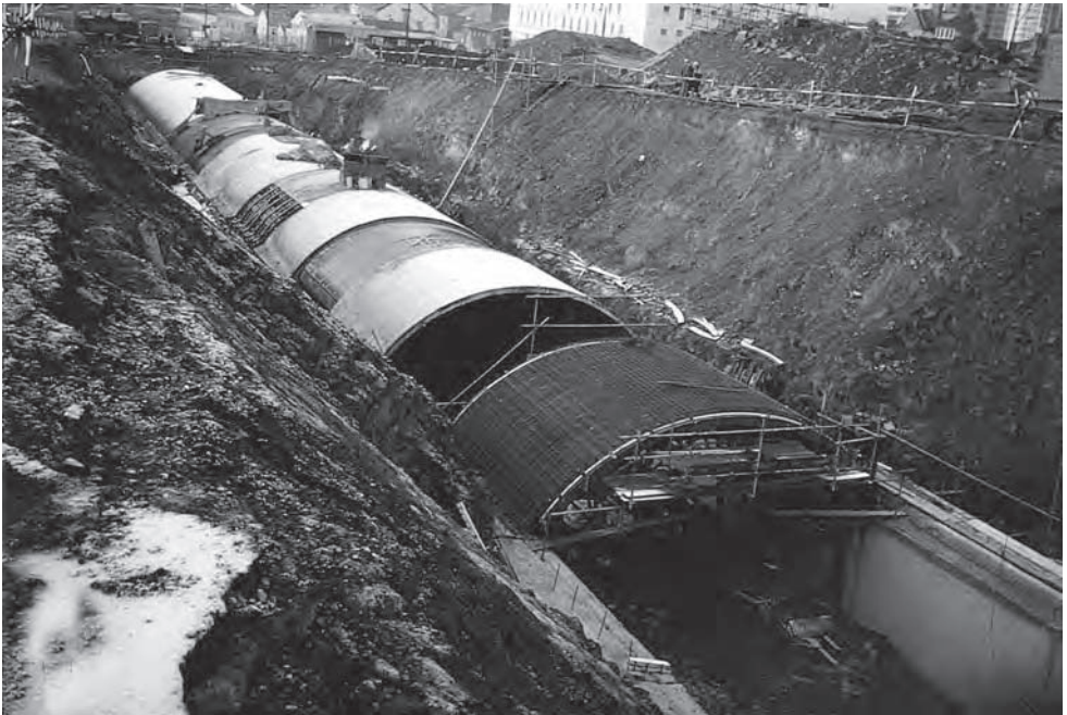
Figure 17.7 Byker Tunnel under construction (Photo: Robert Benaim)
