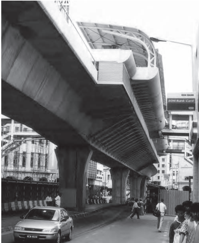
Figure 9.9 STAR Viaduct: elevated station (Photo: Benaim)
