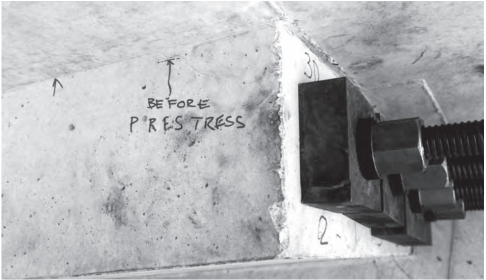
Figure 5.9d Typical prestress anchors: bar anchors (Photo: Benaim)
