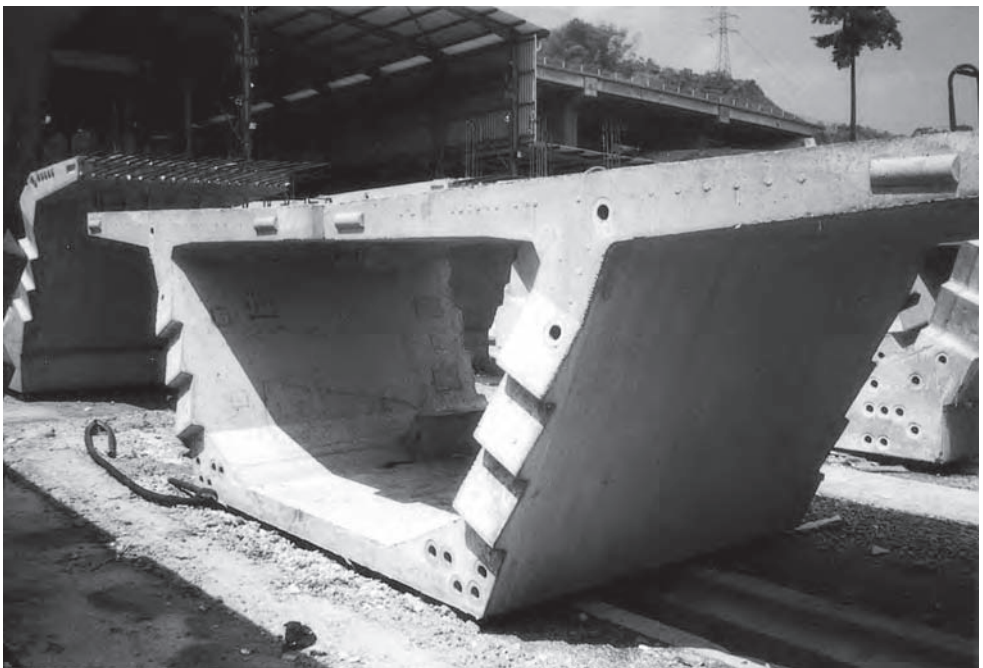
Figure 14.9 STAR: typical segment details (Photo: Benaïm)
