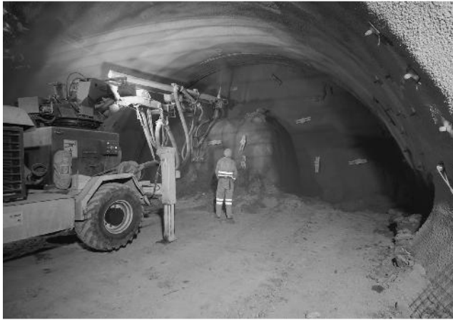
Figure 4.13 Installation of temporary dowels into the tunnel face during the construction of the Lainzer Tunnel LT31 in Vienna, Austria
