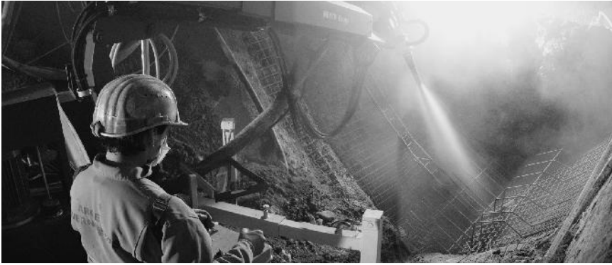
Figure 4.18 Sprayed concrete application of the invert of a side wall drift during the construction of the Lainzer Tunnel LT31 in Vienna, Austria
