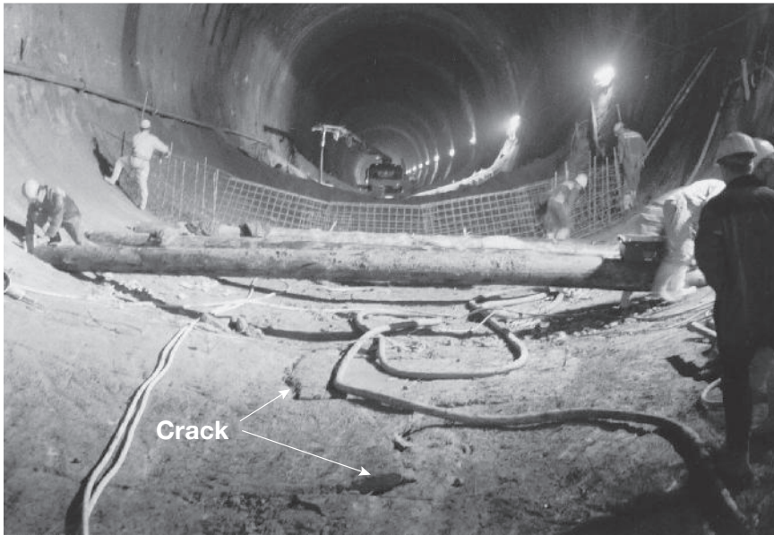
Figure 8.2 Contingency measures in the form of tree trunks at the completed cross section due to cracking after removing the backfill
