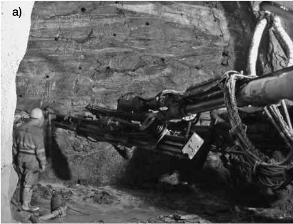
Figure 5.36 Examples of drilling blasting holes, a) and b) for an emergency cross passage, Katschberg Tunnel, Austria, c) for the Spillvatten Tunnel, Goeteborg, Sweden (an 8 km sewer tunnel, cross sectional area 11 m 2 , ground included granitic gneiss)
