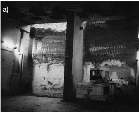
Figure 5.80 a) Excavating the lower half of a 10 m high face through frozen, waterbearing sands and gravels, and b) Webster Schaeff excavating machines used on the Boston jacked box tunnels (Clayton et al. 2001) (courtesy of BAM Nuttall Ltd and John Ropkins Ltd)
