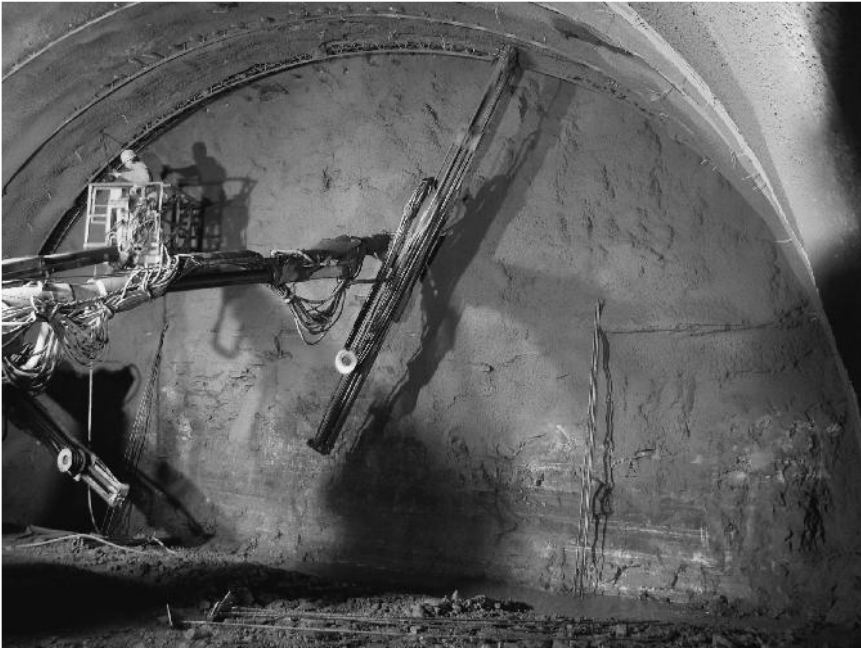
Figure 4.9 Anchor installation associated with sprayed concrete lining, HKT Tunnel, Germany (courtesy of ALPINE BeMo Tunnelling GmbH Innsbruck)
