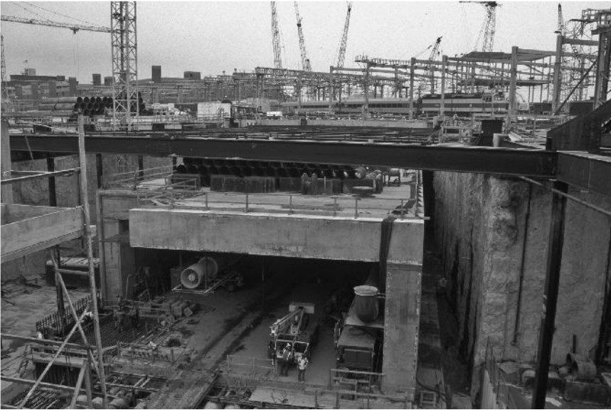
Figure 5.78 One of the jacked box tunnels during the jacking process, note the cover depth above the tunnel and rail road lines at the ground surface (courtesy of Massachusetts Turnpike Authority)
