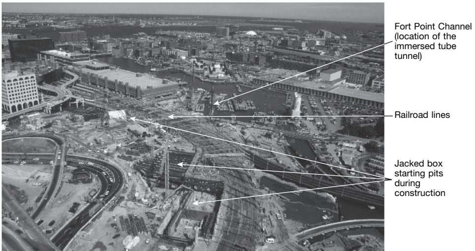
Figure 5.77 An overview of the jacked box sites in Boston showing the railroad lines and Fort Point Channel (courtesy of Massachusetts Turnpike Authority)
