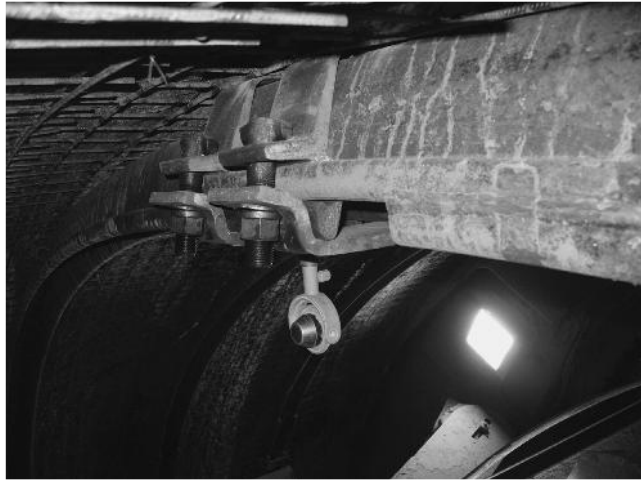
Figure 4.21 A load connection fitting for steel girders as used on the Gotthard Base Tunnel (Faido)
