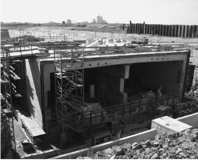
Figure 5.64 Construction of one of the elements for the Limerick immersed tube tunnel in Ireland (courtesy of COWI A/S)
