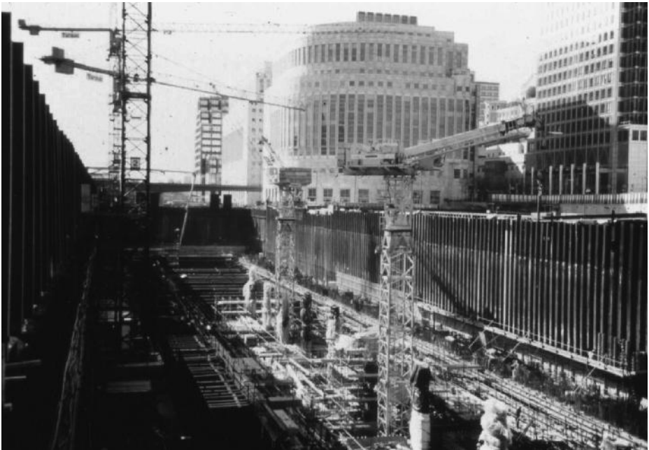
Figure 5.51 Canary Wharf Station during construction on the London Underground Jubilee Line Extension, UK
