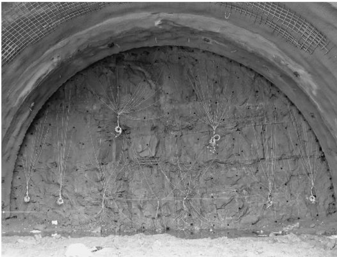
Figure 5.41 Example of a face ready to blast in the Heidkopf Tunnel, Germany
