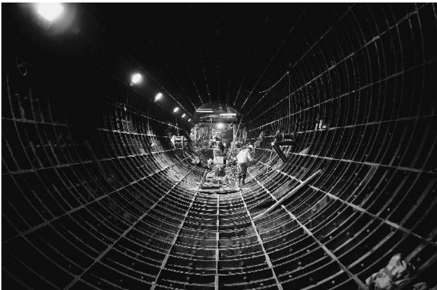
Figure 4.25 Example of bolted SGI lining as used in London, UK (courtesy of ALPINE BeMo Tunnelling GmbH Innsbruck)
