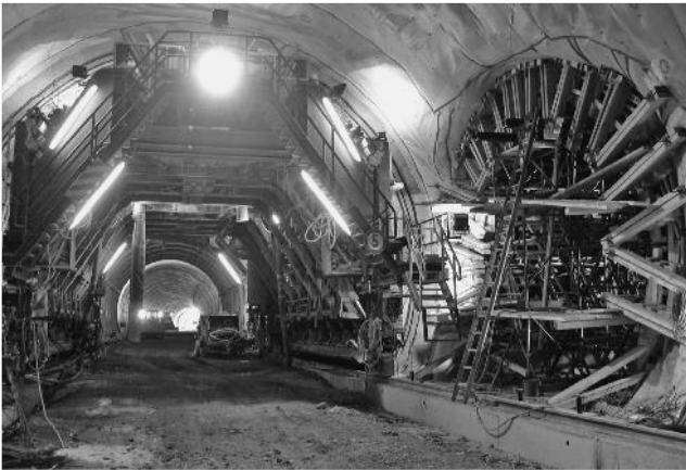
Figure 4.29 Inner lining construction, including waterproofing as used for the emergency cross-passage, Heidkopf Tunnel, Germany (courtesy of ALPINE BeMo Tunnelling GmbH Innsbruck)
