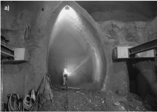
Figure 4.18 Sprayed concrete application of the invert of a side wall drift during the construction of the Lainzer Tunnel LT31 in Vienna, Austria
