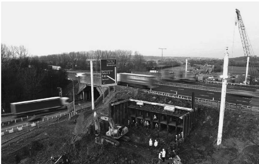
Figure 5.76 Completion of the jacking process showing the shield (Allenby and Ropkins 2004, courtesy of BAM Nuttall Ltd and John Ropkins Ltd)
