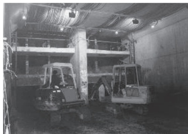
c) Rear view of the face during excavation
