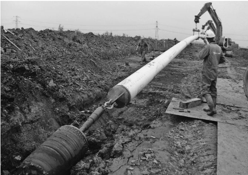
Figure 5.89 Pullback operations showing back reamer and final pipe (courtesy of Prime Drilling HDD-Technology)
