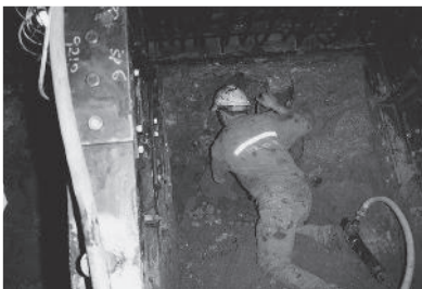
b) Hand mining in a top compartment through very weak, loose sand and silt
