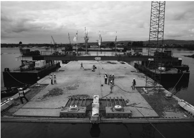
Figure 5.65 One of the elements for the Limerick immersed tube tunnel being towed into position ready for sinking (courtesy of COWI A/S)
