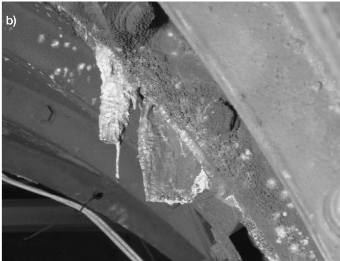
Figure 8.13 a) Existing Piccadilly Line tunnels, SGI-Segments (LHS), Concrete Segments (RHS), b) existing Piccadilly Line Eastbound Tunnel, stalactites on the SGI-Segments
