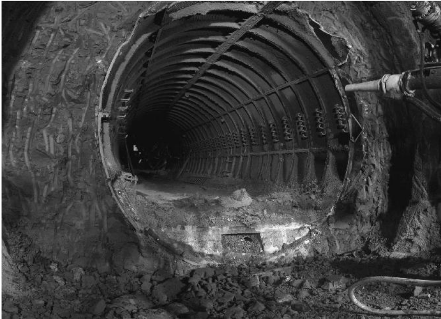
Figure 8.12 View into the unplugged existing Piccadilly Line Eastbound Turnout tunnel
