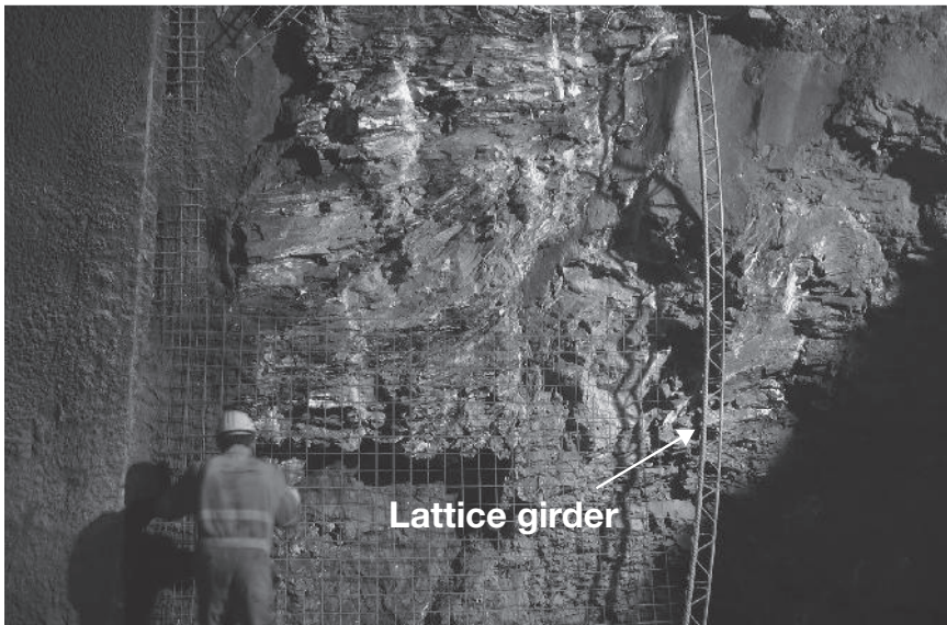
Figure 4.20 Mesh installation and a lattice girder arrangement
