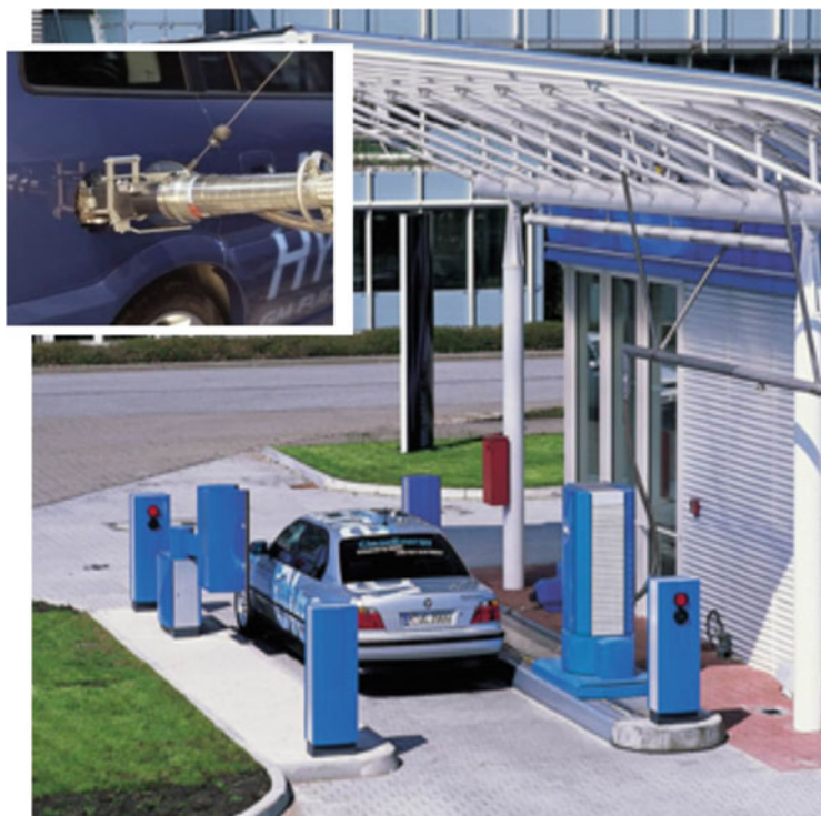
Fig. 3.33 Hydrogen filling station for automobiles (Source: BMW)
