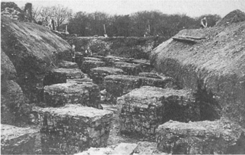
Figure 6.3 Abandoned room and pillar workings for coal, which have been exposed during excavations at a locality in Central Scotland. Notice how close to the soil cover the workings extend. (Reproduced by kind permission of Mr George Archibald, Subsidence Engineer, National Coal Board.)
