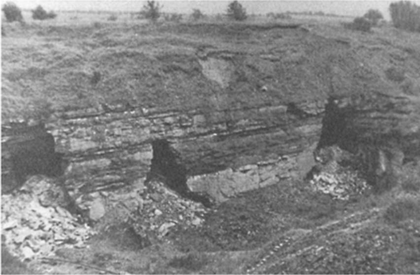
Figure 6.4 A quarry face showing abandoned room and pillar workings which are partially collapsed. The voids (rooms) have migrated upwards as the roofs have collapsed, and in one case (extreme left of photograph) only a thin layer of rock separates the void from the overlying soil. (Reproduced by kind permission of Messrs J.W.H. Ross & Co., Mining Engineers, Glasgow.)
