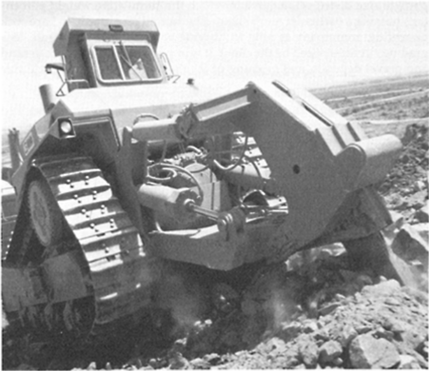
Figure 7.5 Excavation of rocks using a mechanical ripper. (Photograph by courtesy of the Caterpillar Tractor Company, Illinois.)
