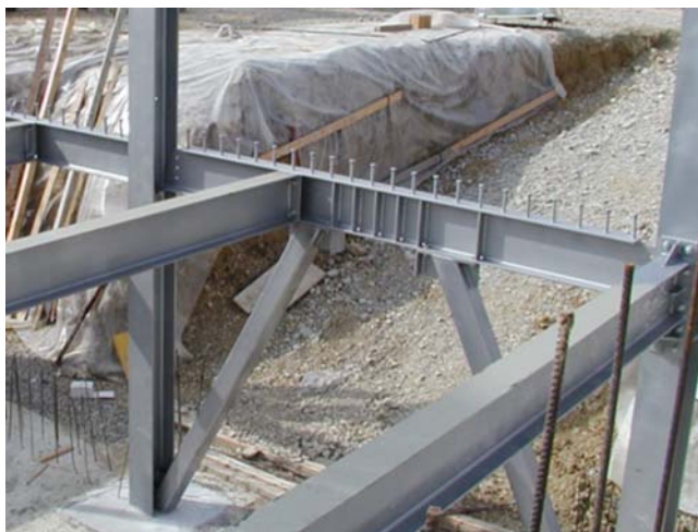
Figure 4.109 Links in eccentric braces.
