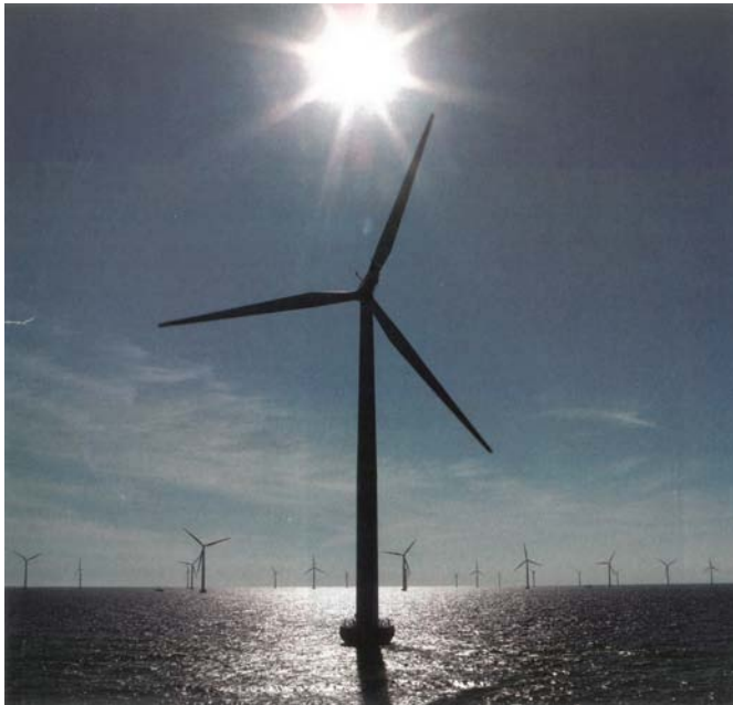
Fig. 3.14 The 165.6 MW Nysted offshore wind farm, Denmark, using 72 Bonus turbines, opened at the end of 2003. How will the larger wind farms of the future meet the challenges of interconnection and energy storage? NYSTED HAVMOELLEPARC. 14
