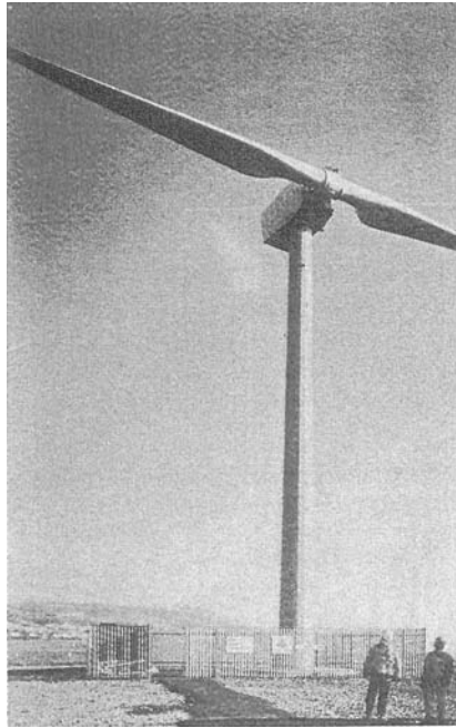
Fig. 3.11 3 MW wind machine in Orkney, Scotland. 12
