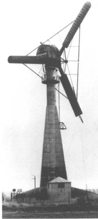
Fig. 3.7 Restored Gedser wind turbine 200 kW at 33.6 mph. (Ref. Danish Wind Industry Association, 2009) ( http://www.talentfactory.dk/en/pictures/juul.htm ).
