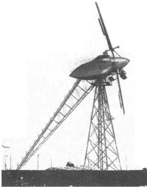
Fig. 3.3 Russian wind-turbine; 100 kW (24.6 mph rated wind speed).
