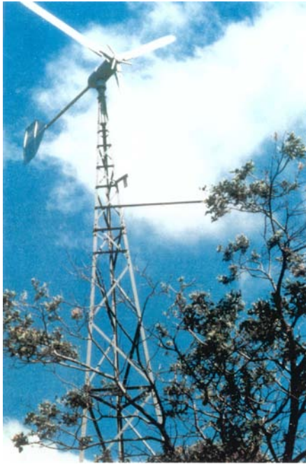
Fig. 3.2 Propeller driven wind turbine for generating electricity [Photographed by author WS in Wisconsin, USA-1997].
