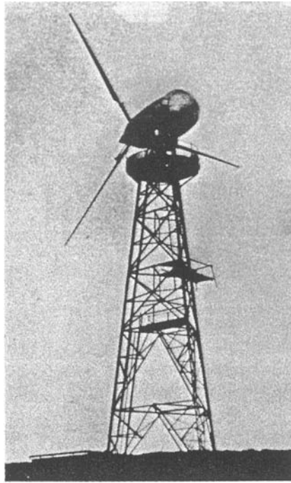
Fig. 3.5 British wind-turbine, John Brown design located on Cape Costa in the Orkney Islands; 100 kW (35 mph rated wind speed).
