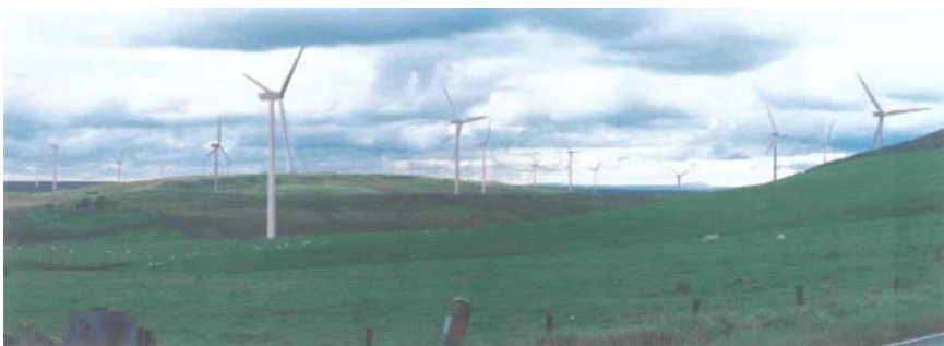
Fig. 3.17 Whitelee Wind Farm, Eaglesham, Scotland, 140, 2.3 MW, 3-blade cantilevered construction (courtesy Scottish Power).
