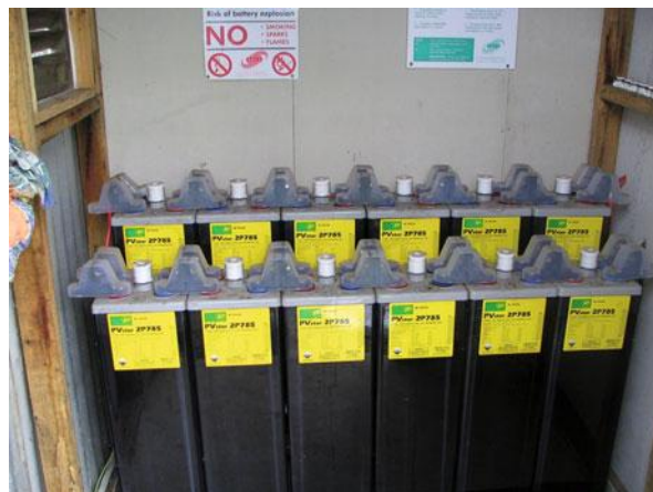
Figure 1.6 Batteries in a stand-alone solar electric system
