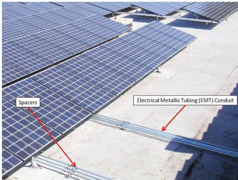
Figure 14.13 The DC conductors are housed inside a metallic conduit as per the guidelines in the National Electric Code (NEC). The 2008 NEC states that conduit in direct contact with a roof under full sunlight will experience an internal temperature of 33°C (60°F) above ambient while conduit that is mounted between 0.5 and 3.5 inches above the roof (as in this system) will experience an internal temperature of 22°C (40°F) above ambient. It is for this reason that the installers have mounted the conduit several inches above the surface of the roof
