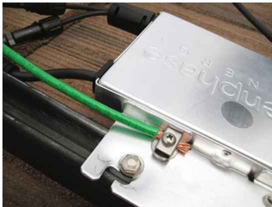
Figure 14.22 In accordance with the National Electric Code (NEC), all metallic parts of the PV array which could potentially become exposed to live current are mechanically bonded to the earth (grounded/earthed) using either bare copper or green cables. This includes the PV module frames, mounting system and conduit as well as the individual micro-inverters as shown above
