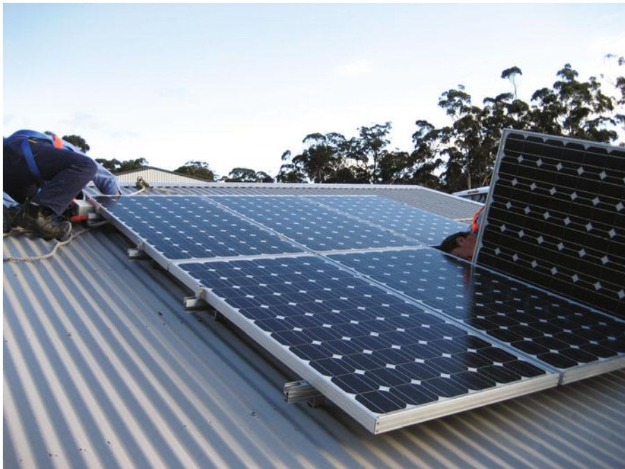
Figure 6.6 Corrugated metal roof installation
