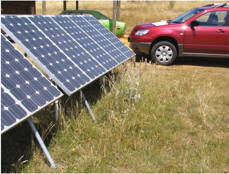
Figure 6.14 The grass is low now, but if it grows high enough it could shade the array
