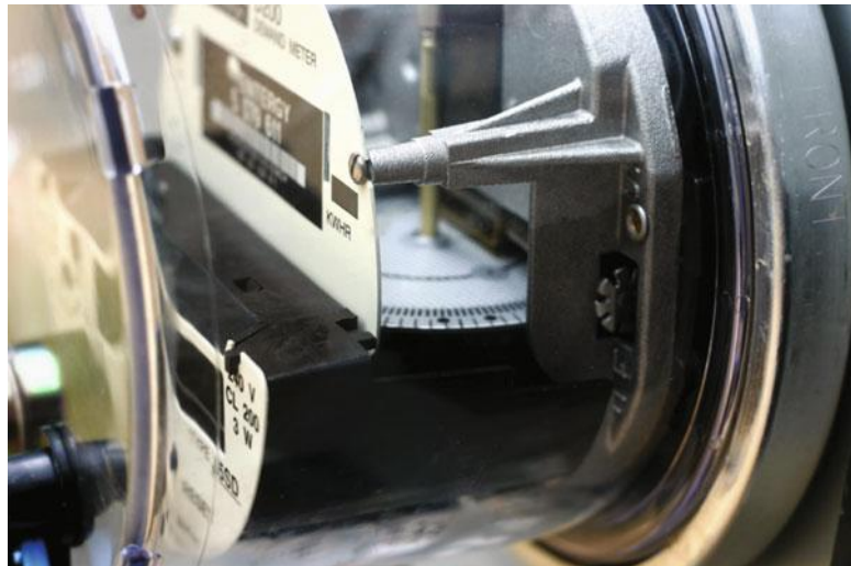
Figure 5.36 The single rotating disc in the centre of this net meter is clearly visible: when electricity is consumed (by loads within the building) it rotates forwards and when electricity is produced (by the PV system) it rotates backwards
