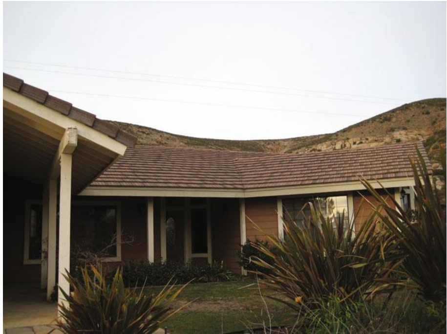
Figure 14.20 This flat tile residential rooftop presented some common design challenges for a typical PV system using a centralized inverter; there are several different roof orientations with suitable solar access (south, west and east). In addition there is not enough available space on each roof face to mount a complete series string, meaning that modules within the same series string would have to be mounted facing different orientations. Modules facing different directions would receive different amounts of solar radiation (see Chapters 7 and 9) and hence have different power outputs. As discussed in Chapter 4, it is not desirable to connect PV modules with very different outputs in series and the total power output of the system would suffer
