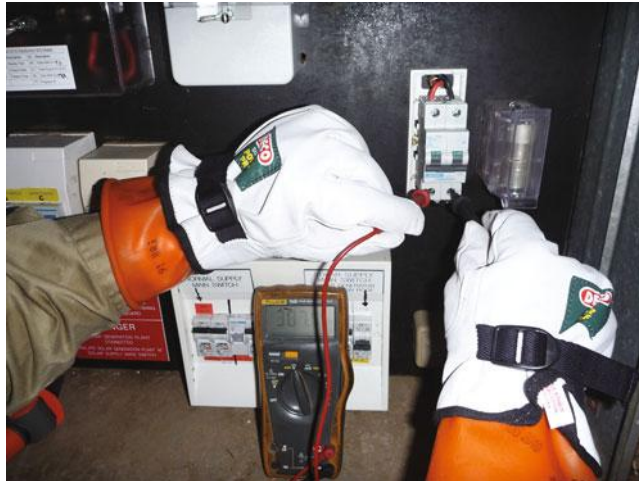
Figure 11.1 An electrician checks the open-circuit voltage and polarity of an array cable entering the inverter
