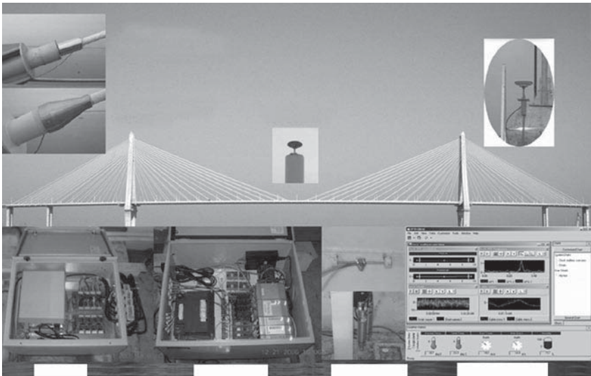
5.20 Real-time health monitoring system in Zhanjiang Bay Bridge.
