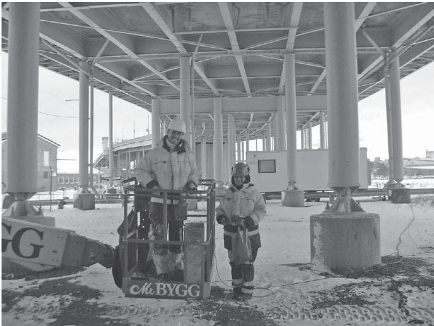
11.10 View to bridge girders and installation equipment and team.
