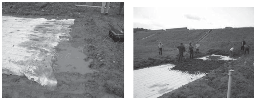
14.4 Sensor-based geotextile mat during the installation on a construction site of a gravity dam in Solina/Poland (textile developed by STFI e. V. Chemnitz/Germany). Photo: BAM.
