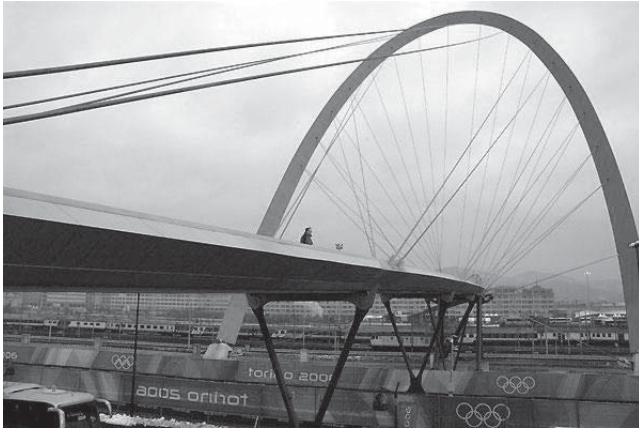
8.17 Aerial view of the Lingotto Bridge's single arch suspended deck.
