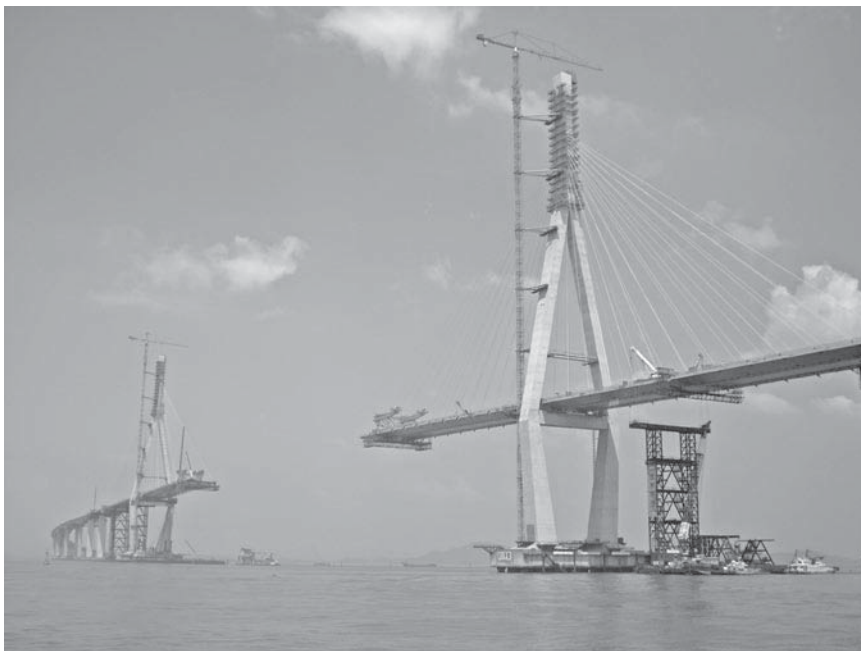
1.2 Construction of Incheon Bridge, Incheon, Korea. SHM can be applied during construction to monitoring of such a unique structure's response during this stage.
