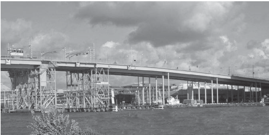
11.9 View of the Göta Bridge.
