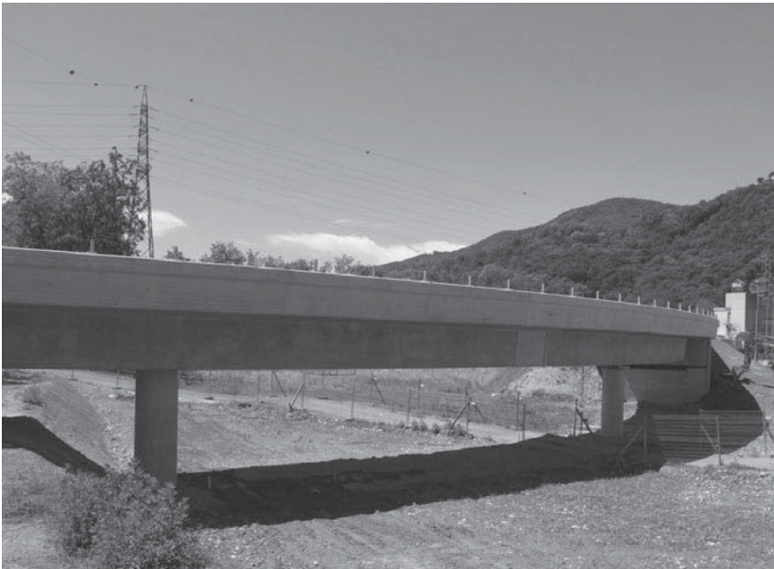
11.3 View of the main span of the Ricciolo Bridge (courtesy of SMARTEC).
