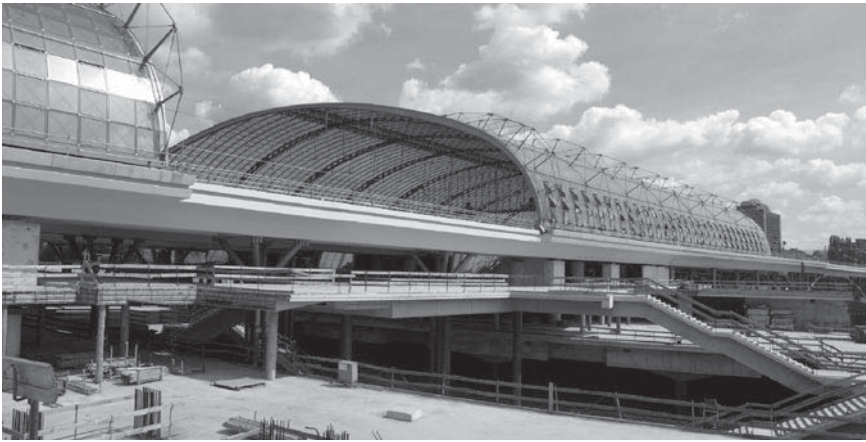
14.5 Upper area of the new Berlin Central railway station during construction. Photo: BAM.
