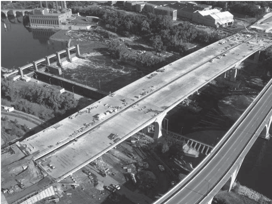
11.1 View of the completed I-35W St. Anthony Falls Bridge (courtesy of Minnesota Department of Transportation).
