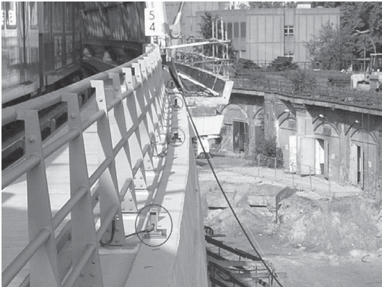
14.8 Components of the laser-based levelling (encircled).
