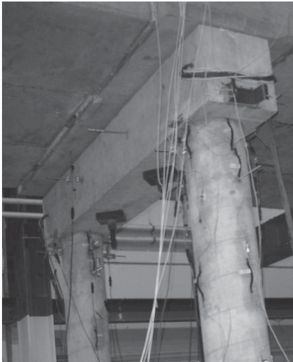
8.23 Crack sensors on a bridge pier.
