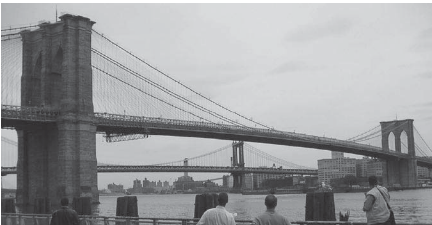
1.3 Brooklyn Bridge, New York City, NY. Brooklyn Bridge as an old landmark structure is an ideal candidate for monitoring for continued use, maintenance, repair and retrofit.
