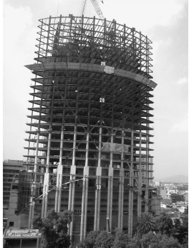
Figure 9.29: Torre Mayor under construction showing the cross-braced dampers. (Courtesy of Douglas P. Taylor of Taylor Devices, Inc.)
