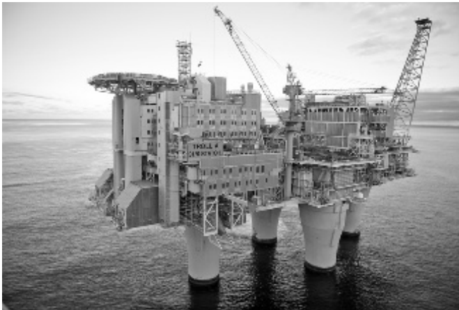
Figure 1.2: The Troll A concrete platform for production of gas is located off the west coast of Norway. The platform was a televised sensation when it was towed into the North Sea in 1996, where it is operated by Statoil. Not only is it among the largest and most complex engineering projects in history, it is the largest object ever to be moved across the surface of the Earth. Troll A has an overall height of 472 m and weighs 656,000 tons. The bottom of the platform is on the seafloor 303 m below the surface. The walls of Troll A's legs are over 1 m thick. (Courtesy of Helge Hansen/StatoilHydro)
