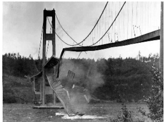
Figure 11.17: In many physics textbooks, the Tacoma Narrows Bridge collapse is presented as an example of forced resonance, with the wind providing an external periodic frequency that matched the bridge's natural structural frequency. The cause of failure was more complicated and involved aeroelastic flutter. (University of Washington Libraries, Special Collections, UW21422)
