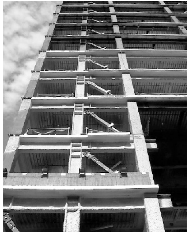
Figure 1.5: Large dampers installed on each floor at the Buddhist Headquarters in Taipei, Taiwan. (Courtesy of Douglas P. Taylor of Taylor Devices, Inc.)
