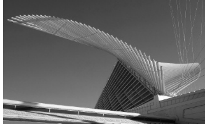
Figure 7.33: The Milwaukee Art Museum's signature wings form a movable sunshade with a 66-m wingspan. The wings consist of 72 steel fins, pinned at a central spine and ranging in length from 8 to 32 m. The mass of the structure is 81,600 kg. It takes 3.5 minutes for the wings to open or close. Sensors on the fins monitor wind speed and direction; if the speed exceeds 37 km/h for more than 3 s, the wings close. (Photograph by M. Nagurka)
