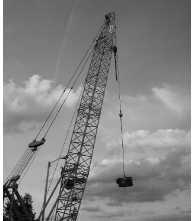
Figure 1.20: The load carried by a crane displays pendular motion. The load exhibits oscillatory motion when the crane is moving the load. (Brookfield, WI; photograph by M. Nagurka)
