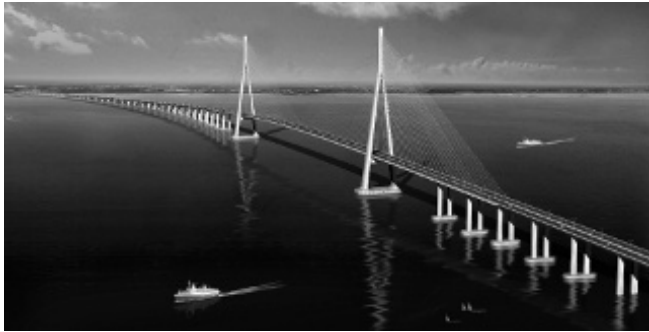
Figure 3.1: The Sutong Changjiang River Bridge in China is a cable-stayed bridge with a span of 1.1 km (the world's longest from 2008-2012). Its two side spans are 300 m each, and the two towers of the bridge are 306 m high. The total bridge length is 8.2 km. (Courtesy of Douglas P. Taylor of Taylor Devices, Inc.)
