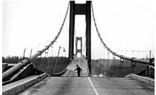
Figure 11.16: The 1940 Tacoma Narrows Bridge spanned the Tacoma Narrows strait of Puget Sound. It opened to traffic on July 1, 1940, and collapsed into Puget Sound on November 7. It twisted and vibrated violently on the day of the collapse. (James Bashford Press Photos, PH Coll. 290.30 University of Washington Libraries. Special Collections Division)
