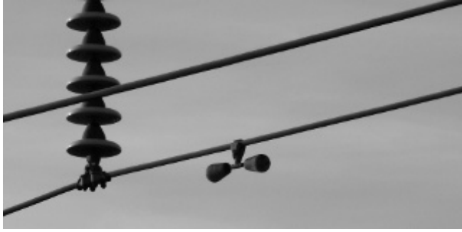
Figure 6.26: A Stockbridge damper on a power line is shown at the center. The damper is placed near a suspension clamp, at a distance less than one-half wavelength of the highest frequency mode to be absorbed. (Glendale, WI; photograph by M. Nagurka)
