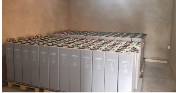
Fig. 8.21 Battery bank from a mini-grid in Nigeria; the battery bank has not been connected to the DC bus (courtesy of GVE Projects)
