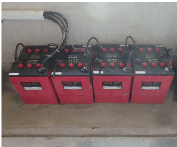
Fig. 8.4 A 48 V battery bank for a mini-grid in Kenya consisting of a string of eight, six-volt batteries arranged in series (courtesy of author)
