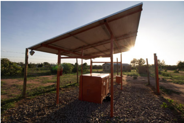
Fig. 12.24 The PV array of the Ighombwe mini-grid with the batteries, inverters and meters securely located in the housing below (courtesy of PowerGen)
