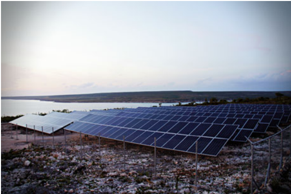
Fig. 12.22 A 200 kW PV array is used in the Môle-Saint-Nicolas mini-grid (courtesy of Sigora Haiti)
