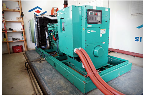
Fig. 5.11 A 660 kW diesel gen set used to power a mini-grid in Haiti (courtesy of Sigora Haiti)
