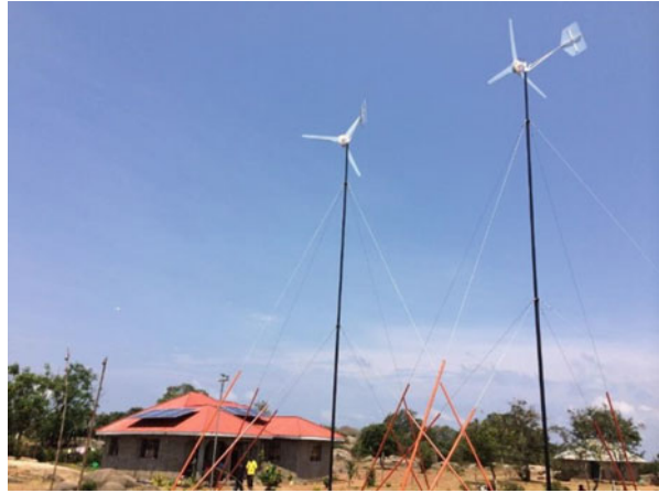
Fig. 4.2 A small-scale, decentralized, hybrid mini-grid using wind and solar power in Muhuru Bay, Kenya (courtesy E. Patten)
