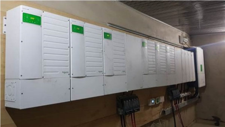
Fig. 9.3 The control room of a large mini-grid in Nigeria, consisting of inverters, charge controllers, and system monitoring equipment (courtesy of GVE Projects)
