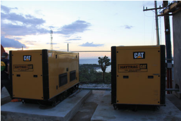
Fig. 12.21 Two 100 kW gen sets used in the Môle-Saint-Nicolas mini-grid (courtesy of Sigora Haiti)
