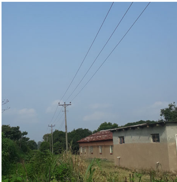
Fig. 3.4 A typical three-phase overhead distribution line (courtesy of R. Ngoma)
