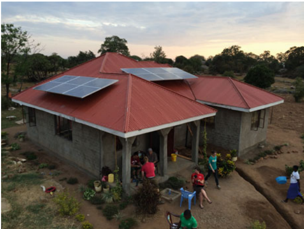
Fig. 7.1 A 3 kW PV array split into two strings in Kenya (courtesy E. Patten)
