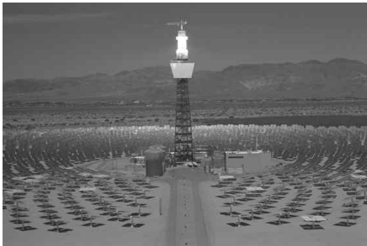
FIGURE 7.4 Solar Two, Barstow, California. Notice receiver, which is white hot, and the oil storage tanks at the bottom. (From Sandia Labs.)
