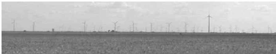
FIGURE 14.1 Visual aspect of wind turbines near Hitchland, Texas, looking south. Foreground: 3.2 km to one turbine, Vestas V 90, 3 MW, diameter = 90 m, 80-m tower; middle left, 4.4 km to row of eight Suzlon wind turbines, 1.25 MW, diameter = 64 m, 72-m tower; background, John Deere 4 wind farm, 9.5 km to first row, 14.5 km to back row, 38 Suzlon wind turbines, 2.1 MW, diameter = 88 m, 80-m tower.
