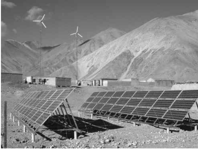
FIGURE 15.3 Hybrid system (54 kW) for village power, Subashi, Xingiang Province, China. (Courtesy of Charlie Dou.)
