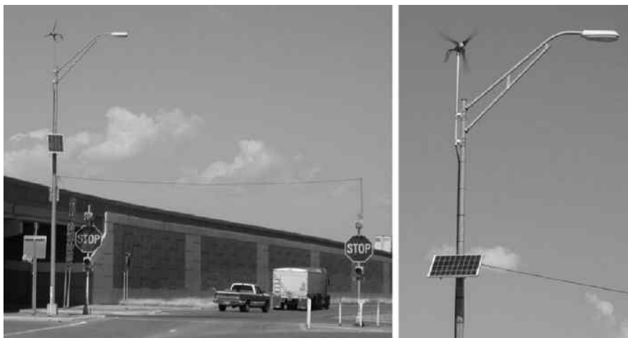
FIGURE 9.20 PV-wind powers streetlight and flashing red lights at stop signs, McCormick Road on I27 between Canyon and Amarillo, Texas.
