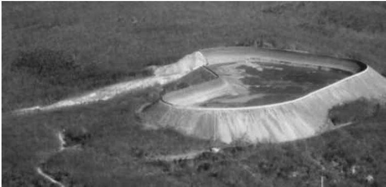
FIGURE 13.8 Upper reservoir for Taum Sauk pumped hydro plant, Missouri. Notice scouring of the creek due to wall failure. (Source: U.S. Geological Survey photo 037.)
