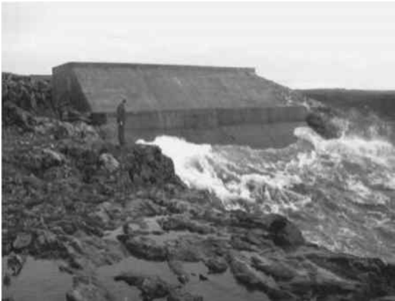
FIGURE 12.26 LIMPET on Islay Island, Scotland, 500 kW; installed 2000. (Courtesy of Voith Hydro Wavgen.).
