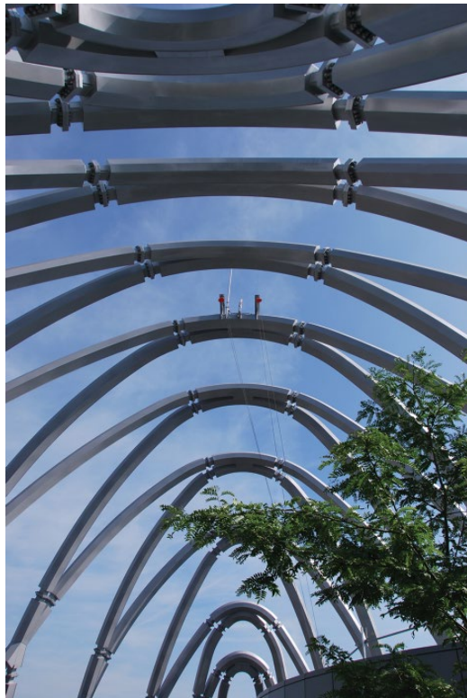
Figure 1 View from below the arched steel structure. © ConstruirAcier.
