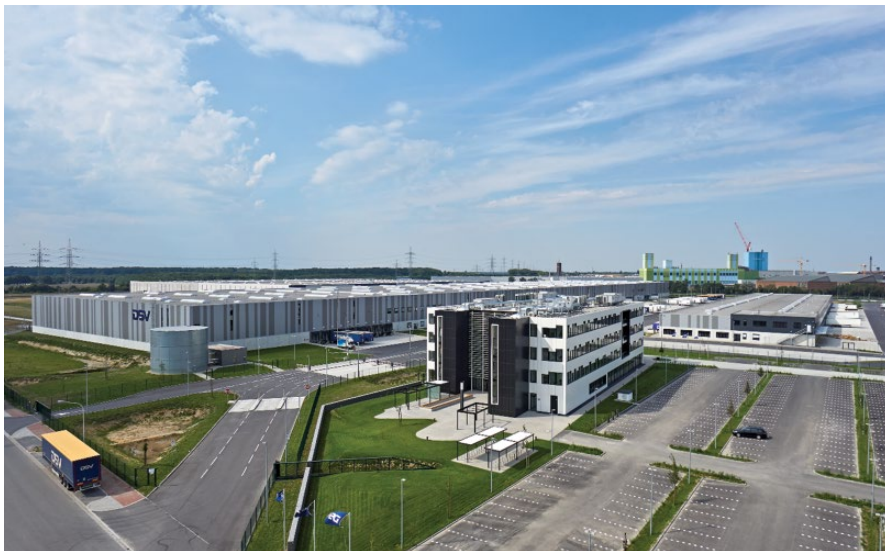
Figure 1 The office is located near the logistics building – 6570 m 2 office space, 300 m 2 basement. © Goldbeck.
