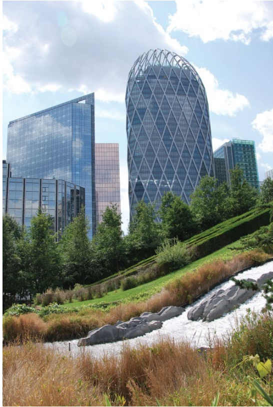
Figure 2 General view of the D2 Tower in Paris – La Défense. © ConstruirAcier.
