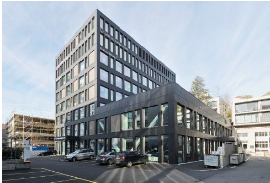
Figure 1 Residential and office building in Baden. © rgp Rolf Graf & Partner Architekten.
