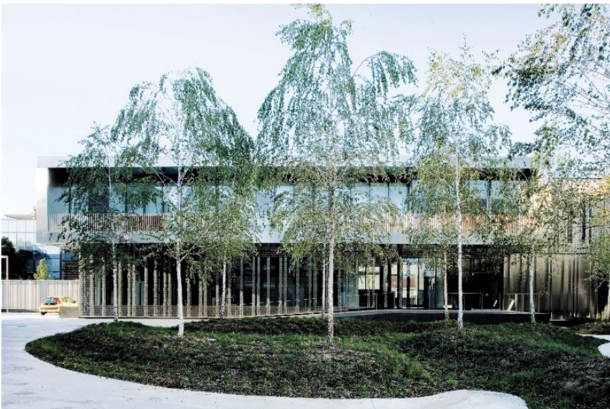
Figure 3 View from the inside of the production side. © Filippo Romano/Stahlbau Pichler.
