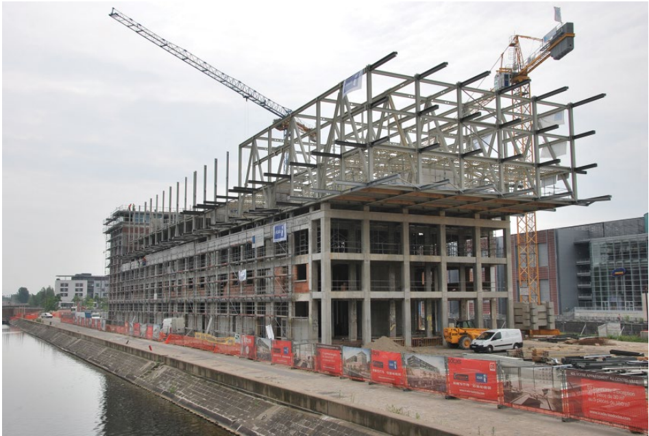
Figure 2 The old Seegmuller warehouse, built in 1932, was refurbished and enlarged by a three-storey steel structure. © ConstruirAcier.
