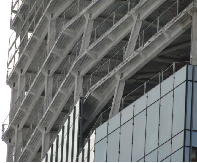
Figure 2 Steel structure with inclined columns. © bauforumstahl.
