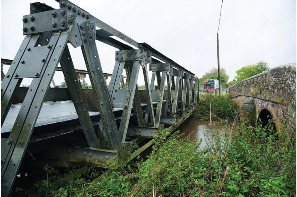
Figure 4.35 This hot-dip galvanized Callender-Hamilton bridge was built 1942 at Lydlinch. © Iqbal Johal.
