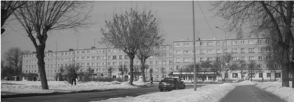
Figure 4. Multi-storey residential housing along Liela Street (Source: photo by the author, 2006)
