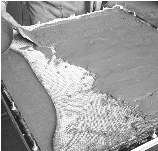
Figure 2. Concrete shell fabrication reinforced by three layers of knitted glass fiber fabric
