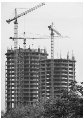
Figure 1. Multifunctional complex “Z-towers” construction process
