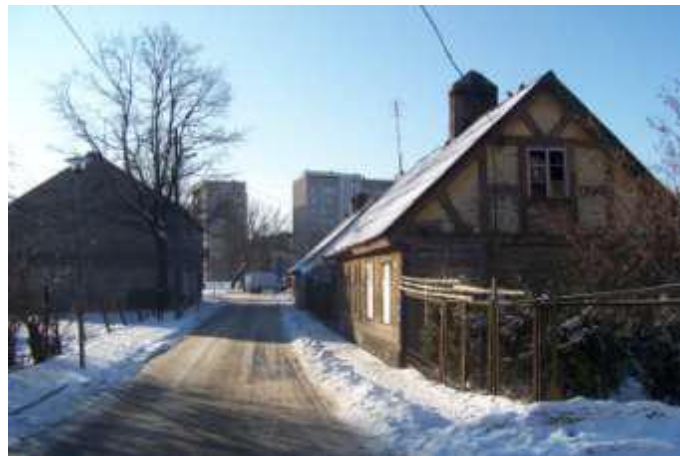
Figure 10. In the junction of M. Dambja street and Kr. Barona street, the tree canopy exceeds the building's crest (Author's photo, 2012)
