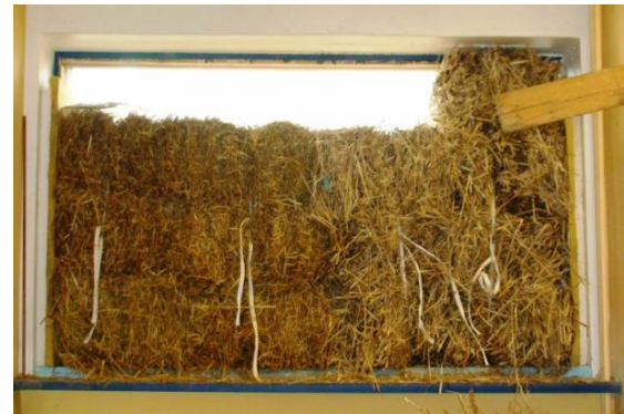
Figure 3. The building of a test wall of straw and reed bales (walls S3 and S4)
