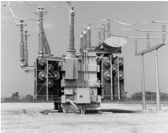
FIGURE 4.2 Installed view of a three-phase, 345/161 kV autotransformer with power ratings of 214/285/357 MVA for OA/FA/FOA. (Courtesy of North American Transformer, Milpitas, CA.)
