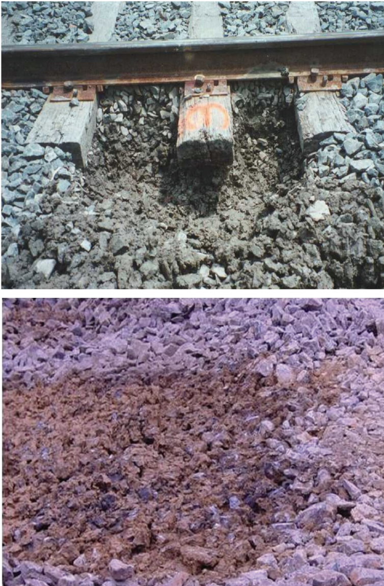
Figure 1.4 Fouled ballast.
