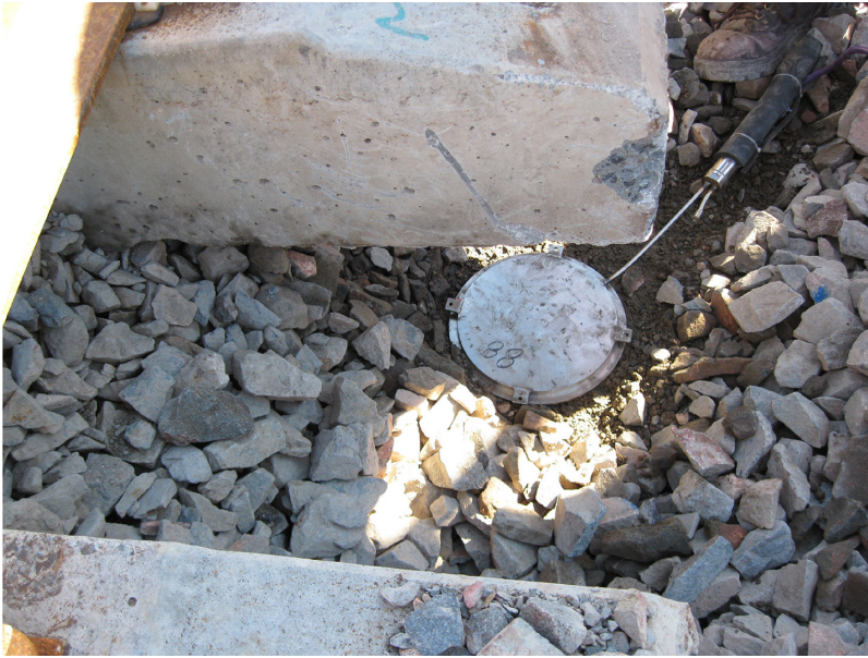
Figure C6 Installation of pressure cell at the ballast–capping interface at Singleton.
