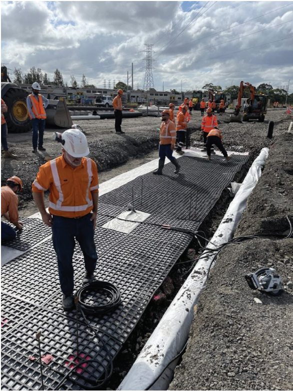
Figure E3 Installing energy-absorbing rubber seams with instrumentations.
