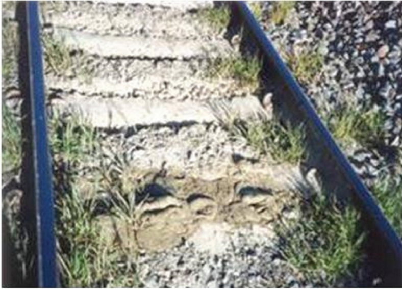
Figure 1.8 Dried slurry deposited around the sleepers.
