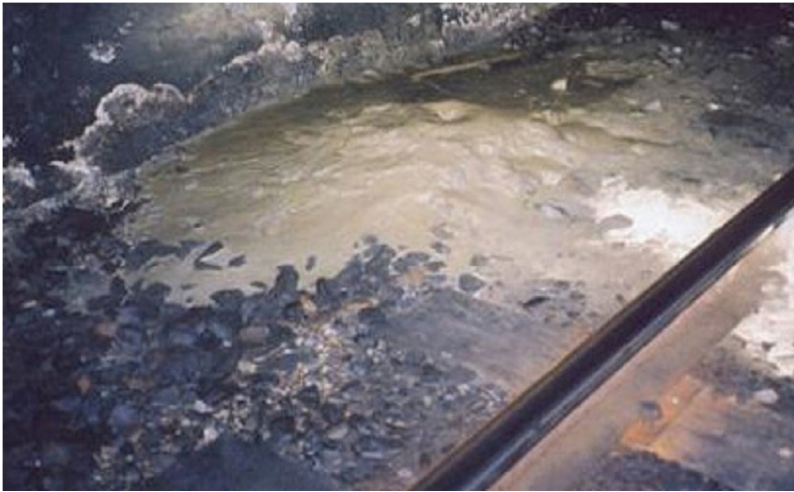
Figure 1.7 Clay pumping along a railway line in the state of Victoria, Australia.
