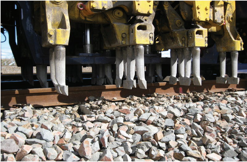
Figure C4 Automated tamping equipment at Singleton.
