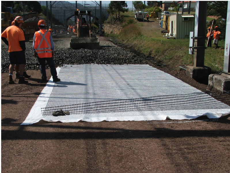
Figure C1 Laying the Geogrid over non-woven geotextile to form a geocomposite layer in fully instrumented rail track at Bulli town north of Wollongong City, New South Wales.
