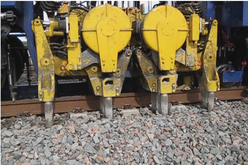
Figure 14.3 Tamping tines penetrating the ballast layer.
