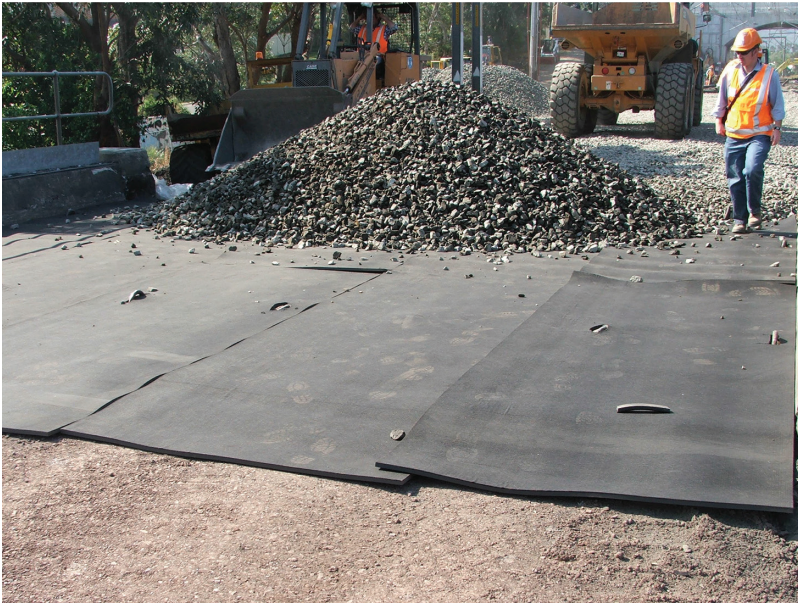
Figure C2 Placing of ballast mat over a bridge deck at Bulli.
