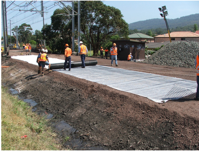
Figure 10.3 Placement of geocomposite over the capping layer.
