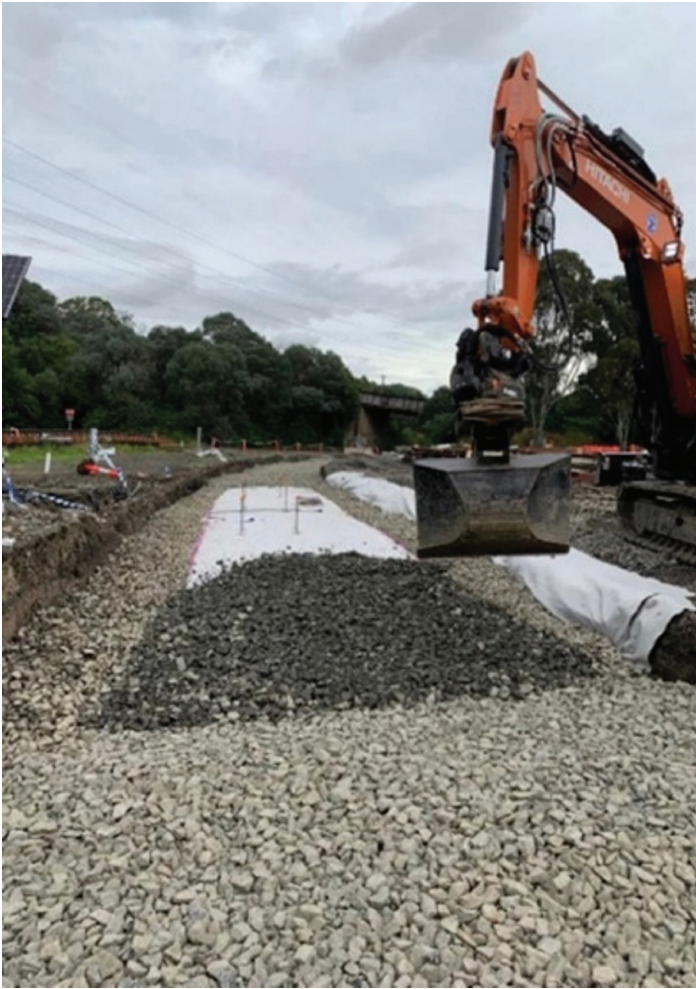
Figure E4 Placing the rubber intermixed ballast system.
