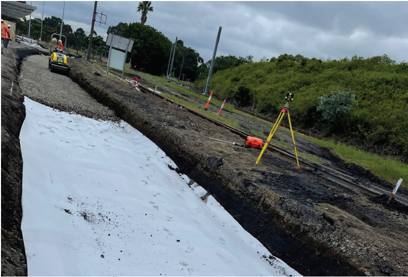
Figure E2 Laying of geotextiles to prevent track instability.
