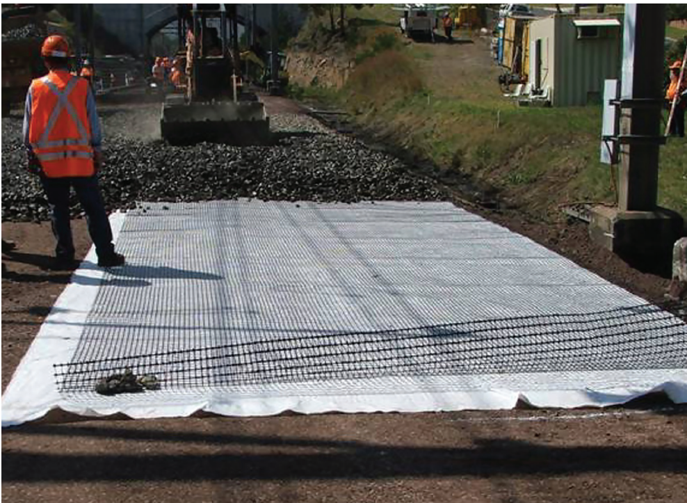
Figure 8.4 Installation of geotextile and geogrid under the ballast layer (NSW, Australia).
