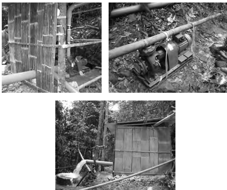
Figure 2.8 Photos of the powerhouse, turbine and outflow from HKT.
