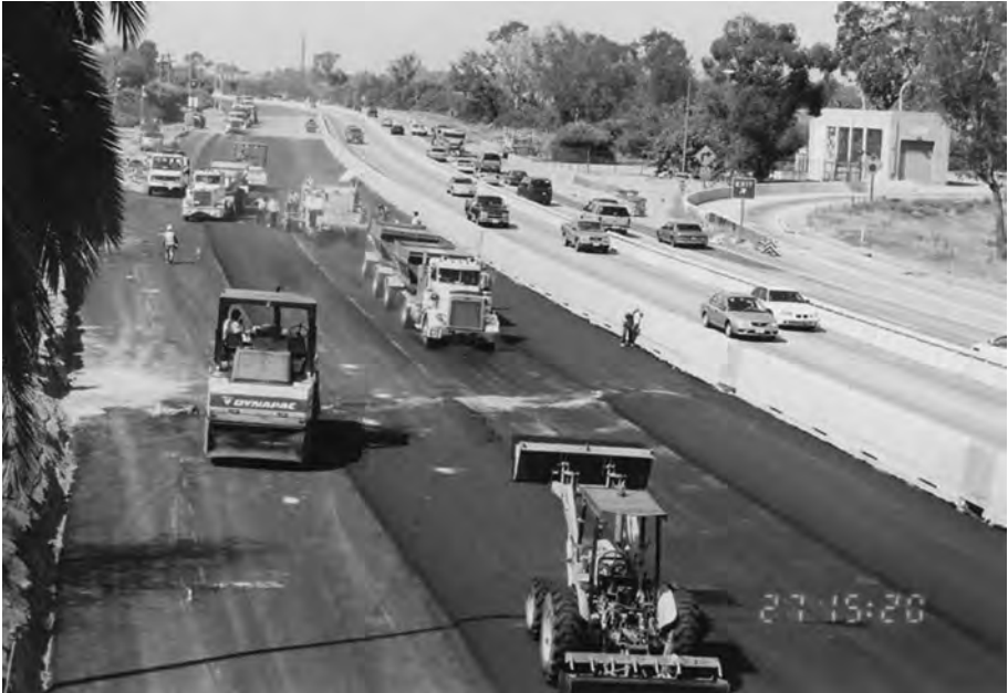
Figure 4.2 Long-life AC pavement rehabilitation on I-710 with 55-hour extended weekend closure.
