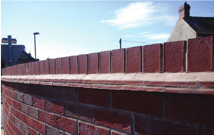
Fig. 226 Double-course tile creasing.
