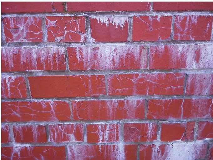
Fig. 265 Lime staining.
