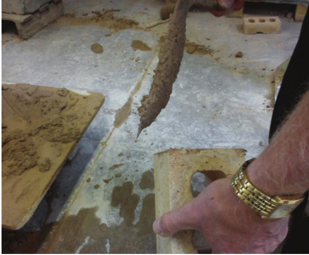
Fig. 117 Preparing to apply a cross-joint.
