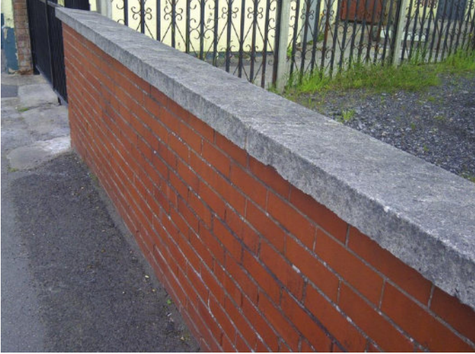
Fig. 238 Pre-cast concrete feather-edge coping.
