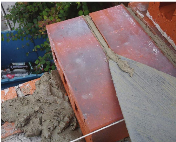
Fig. 213 Excess mortar is trimmed from the cross-joints using the point of the trowel.
