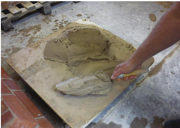
Fig. 110 Picking up the mortar.
