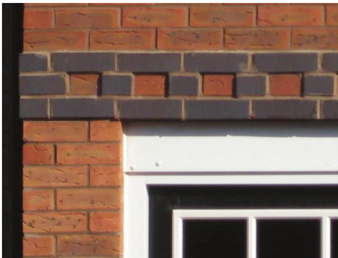
Fig. 253 Dentil course within an oversailing band.
