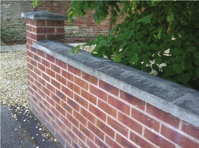
Fig. 239 Pre-cast concrete saddleback coping.
