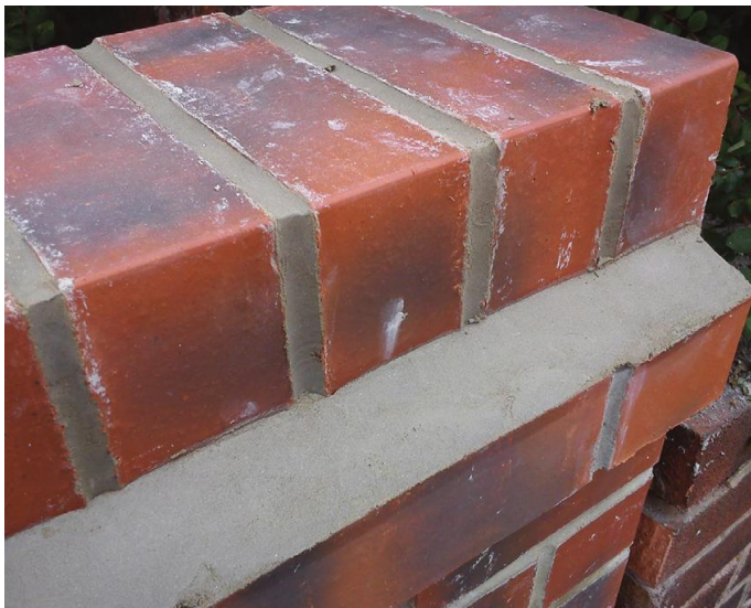
Fig. 233 Finished mortar fillet.
