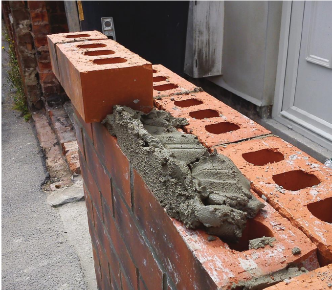
Fig. 220 Exaggerated spreading at outer edge of bed joint for laying oversailing bricks.
