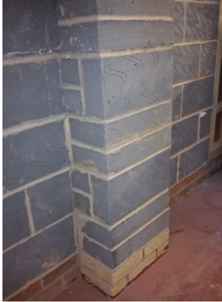
Fig. 104 Attached pier in blockwork.
