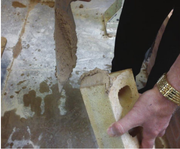
Fig. 118 Applying the first part of the crossjoint.
