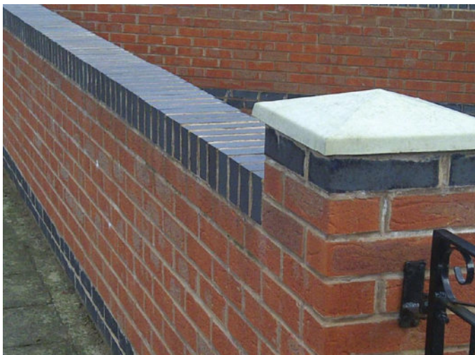
Fig. 240 Pre-cast concrete saddleback pier cap.
