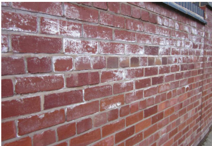
Fig. 264 Efflorescence.
