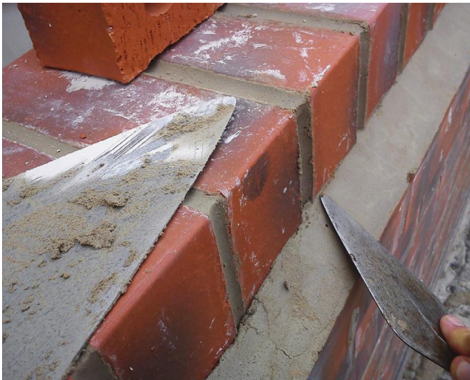
Fig. 232 Mortar fillet polished and compacted with a wet pointing trowel.
