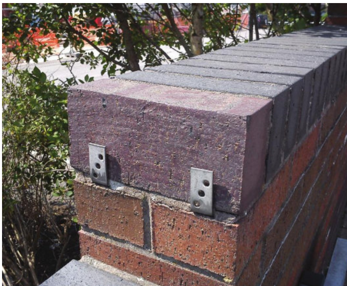
Fig. 209 Simple brick-on-edge coping: the end brick is held in place with galvanized frame cramps.
