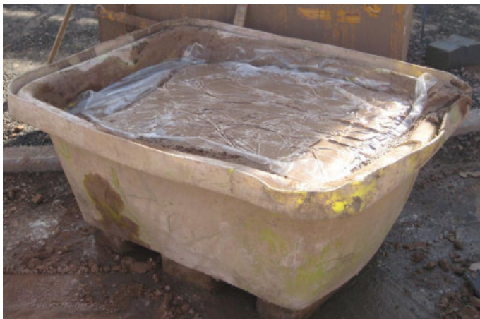
Fig. 24 Ready-mix mortar delivered to site.
