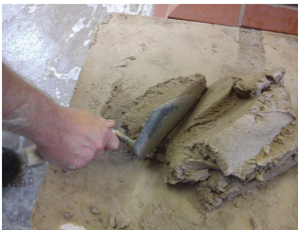
Fig. 107 Cutting mortar.
