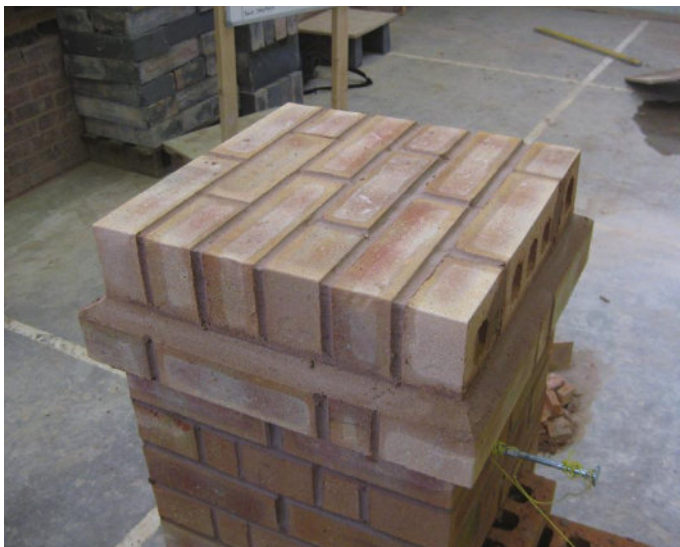
Fig. 237 Bonded brick-on-edge pier cap.
