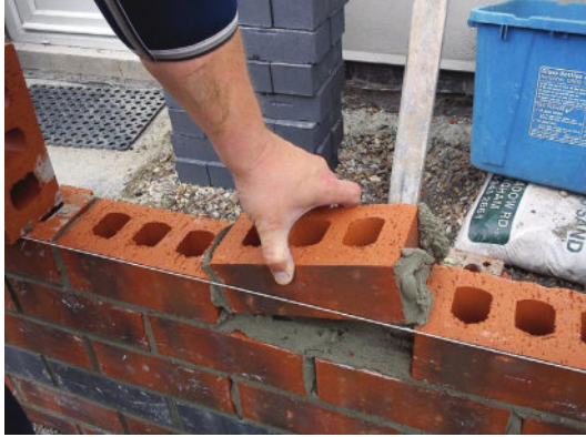
Fig. 141 Laying the last brick to a line.
