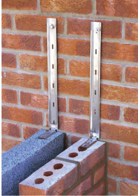
Fig. 276 Staifix universal wall-starter system, a typical example of such a system, shown during construction with a new cavity junction wall being joined to an existing wall. Ancon Building Products
