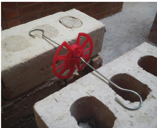
Fig. 176 Plastic insulation-retaining clip.
