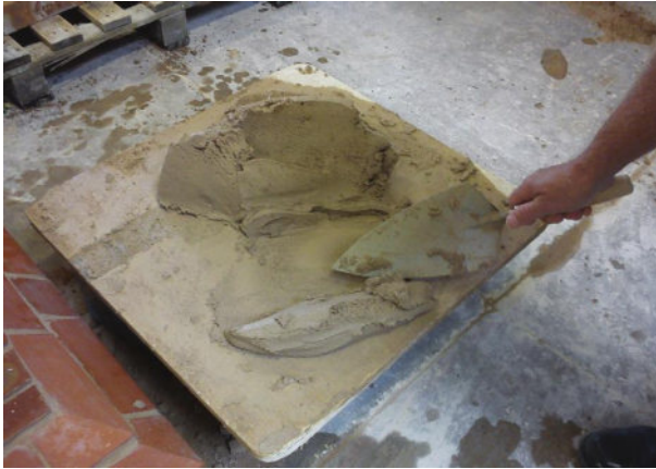
Fig. 109 Preparation for picking up the mortar.
