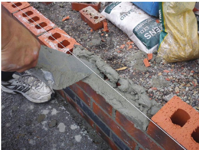
Fig. 140 Furrowing under the line.
