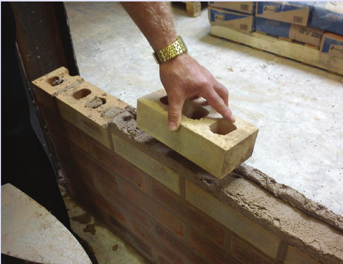
Fig. 114 The correct way to hold a brick.
