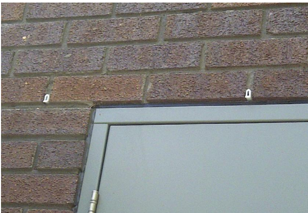
Fig. 191 Plastic weepholes inserted above a door opening.
