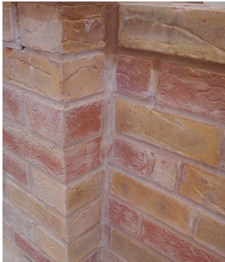
Fig. 165 Half-round jointing correctly finished at an internal corner.
