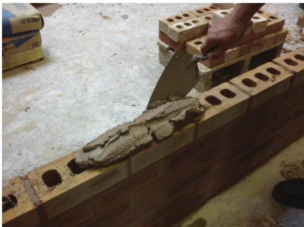
Fig. 111 Spreading mortar.
