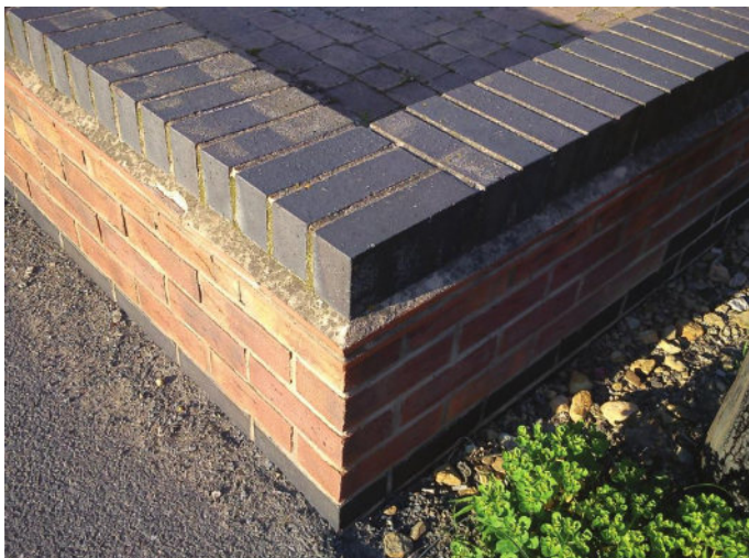
Fig. 215 The simplest method of returning a brick-on-edge coping at a corner.
