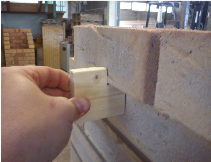
Fig. 219 Gauging a consistent overhang with a notched piece of timber.
