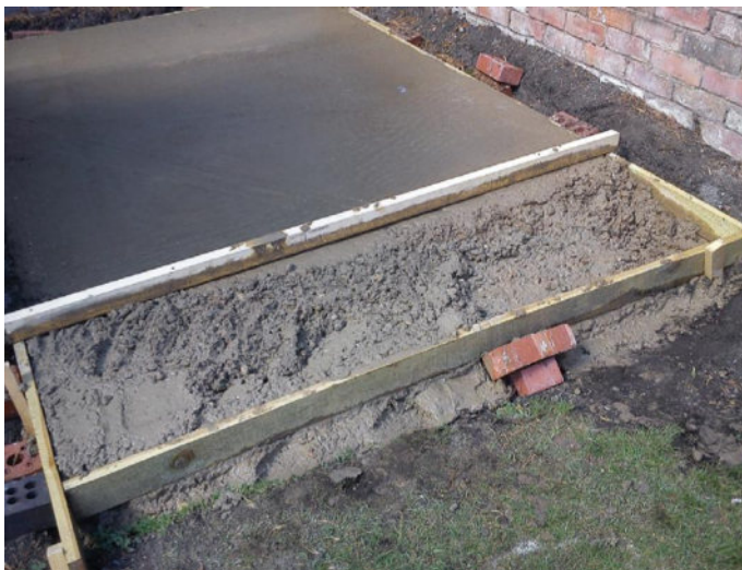
Fig. 15 Use of a tamping board to compact and level concrete within timber framework.
