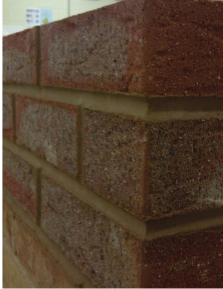
Fig. 164 Half-round jointing correctly finished at an external angle.
