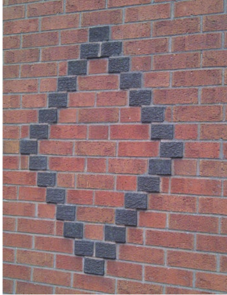
Fig. 251 Projecting single diaper.
