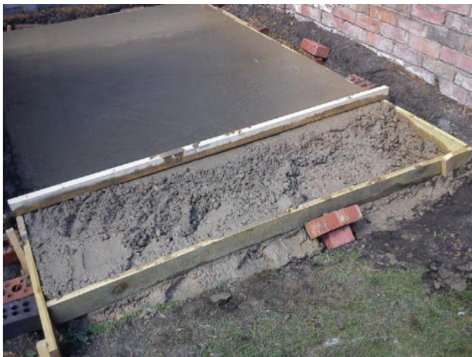
Fig. 47 Simple formwork for a small concrete base.
