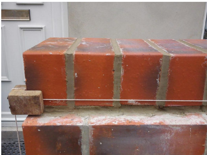
Fig. 230 String-line used as a guide for the top of a mortar fillet.
