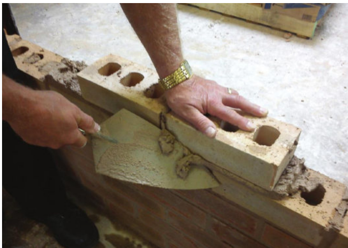
Fig. 121 Laying the next brick.
