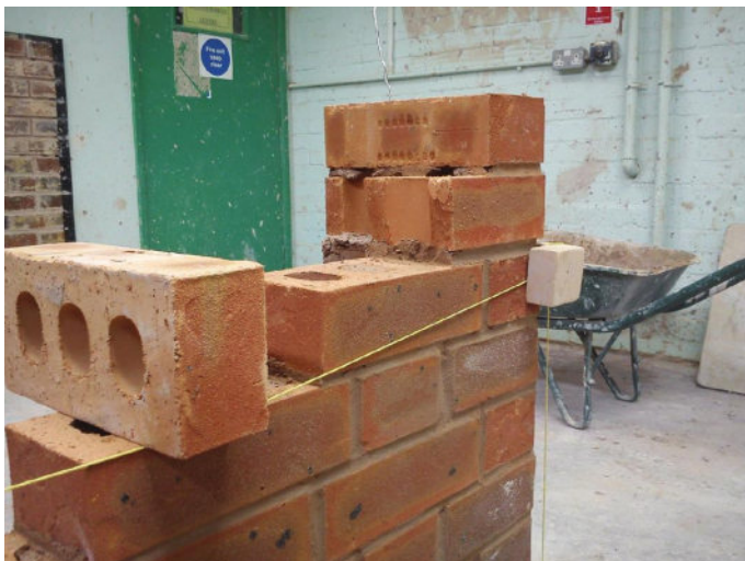
Fig. 137 'Spragging' the line down with a dry brick.
