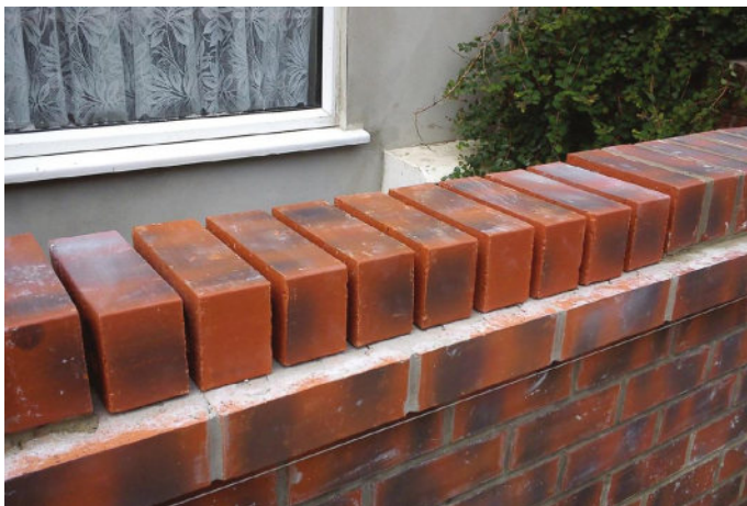
Fig. 211 The middle of the brick-on-edge coping is set-out by dry bonding.
