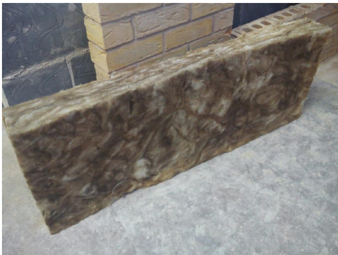
Fig. 173 Full-fill cavity-wall insulation.
