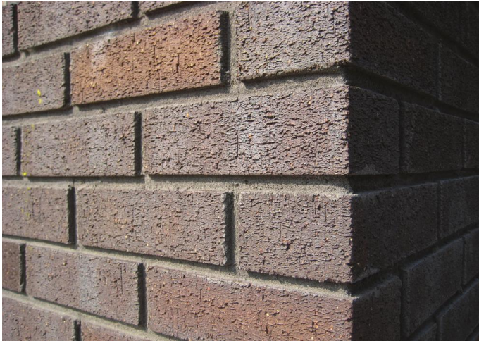
Fig. 157 Recessed joint finish.
