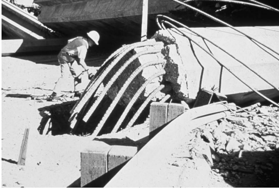
FIGURE 1.13 Lap-splice failure. (With permission from Caltrans.)
