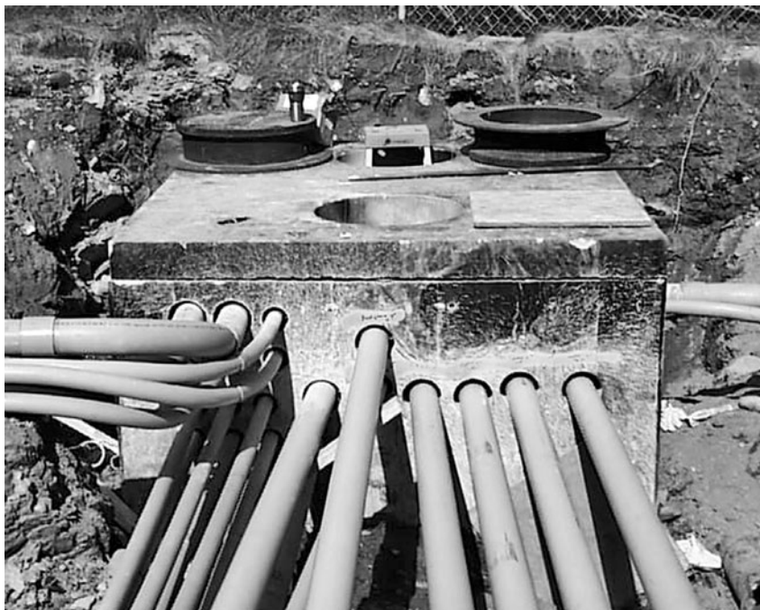
FIGURE 3.2 Conduit and manhole.
