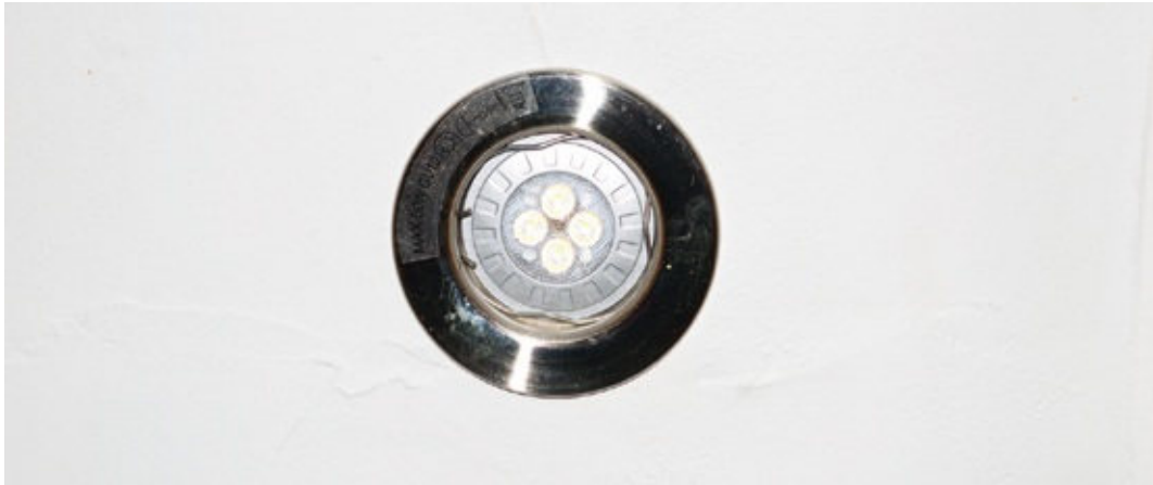
Figure 4.37 Recessed lights are sometimes referred to as downlighters
