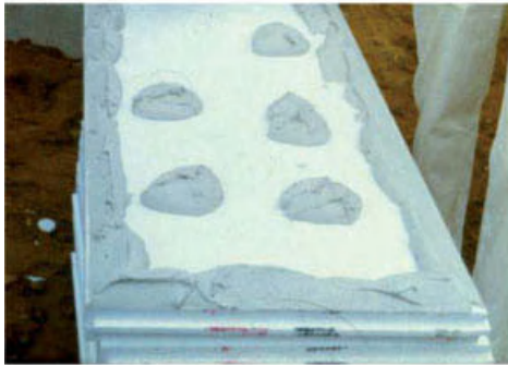
Pointwise mopping the bonding mortar
