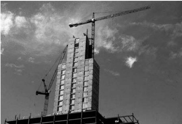
Figure 6.9. High rise with central core under construction.
