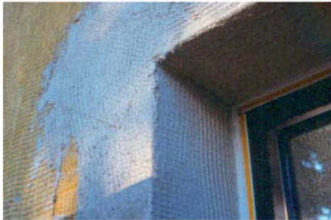
Fixing the stucco guides
