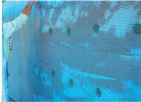
Additional fixing with synthetic nails
