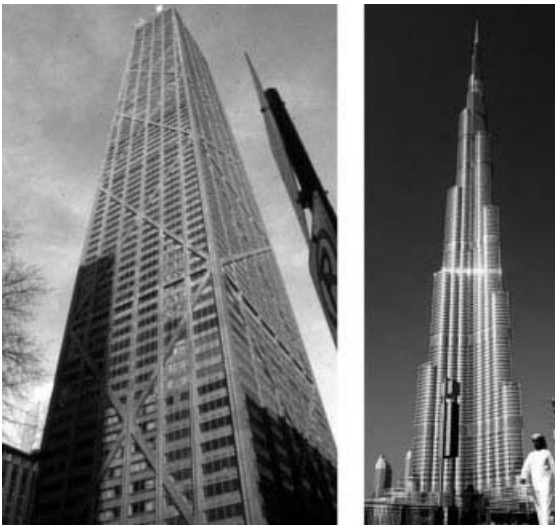
Figure 6.5. Shapes of equal resistance: the John Hancock tower in Chicago and the Burj Khalifa in Dubai.
