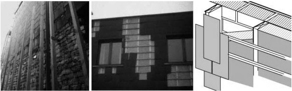
Figure 9.29. Massive walls with outside insulation: stud systems.
