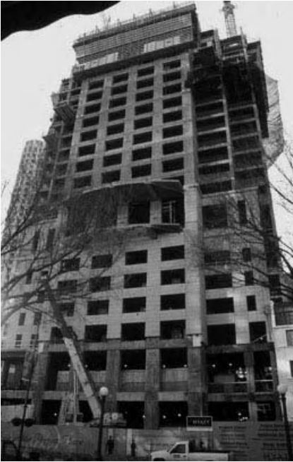
Figure 6.10. Tube as Vierendeel girder.
