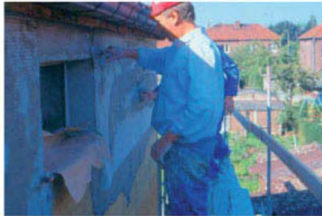
Embedding the glass fibre fabric
