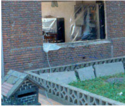
Outer wall to be insulated
