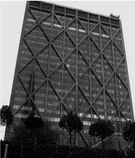
Figure 6.11. Trussed tube.
