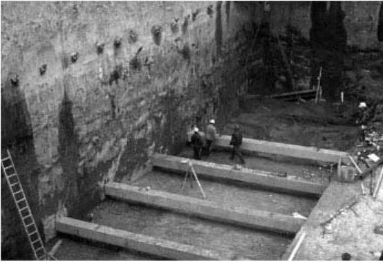
Figure 3.2. Deep walls nailed with grout anchors.
