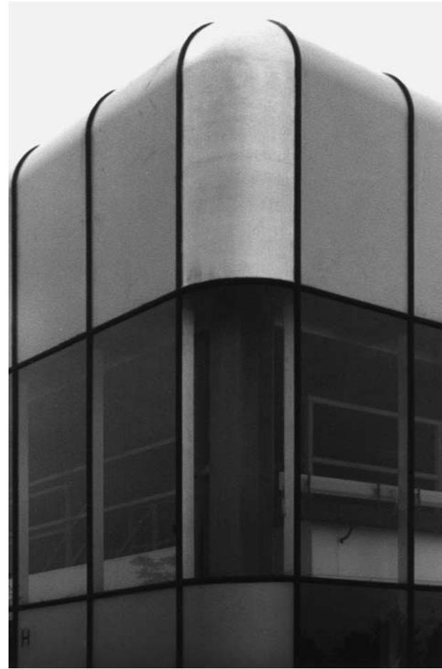
3.13 Corner panels at Winwick Quay (architects: Nicholas Grimshaw Partnership).
