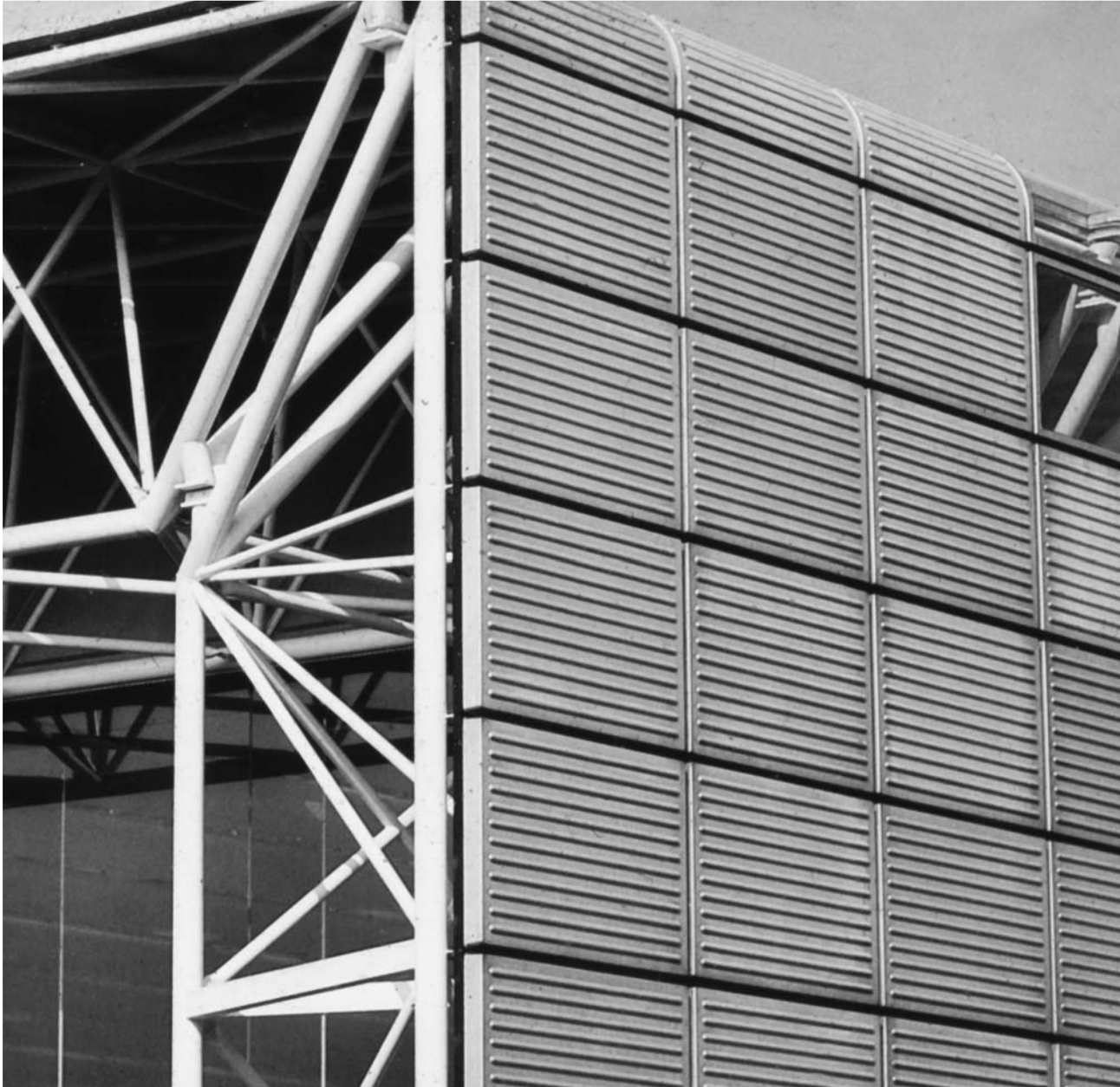
6.7 Sainsbury Centre panels (architects: Foster Associates).
