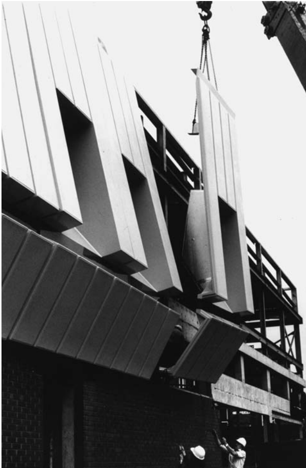
3.12 Nottingham Co-op under construction.
