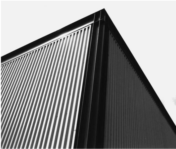
5.30 Corner detail with exposed steel frame.
