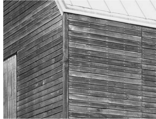
8.22 Cladding of green oak on the Rowing Museum, David Chipperfield, Henley-on-Thames.
