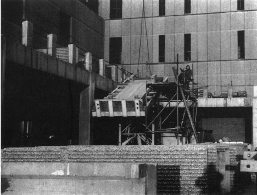
1.15 Tilting platform as used at Liverpool Royal Insurance building.
