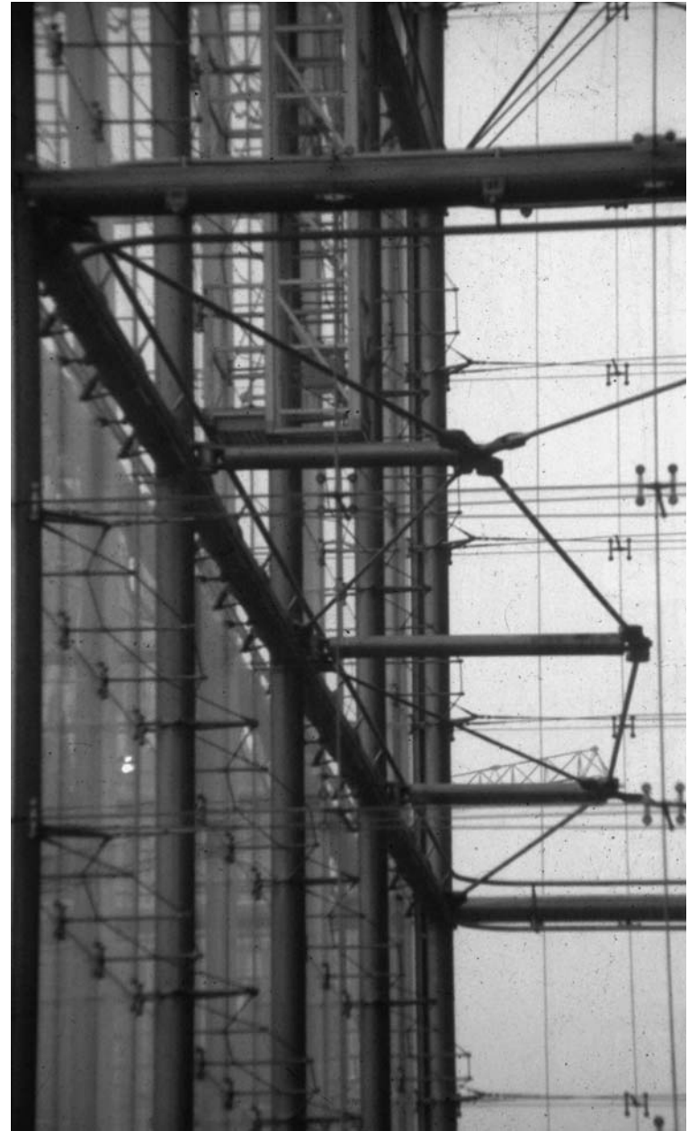
7.30 Parc de la Villette structure support of glazing.
