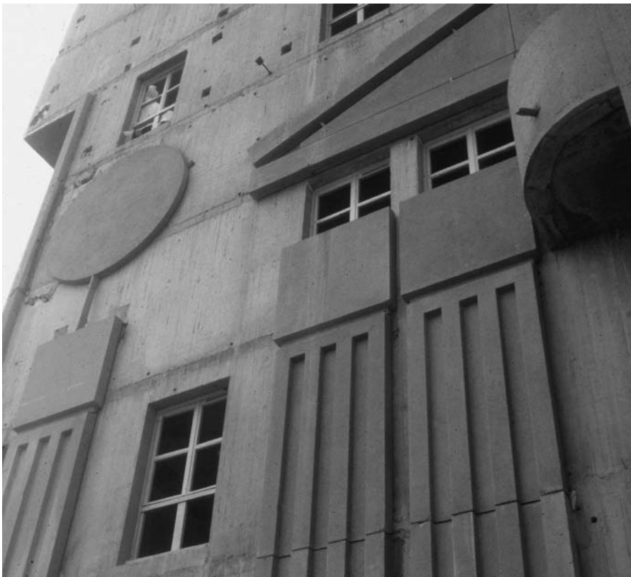
1.1 Construction of precast and in situ concrete at the Les Espaces d'Abraxas, a monumental housing scheme near Paris (architect: Ricardo Bofill).
