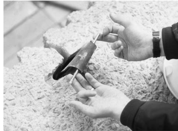
1.25 Baffle fixed over stainless steel pin for easy renewal.
