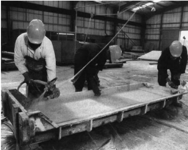
4.2 Typical hand lay-up operation.
