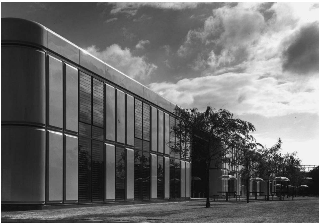
3.11 Panels at Herman Miller factory, Bath (architects: Farrell and Grimshaw).
