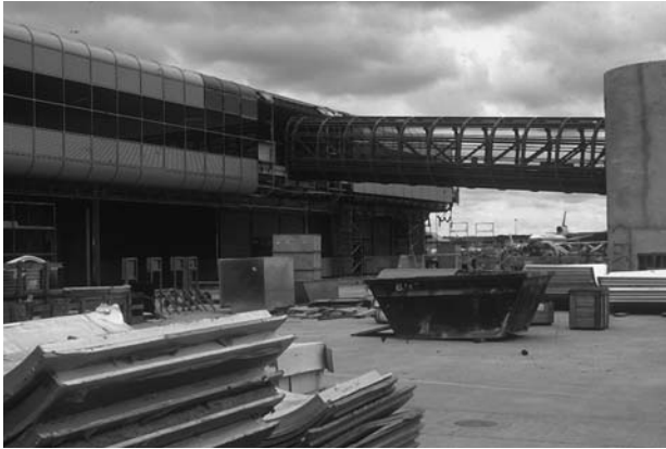
6.10 Assembly of panels at Gatwick Airport North Piers.
