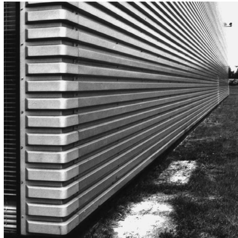
5.14 IBM offices, Greenford (architects: Foster Associates).
