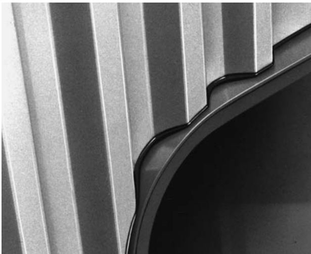
5.31 Neoprene flashing at window opening.
