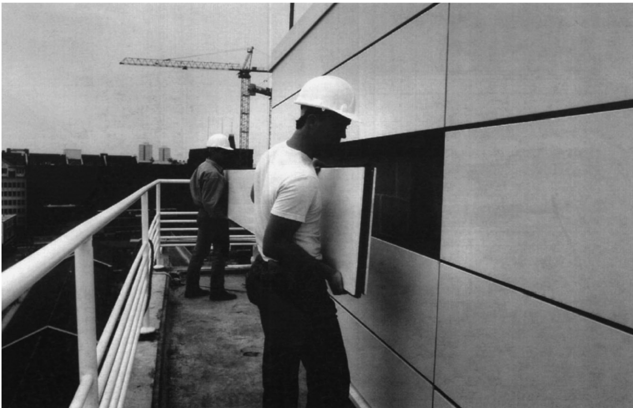
6.37 Interchangeable facade panels.
