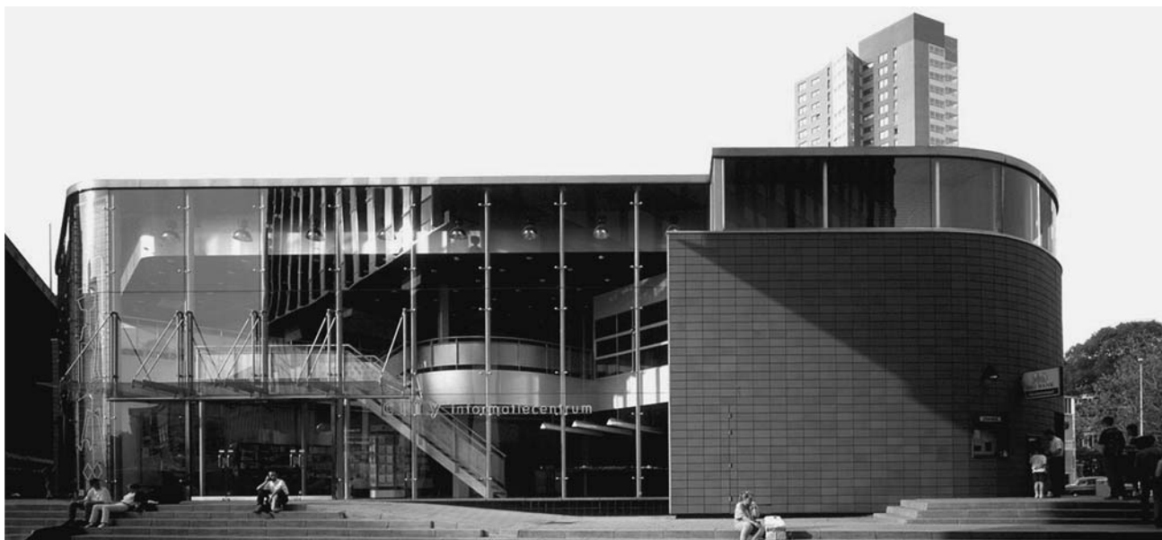
2.5 Churchill Centre Rotterdam (architects: Brookes Stacey Randall). Photo: Christian Richters and Nik Randall.
