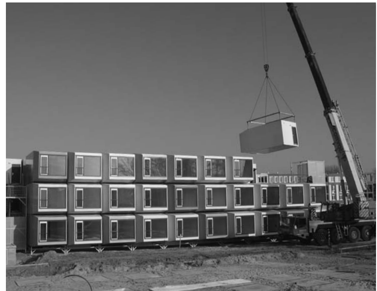
3.30 Placement of Spaceboxes as student accommodation in Amersfoort by Holland Composites Industrials.
