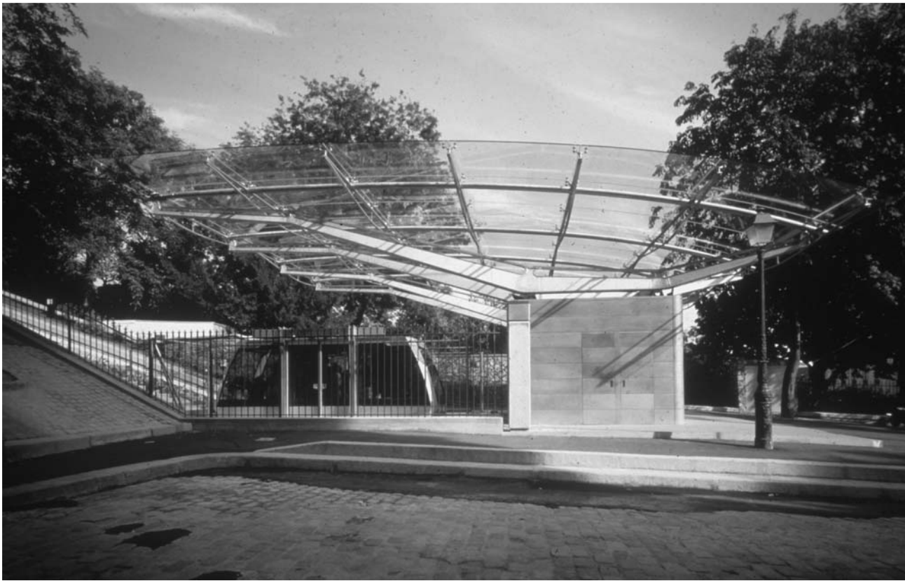
7.32 Curved laminated glass used at Montmartre funicular.
