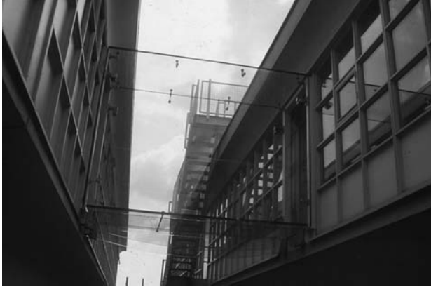
7.38 Laminated toughened glass as used at the glass bridge in Rotterdam by engineer Robert Nijse.
