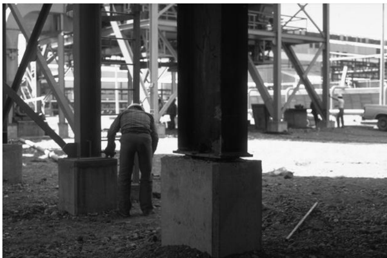
Figure 2.31 Earthquake-induced foundation settlement (Michoacán Guerrero earthquake, 1985).
