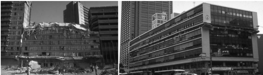
Figure 2.15 Collapse of top floors in Mexico City (1985) or of an intermediate one in Kobe (1995).
