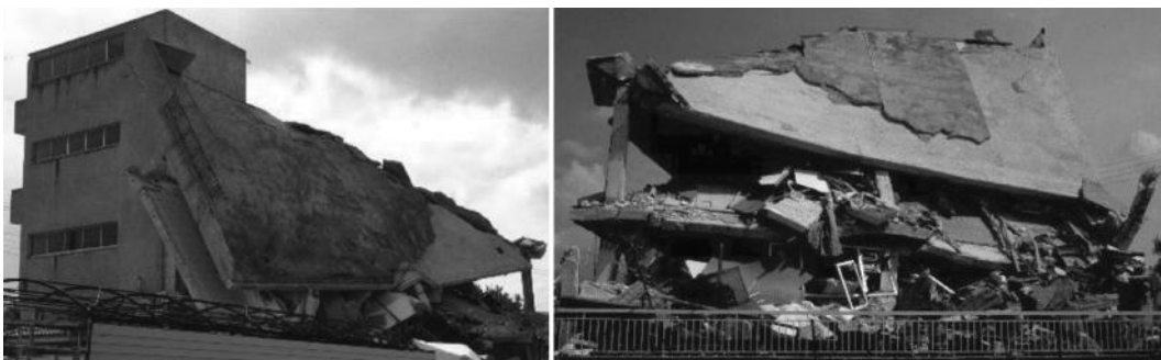
Figure 2.16 Collapse of flexible sides in torsionally imbalanced building with stiffness concentrated near one corner.
