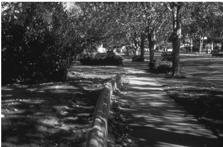
Figure 2.4 Fence offset in Hollister, California.
