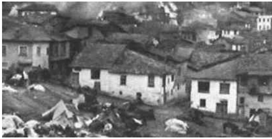
Figure 6.6 The Gediz earthquake (Turkey, 1970).
