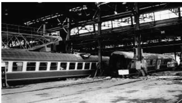
Figure 1.43 Damaged steel building of the railcar factory. (After Erdik, M. 2000: Report on 1999 Kocaeli (Turkey) Earthquake. Bogazici University Report 2000.)
