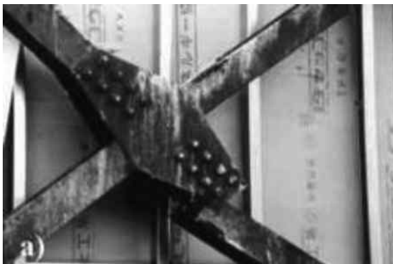
Figure 1.30 Collapse of bolted connections in bracings. (Gioncu, V., Mazzolani, F.M. 2002: Ductility of Seismic Resistant Steel Structures . Spon Press, London; after Fischinger, M. 1997: EASY, Earthquake Engineering Slide Information System. FGG-IKPIP Institute Slovenia.)
