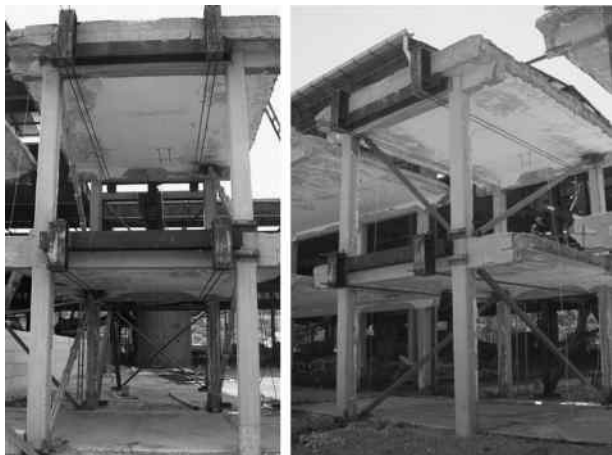
Figure 4.35 The RC structure equipped with BRBs.
