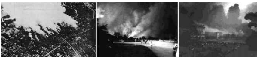
Figure 6.5 The Great Kanto earthquake (Japan, 1923).
