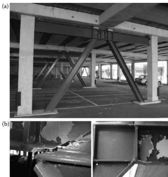
Figure 1.51 Parking garage: (a) eccentrically braced system; (b) damage of the link beam in the welding zone and yielding in the web. (Clifton Ch. et al. 2011: Bulletin of the New Zealand Society for Earthquake Engineering , 44(4):297–318.)
